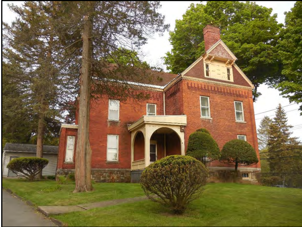
Figure 5. Superintendent's Residence, North Side.
