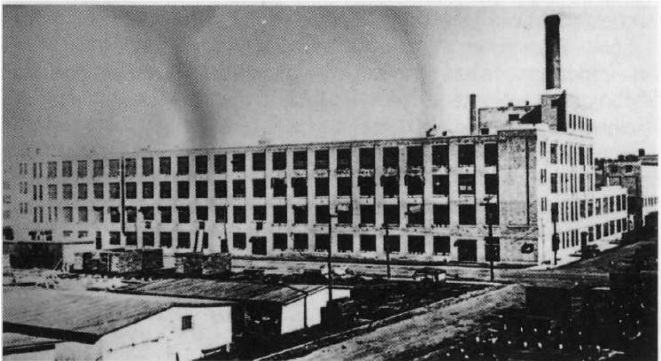
Figure 5: West and south elevations of building, c. 1950s
