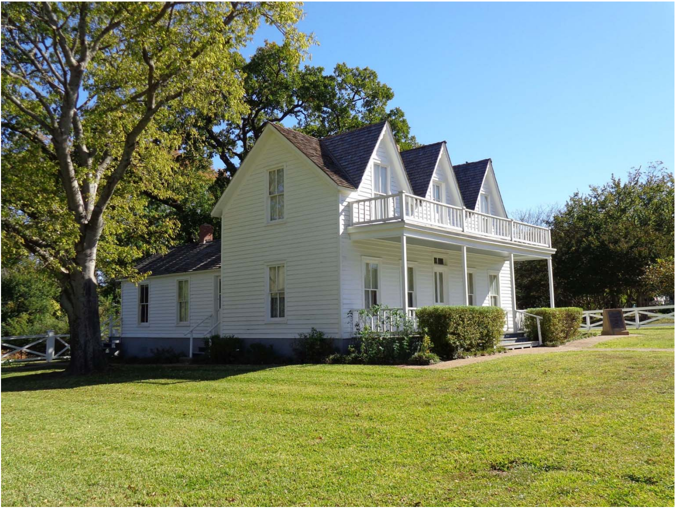
TX_Grayson County_Eisenhower Birthplace_0003 North and west (front) elevations, oblique; view southeast
