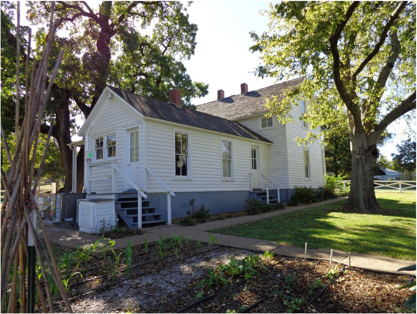
TX_Grayson County_Eisenhower Birthplace_0005 East (rear) elevation of rear ell, and north elevation; view southwest
