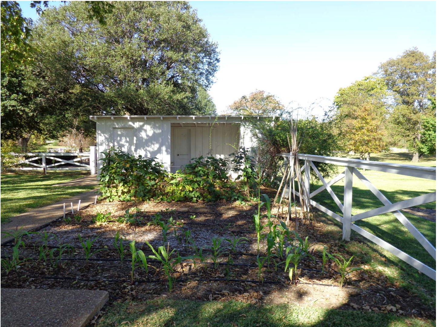
TX_Grayson County_Eisenhower Birthplace_0015 South elevation of outbuilding; view north
