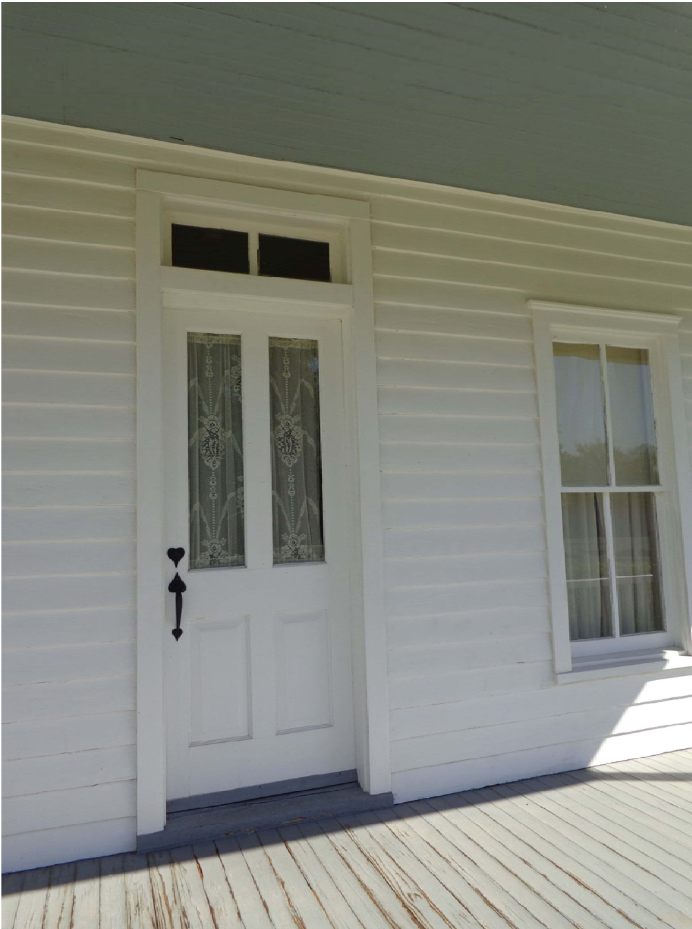
TX_Grayson County_Eisenhower Birthplace_0009 Entry door of west façade; view east
