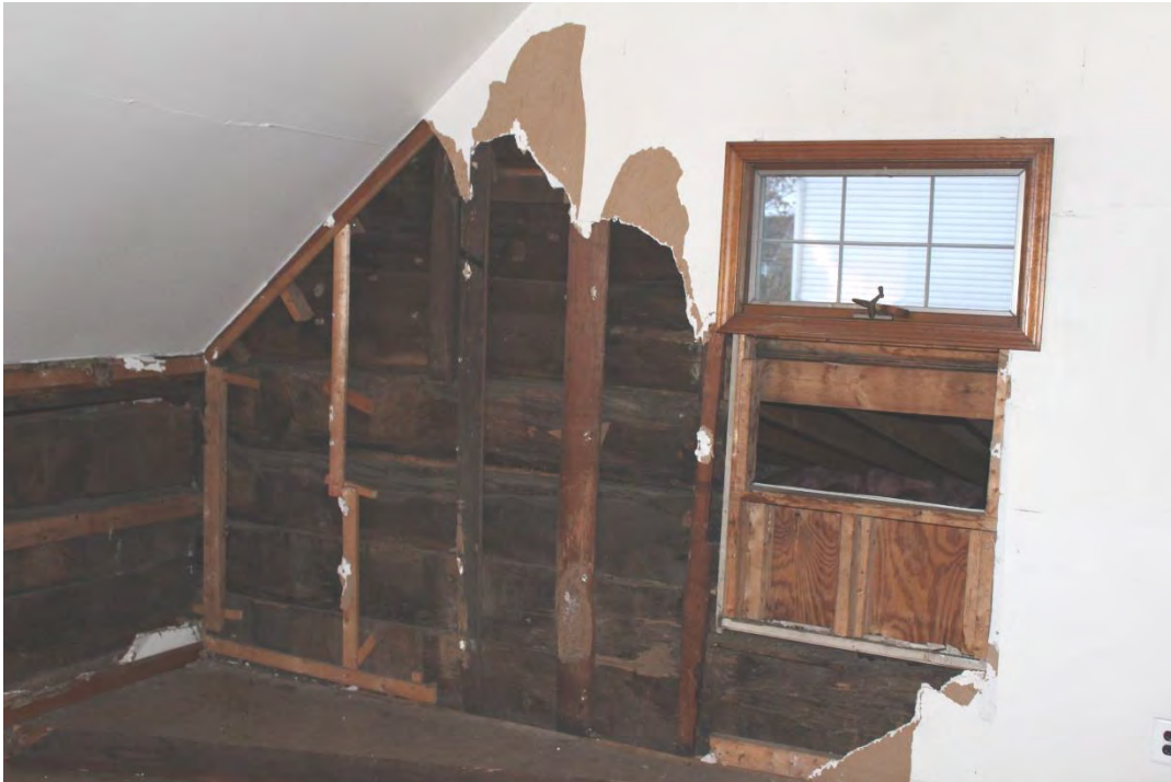
Photo 11: Interior, Original Section, garret, south and east walls.
