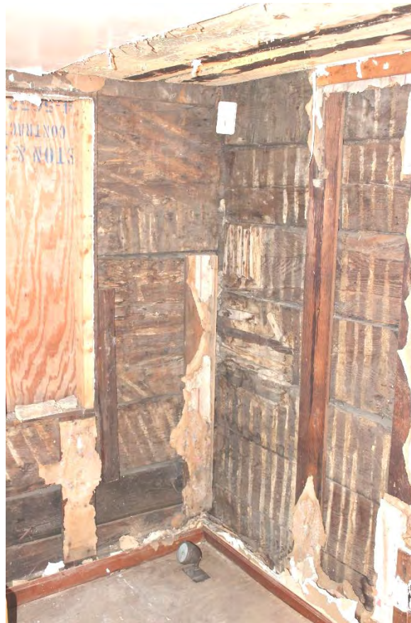
Photo 4: Interior, Original Section, 1 st floor, SW corner.
