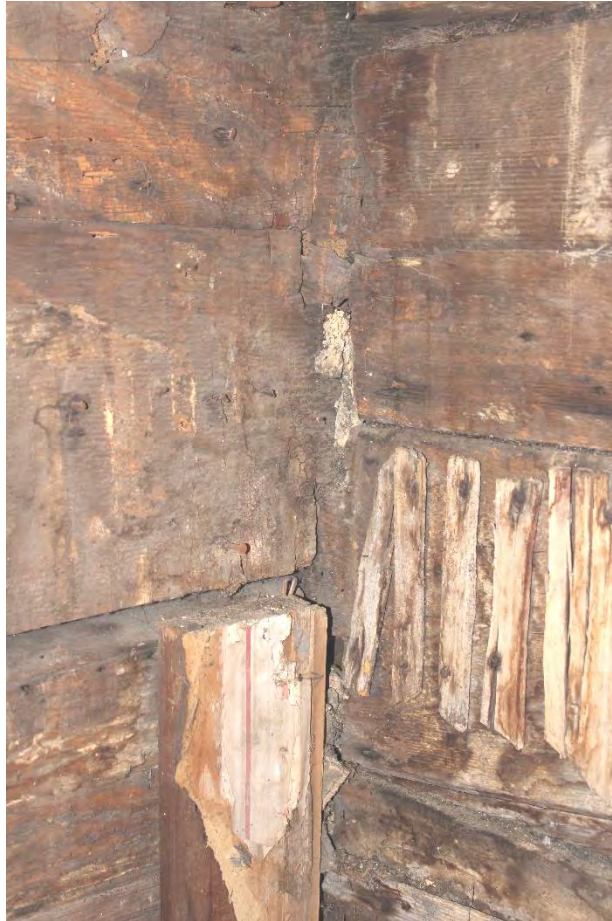
Photo 5: Interior, Original Section, 1 st floor, SW corner, detail of corner-notch joints.
