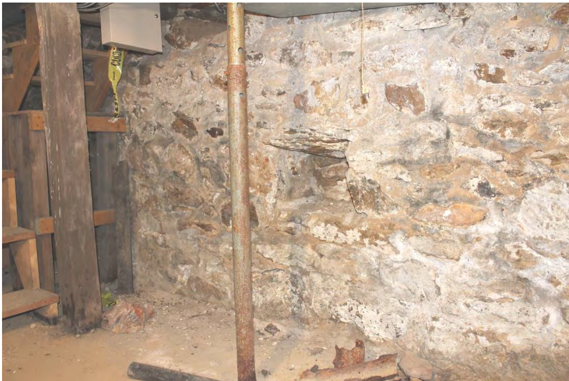
Photo 8: Interior, Original Section, cellar, east wall and shelf niche.
