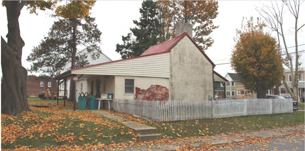
Photo 3: Plank House, east and north elevations.
