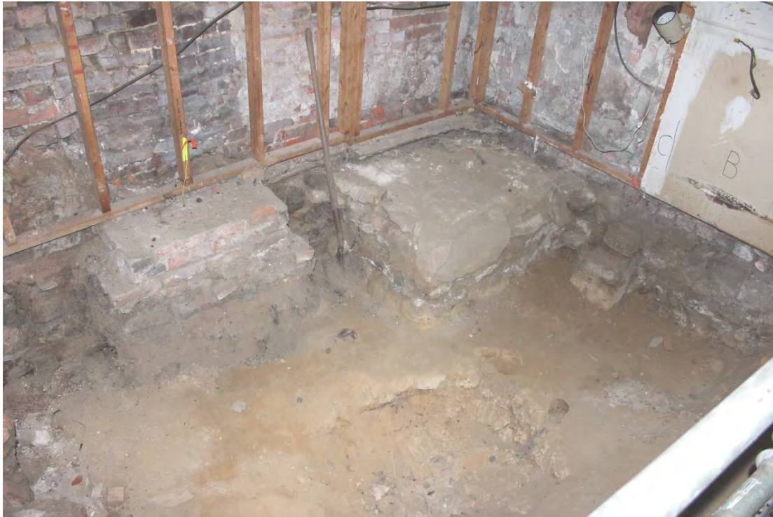
Photo 13: Interior, East Addition, remnants of original hearth structure.
