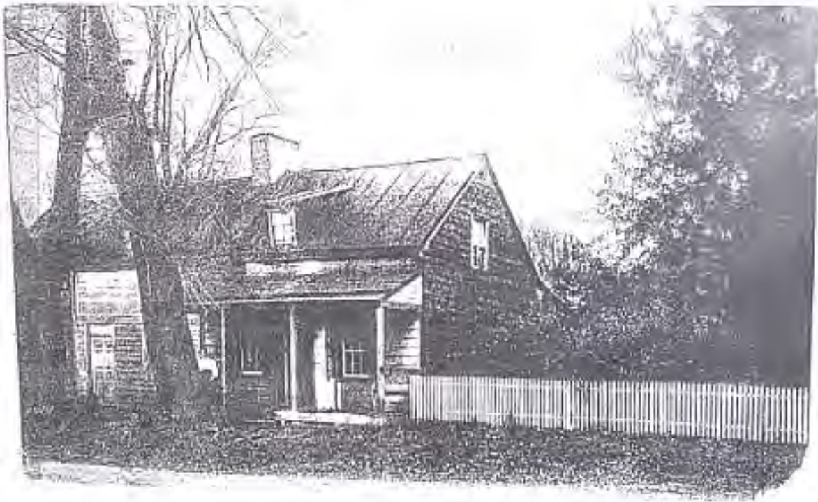
Figure 8: Historic photo, probably early 1900s, note presence of two added sections to left.
