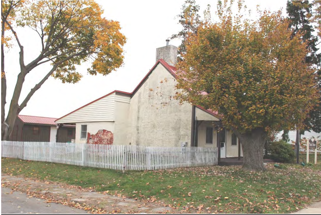
Photo 1: Plank House, north and west elevations.
