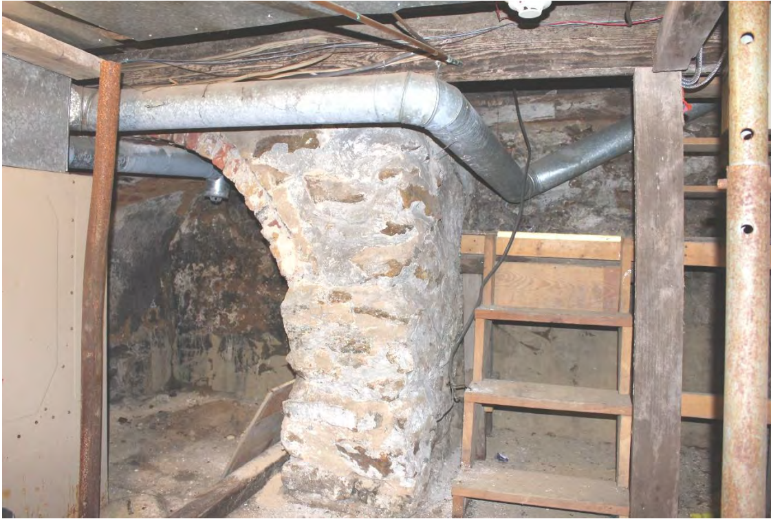
Photo 7: Interior, Original Section, cellar, north wall and relieving arch.
