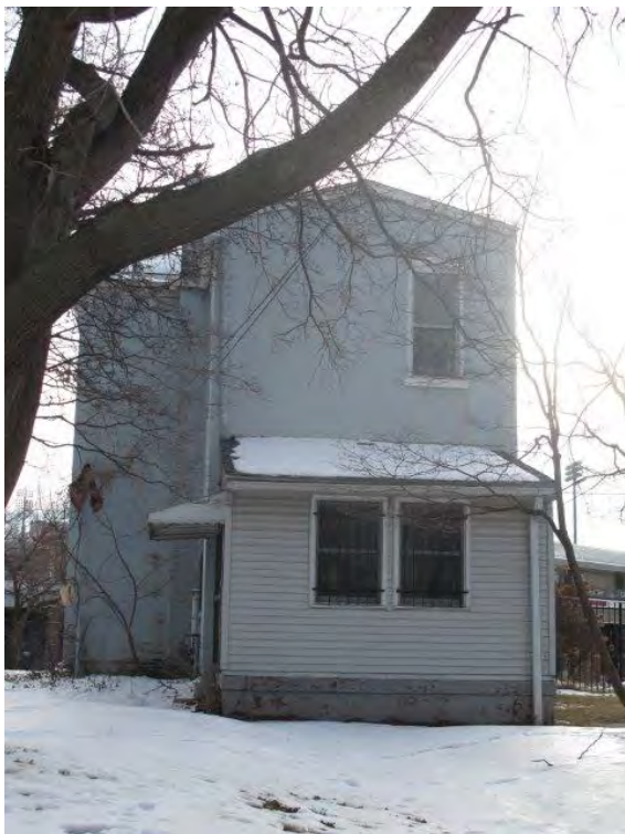
Photo 4: West (rear) elevation
