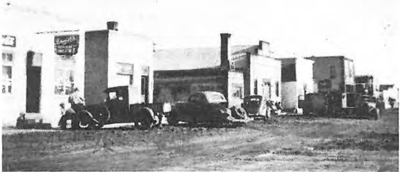
Fig. 20: Historic photo streetview of Forest River’s main street – north block, looking south 1941 [Forest River State Bank located far right] ( Forest River North Dakota 1887-1987, 1987 )
