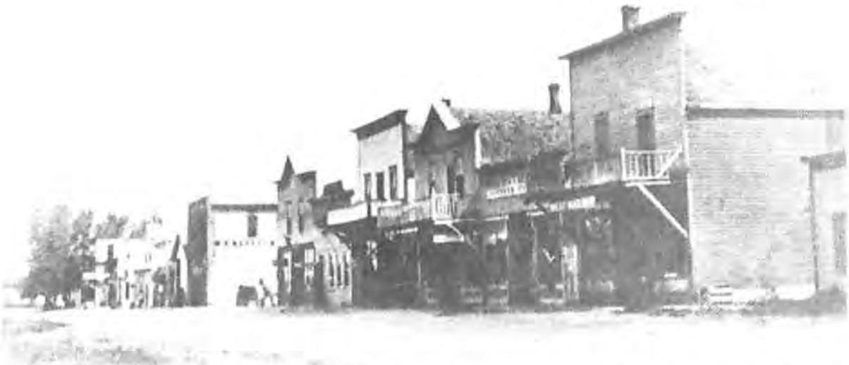
Fig. 5: Historic photo streetview of Forest River's main street – south block looking north prior to 1918 fire, 1916 ( Forest River North Dakota 1887-1987, 1987 )
