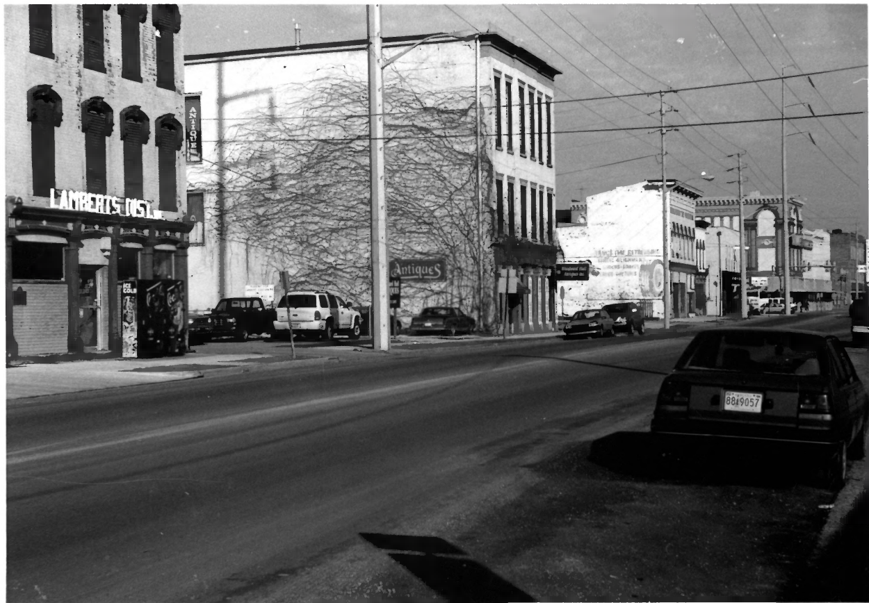
142 W. MAIN, NEW ALBANY DOWNTOWN HIST. DIST, FLOYD CO. IN , PHOTO NO. 33
