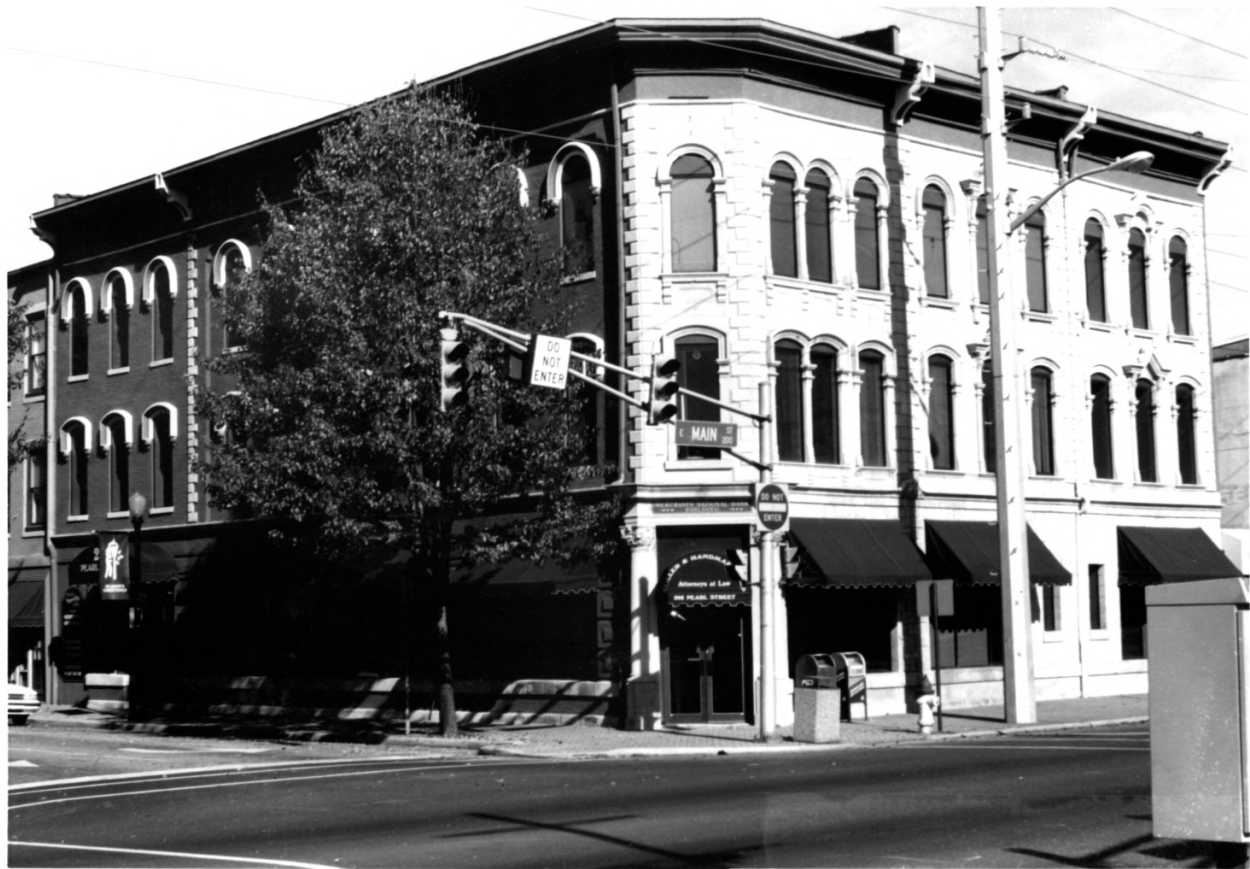
202-204 PEARL ST., NEW ALBANY DOWNTOWN HIST. DIST. ROYD CO., IN, PHOTO No. 28
