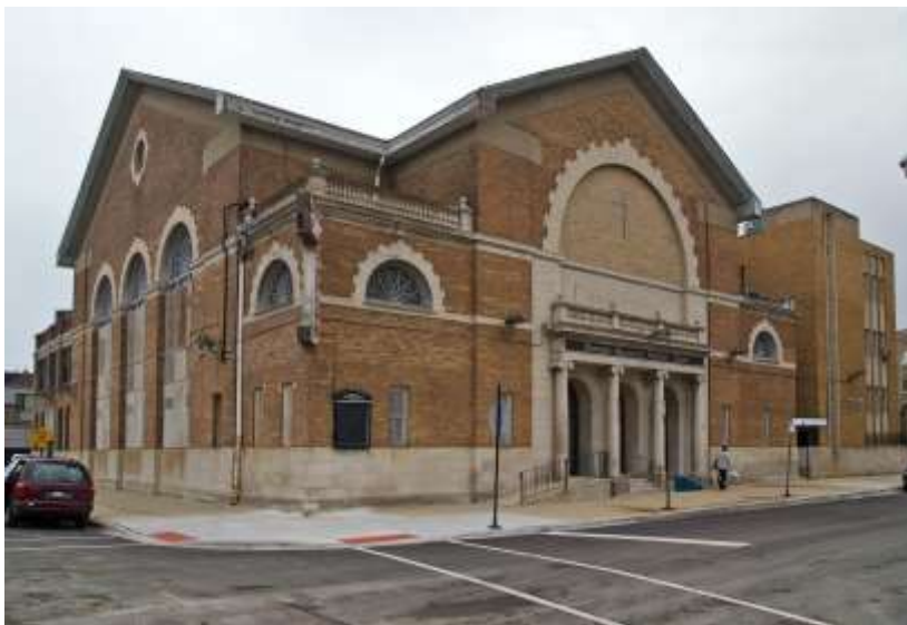
Above left: Site Plan showing Ebenezer Baptist Missionary Baptist Church and Dr. Frank K. Sims Education Center; From Commission on Chicago Landmarks -- Landmarks Designation Report: Ebenezer Missionary Baptist Church -- prepared by the Historic Preservation Division Staff, Department of Housing and Economic Development, June, 2011. Above right: View showing the church and center, facing northeast. Google Earth. Below: View showing the church and center, facing southeast. Photographer, Kevin Eatinger.
