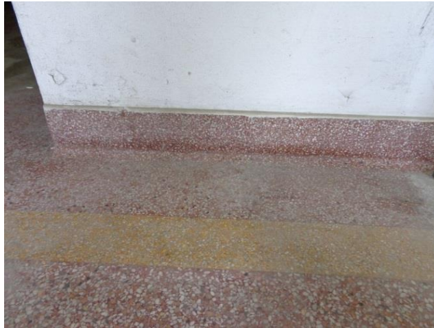
Figure 11 & 12: Terrazzo floors at the portico and on the first floor. Photos by Guillermo Ortiz Palacios June 2014.
