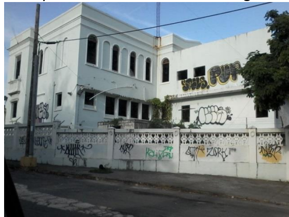
Figure 2: Building addition in the side view. Photo by Maria F. López July, 2015
