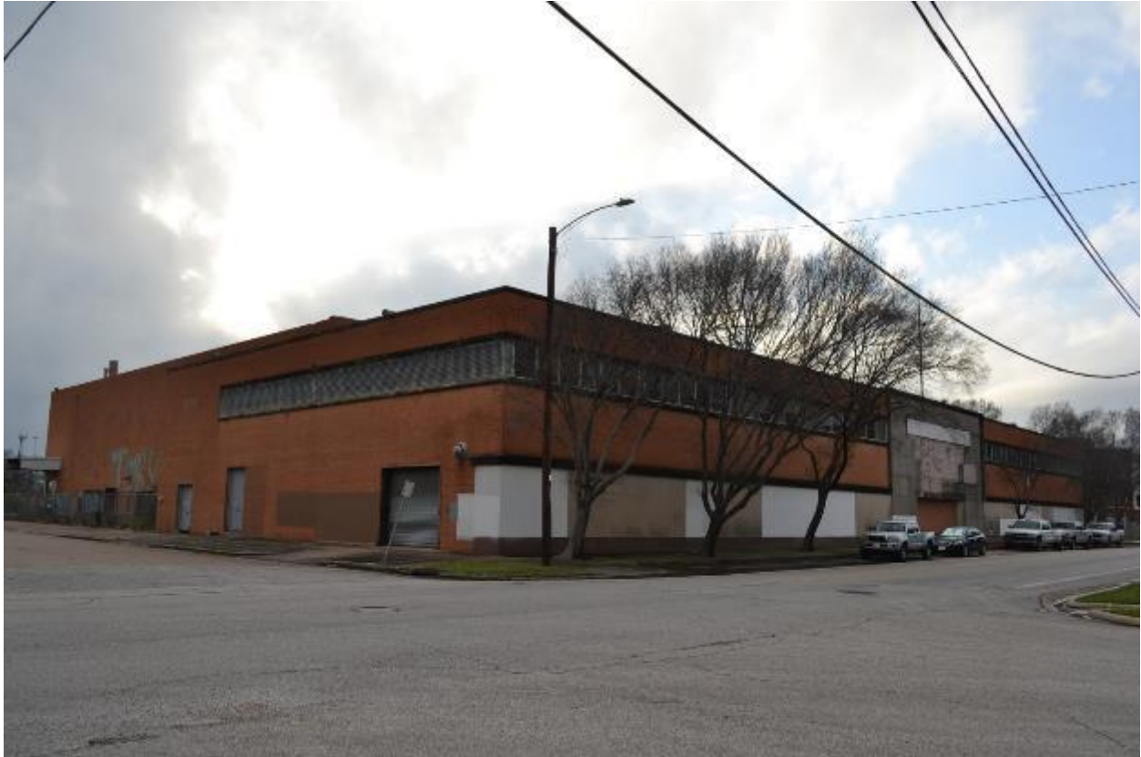
Photo 1 – East elevation (L) and north façade (R), view southwest.
