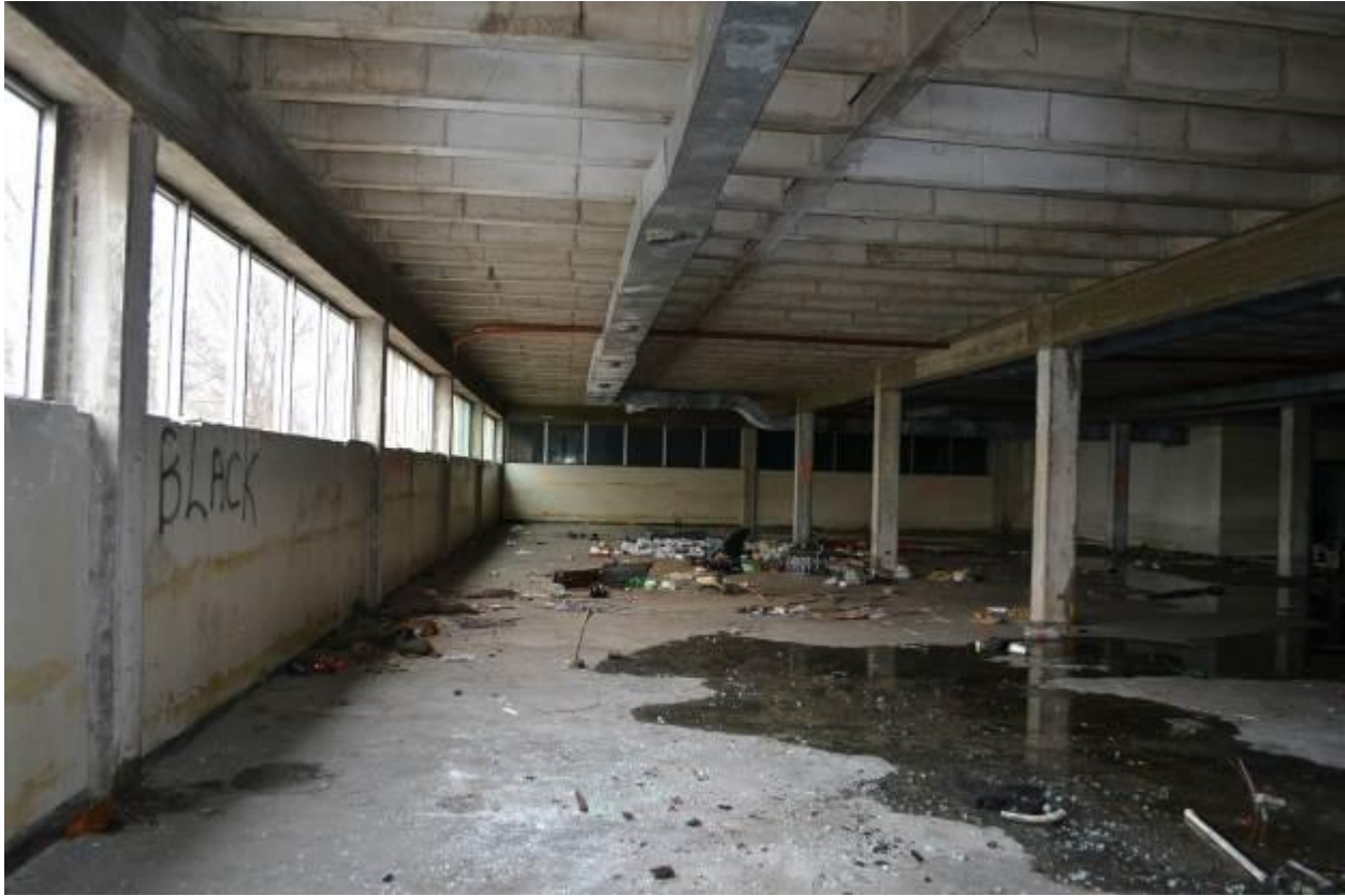
Photo 14 – Interior, second floor newsroom, view east. Original ribbon windows intact.
