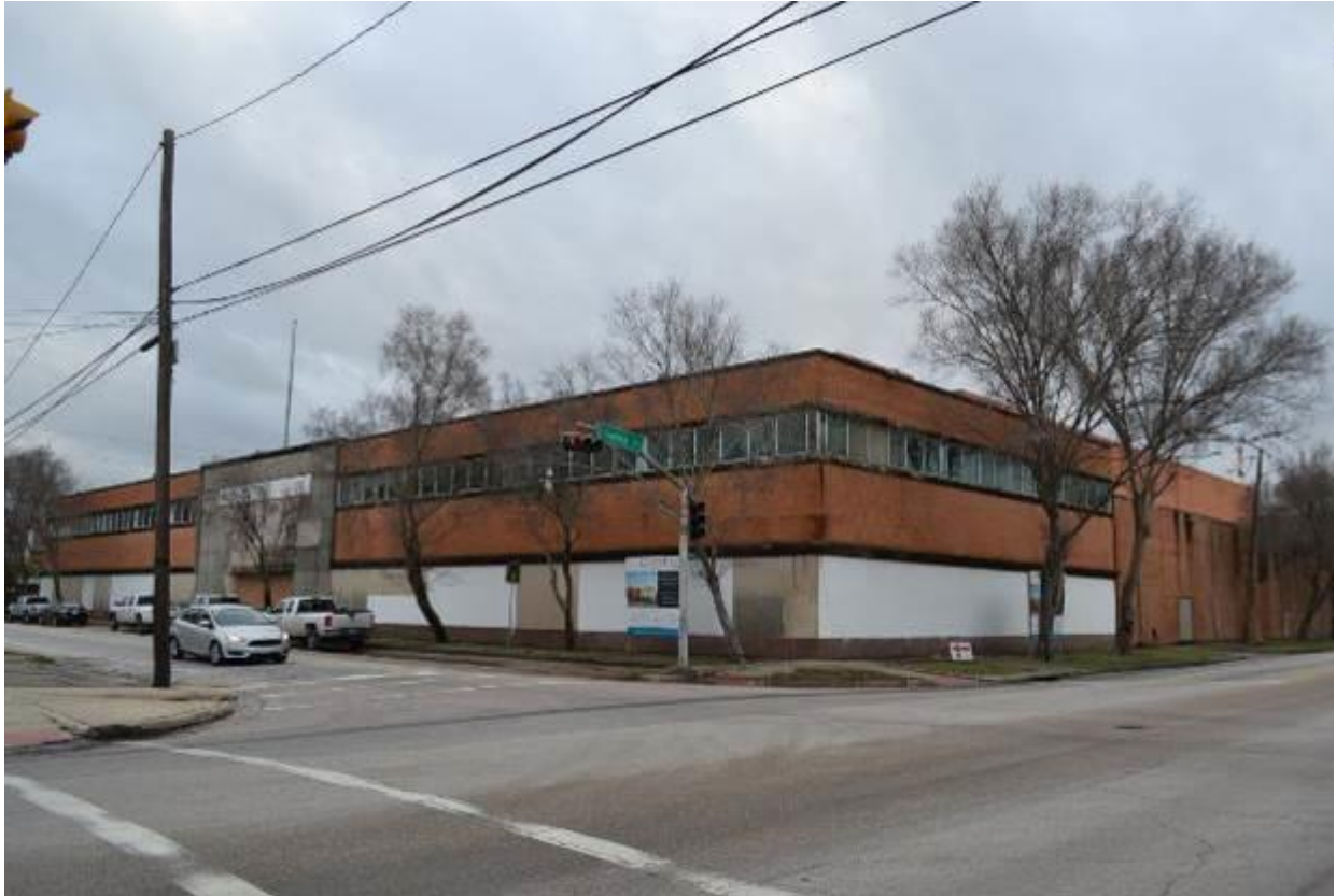
Photo 2 – North façade (L) and west elevation (R), view southeast.
