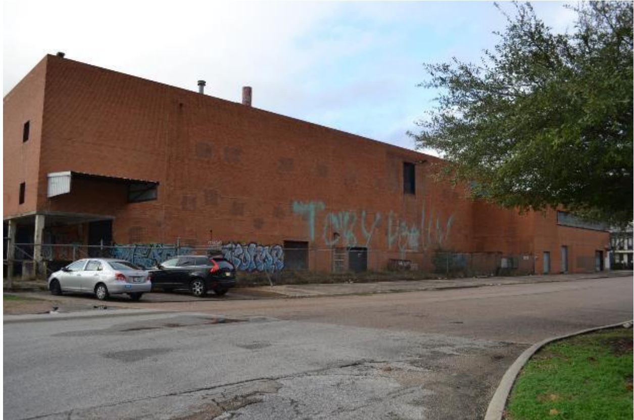
Photo 5 – East elevation, view northwest.
