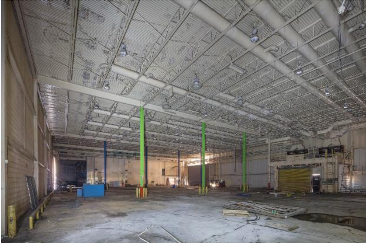
Photo 10 – Interior, 1972 metal warehouse addition, view northeast.
