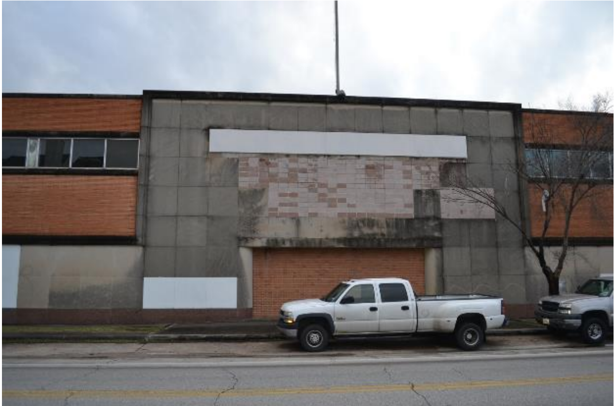
Photo 6 – Entrance detail on primary facade, view south.
