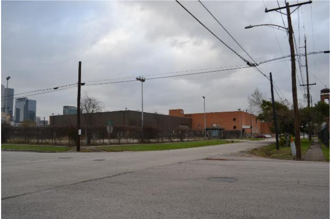
Photo 4 – South (L) and east (far R) elevations, view northwest.
