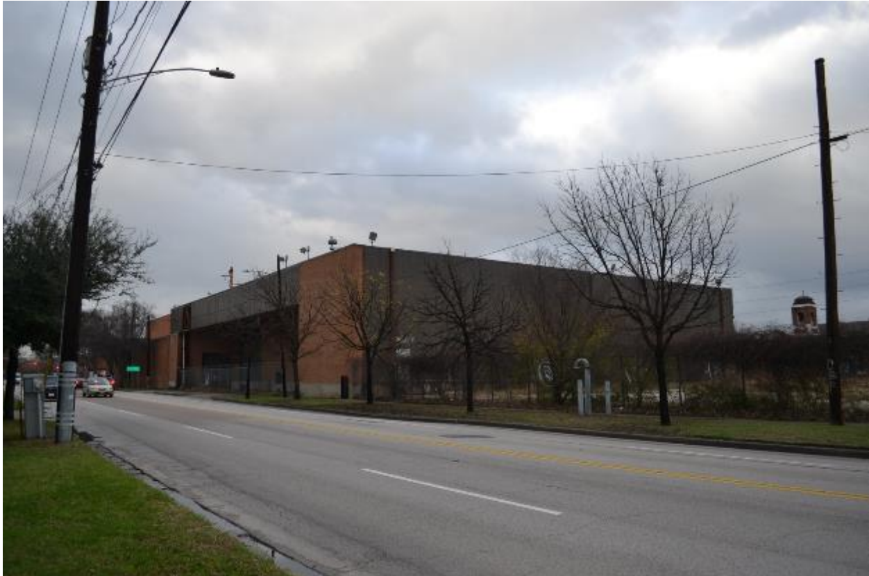
Photo 3 – West (L) and south (R) elevations, view northeast.
