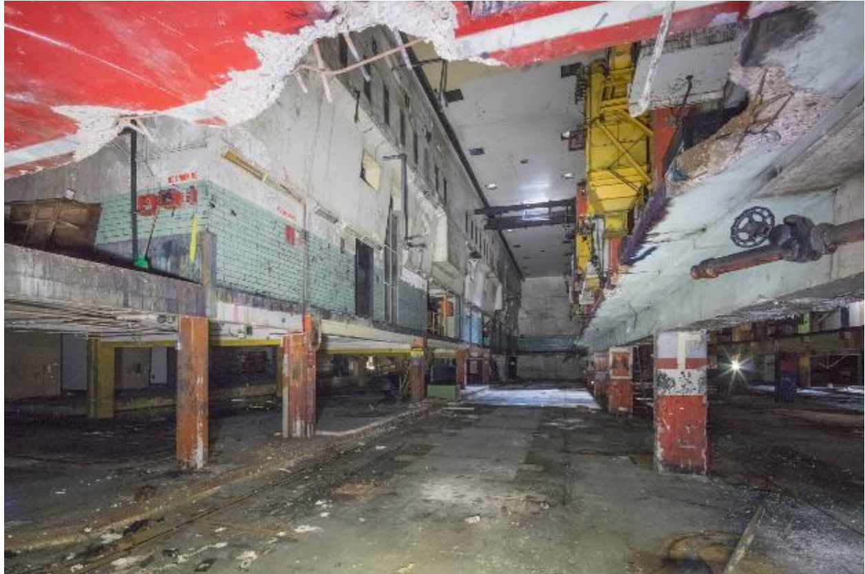
Photo 7 – Interior, press room printing bay, view south
