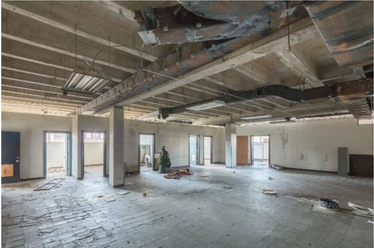
Photo 12 – Interior, second floor executive offices, view northwest.
