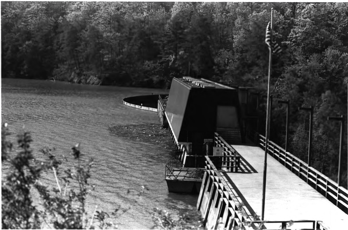
Ocoee Hydroelectric Station Parksville vicinity, Polk Co., TN
