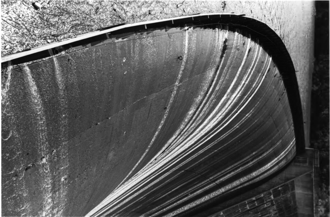
Oloee No. 1 Hydroelectric Station Parksville vicinity, Polk Co., TN
