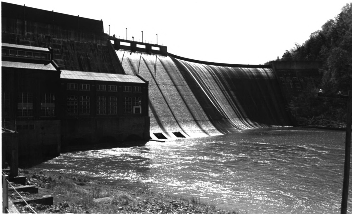
Ocoee No. 1 Hydroelectric Station Parkersville vicinity, Polk Co., TN
