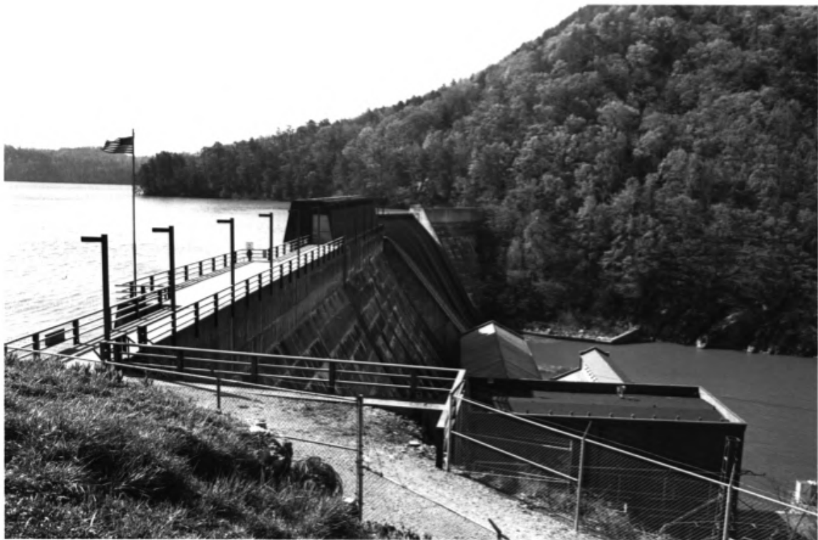
Ocoee Nat Hydroelectric Station Parkersville vicinity, Polk Co., TN.
