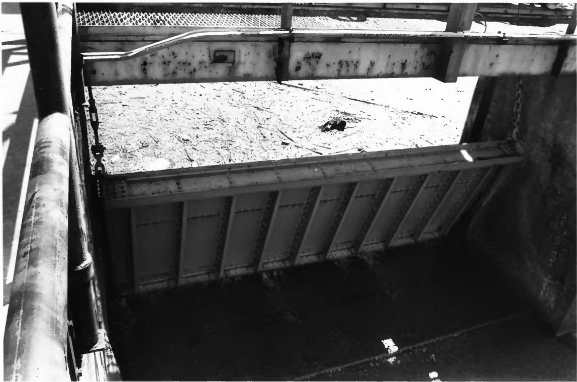
Ocoee No. 1 Hydroelectric Station Parkersville vicinity, Polk Co., TN
