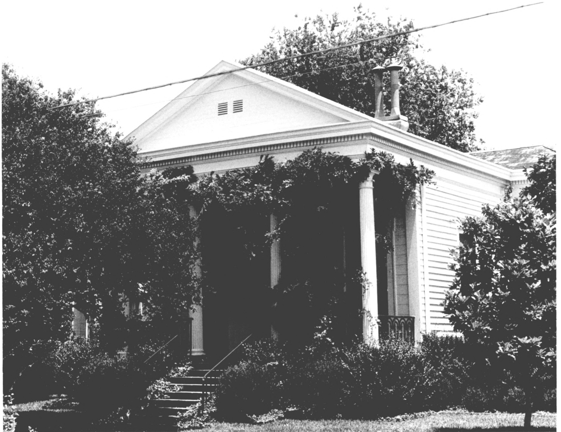
James H. Dillard House, New Orleans, Louisiana
