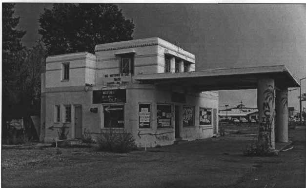
ATTACHMENT 4, Abandoned gas station in Longmont, Colorado, built c. 1925.
