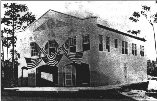
ATTACHMENT 1, Homestead Town Hall, c. 1917. Note the painted oculus motif in the pediment and painted squares in the frieze that recall the facade of the Church of Santa Maria Novella below.
