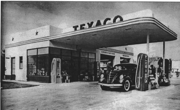
ATTACHMENT 3, Texaco gas station designed by Walter Dorwin Teague, c. 1935.
