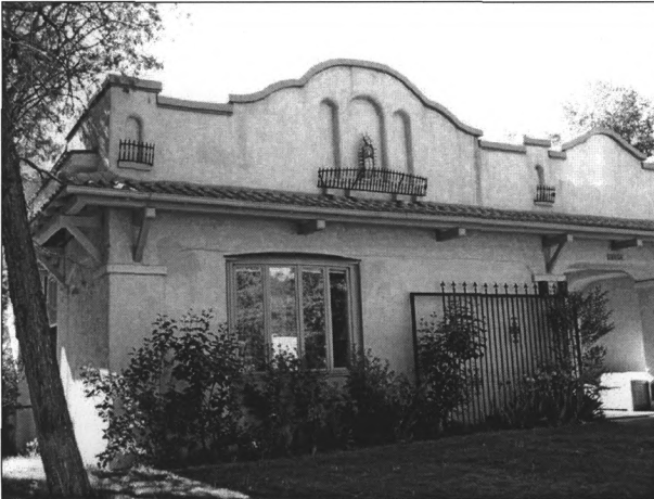
ATTACHMENT 5, variation of the mission style parapet on a Durango, Colorado residence, c. 1925.
