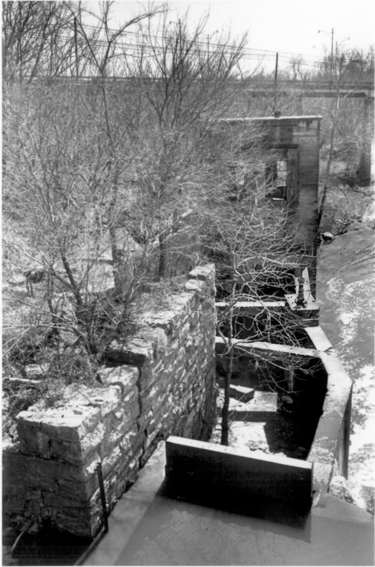
McMinville Hydroelectric Station McMinville, Warren County, TN
