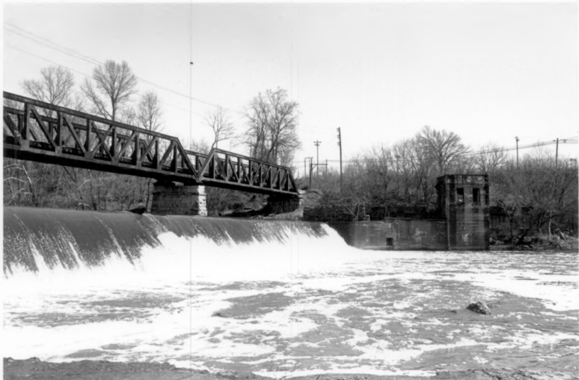
McMinnville Hydro electric Station McMinnville, Warren County, TN
