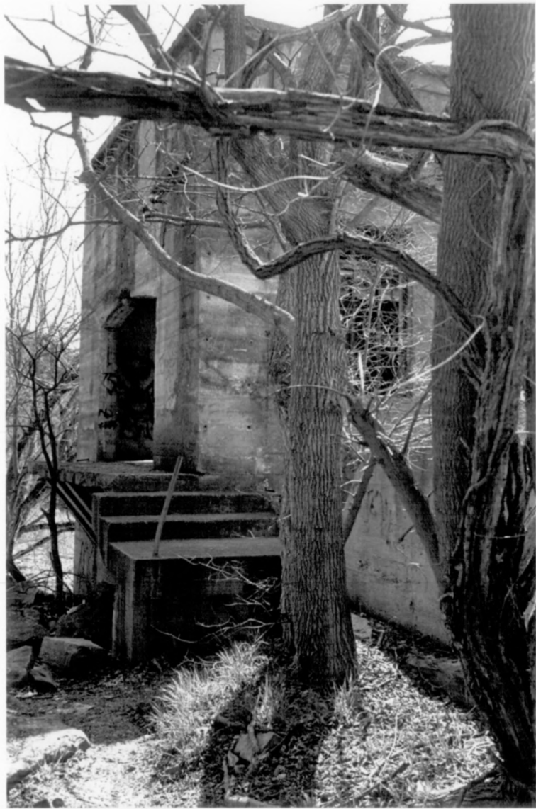
McMinnville Hydroelectric Station McMinnville, Warren County, TN
