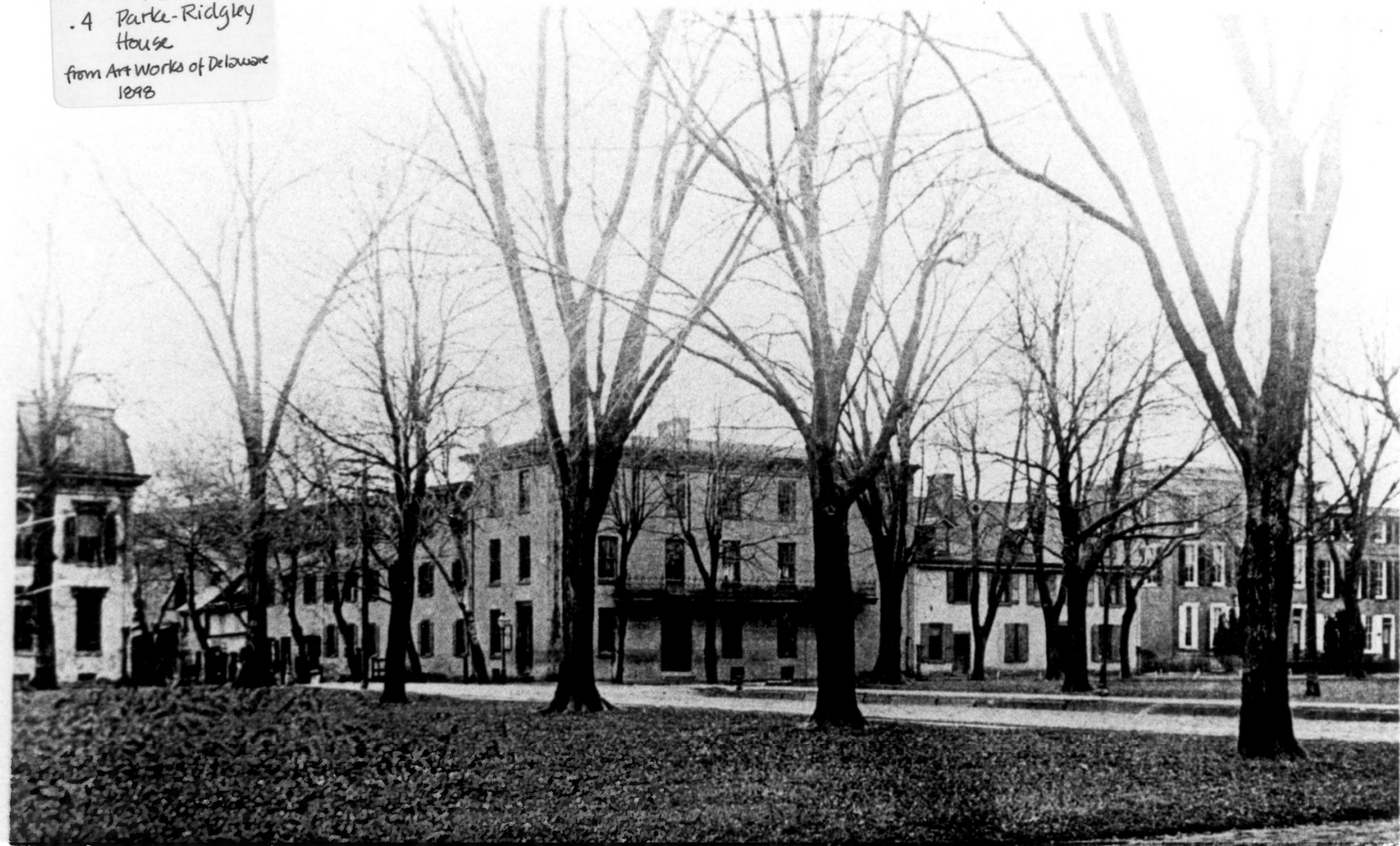
CAPITOL HOTEL AND OLD RIDGLEY HOUSE—DOVER, DELAWARE.
