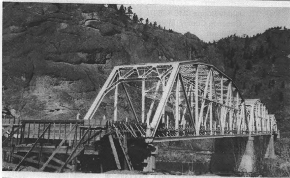
Photograph 0001. Hardy Bridge under construction. View to the northeast.
