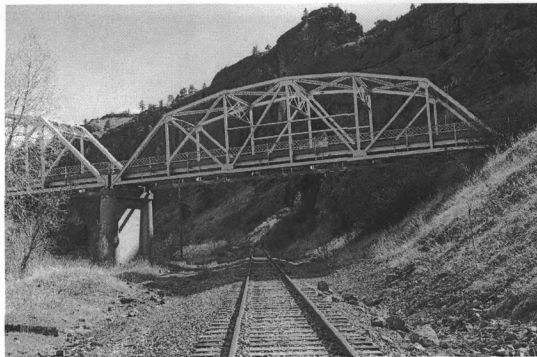
Photo 0004. Hardy Bridge. Railroad span. View to the southwest.
