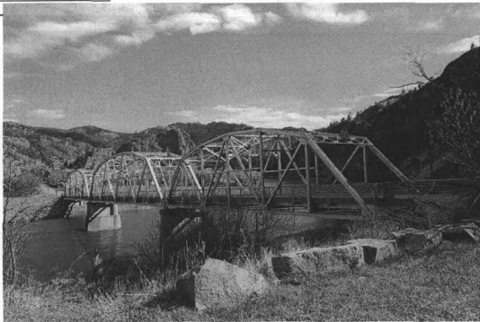
Photo 0003. Hardy Bridge. North side. View to the south-southeast.
