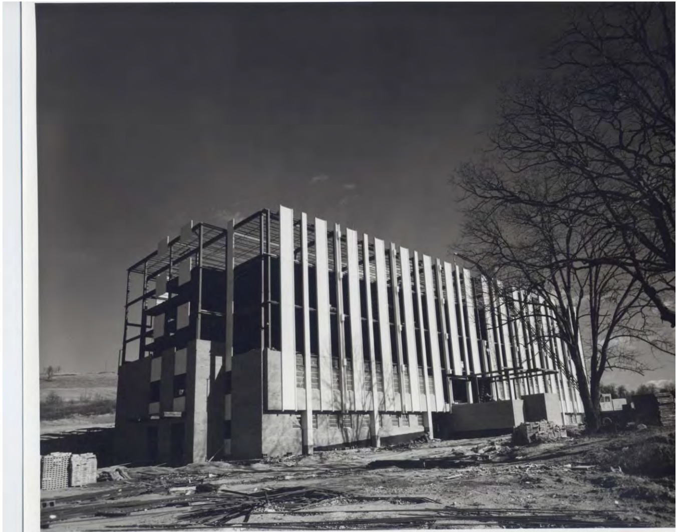
Figure 2. 1965 Photo of Smyth County Community Hospital Under Construction – Original South Façade and West Wall.
