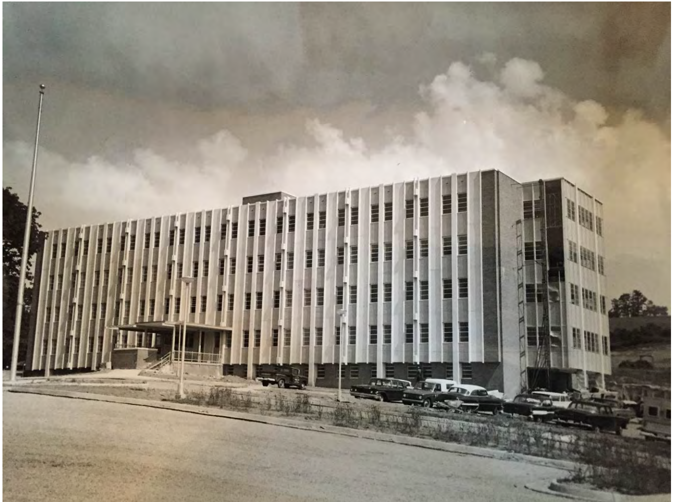
Figure 7. 1967 Photo of Smyth County Community Hospital at Its Opening.
