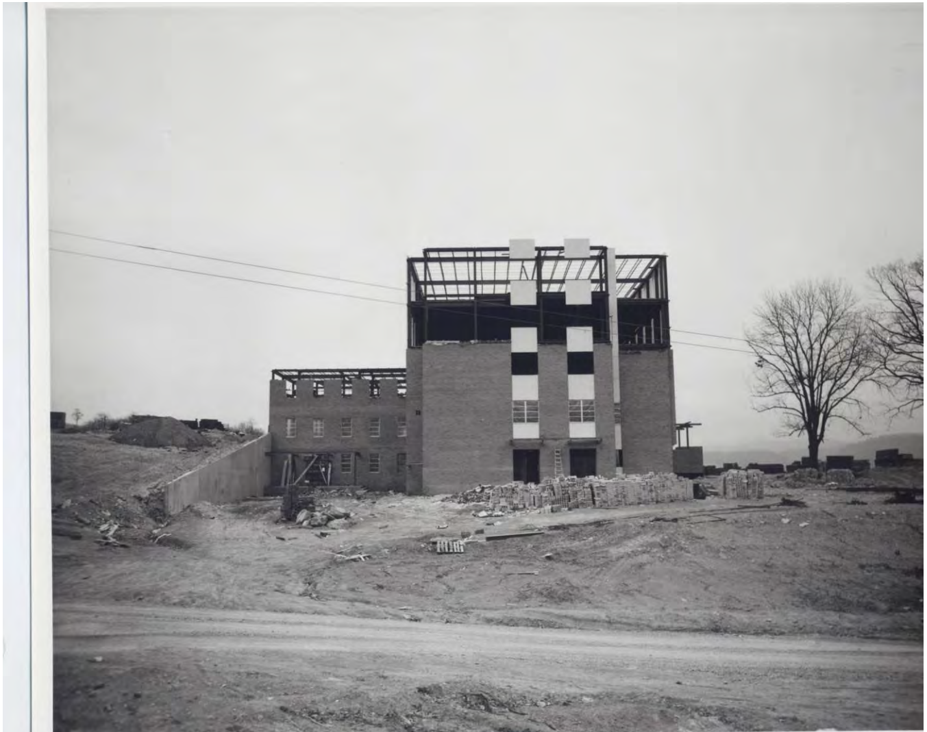
Figure 4. 1965 Photo of Smyth County Community Hospital Under Construction – Original West Wall.
