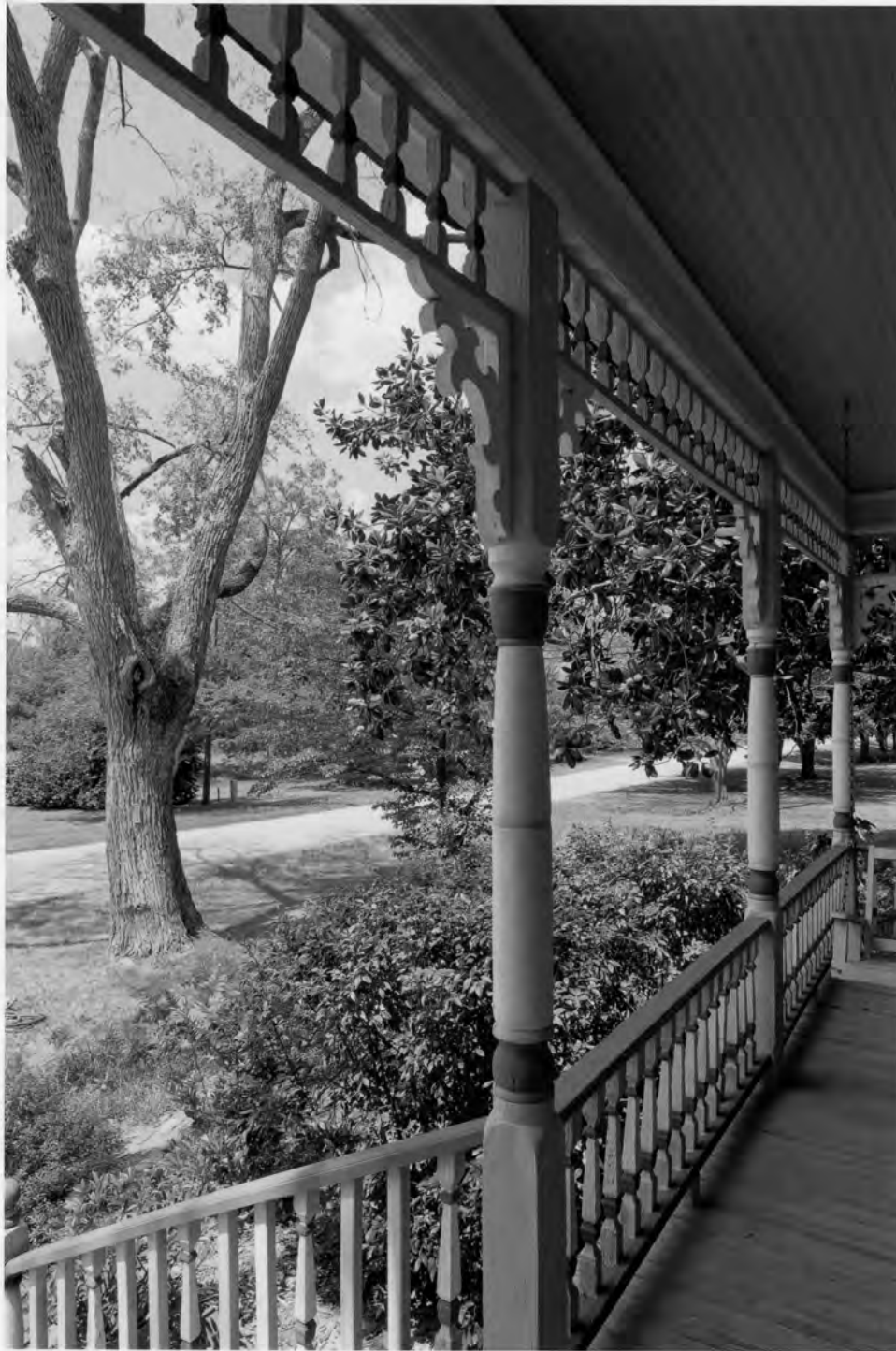
Davis-Proctor House Emanuel County, Georgia Photograph 11 of 21
