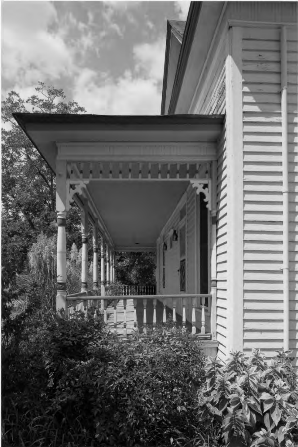
Davis-Proctor House Emanuel County, Georgia Photograph 10 of 21
