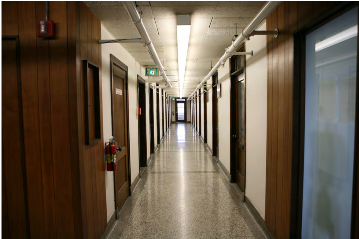
Photograph 14 of 18: Interior view, 6th floor double-loaded corridor, looking northwest. Typical corridor arrangement found on floors 2-6. The 6th floor corridor showcases the original terrazzo floors.
