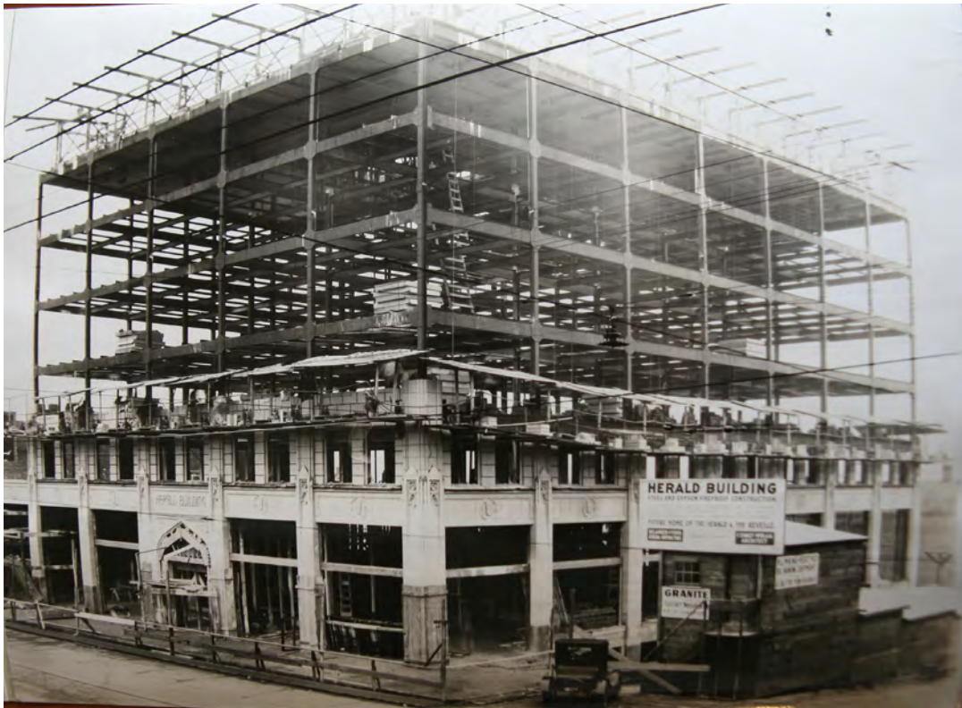
1925-26 view of completed steel structure and terra cotta going up at the 2nd floor, looking west. Source: Bellingham Herald's Jack Carver Collection, Whatcom Museum of History and Art, Bellingham, WA. Courtesy Daylight Properties.
