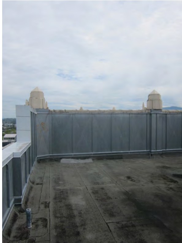
Photograph 17 of 18: View of roof and parapet, looking northeast.
