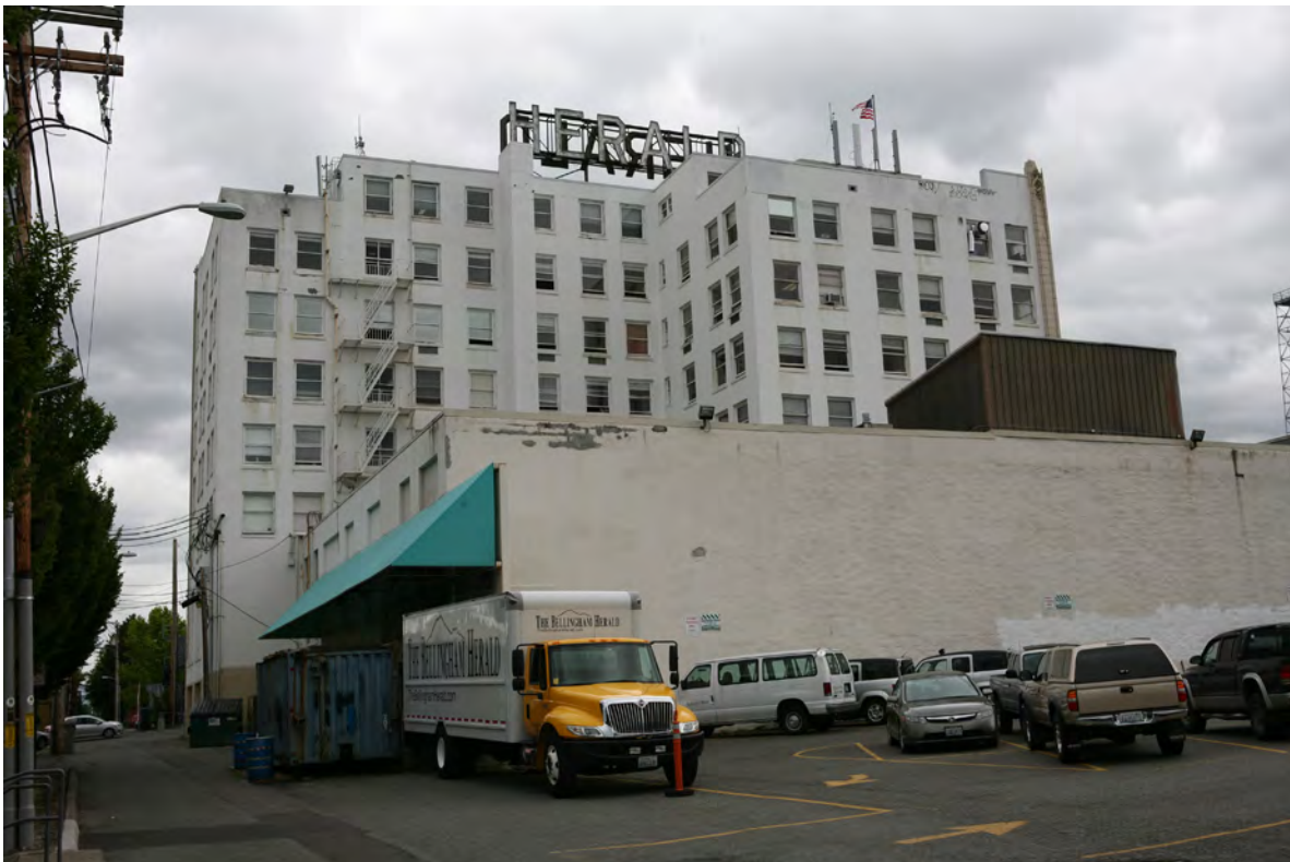
Photograph 4 of 18: View of southwest facade.
