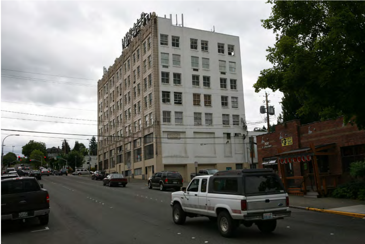
Photograph 3 of 18: View of northeast and northwest facades.
