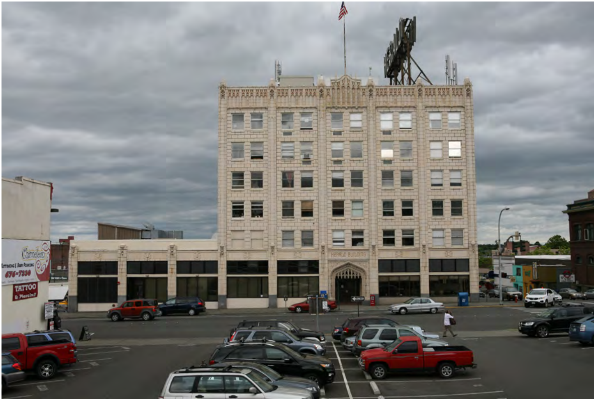
Photograph 1 of 18: View of southeast facade.
