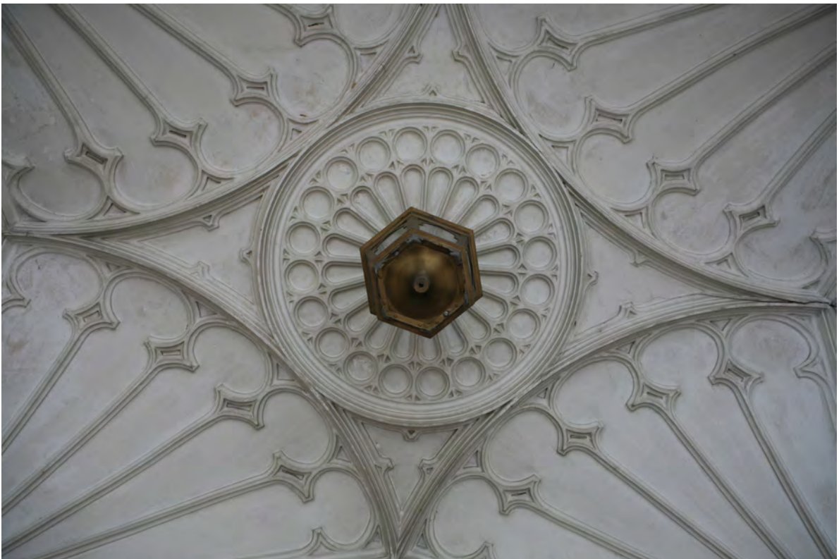
Photograph 8 of 18: Detail of covered vault ceiling in the entry vestibule.
