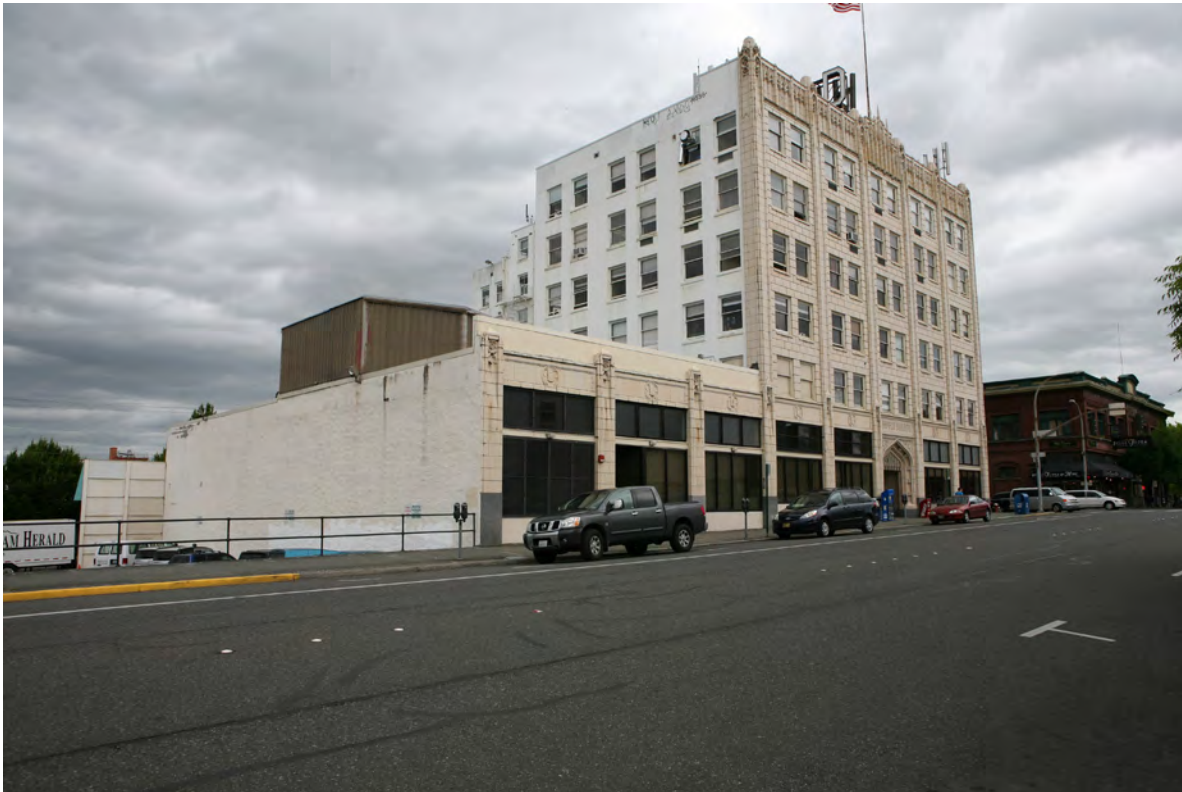
Photograph 5 of 18: View of southwest and southeast facades.
