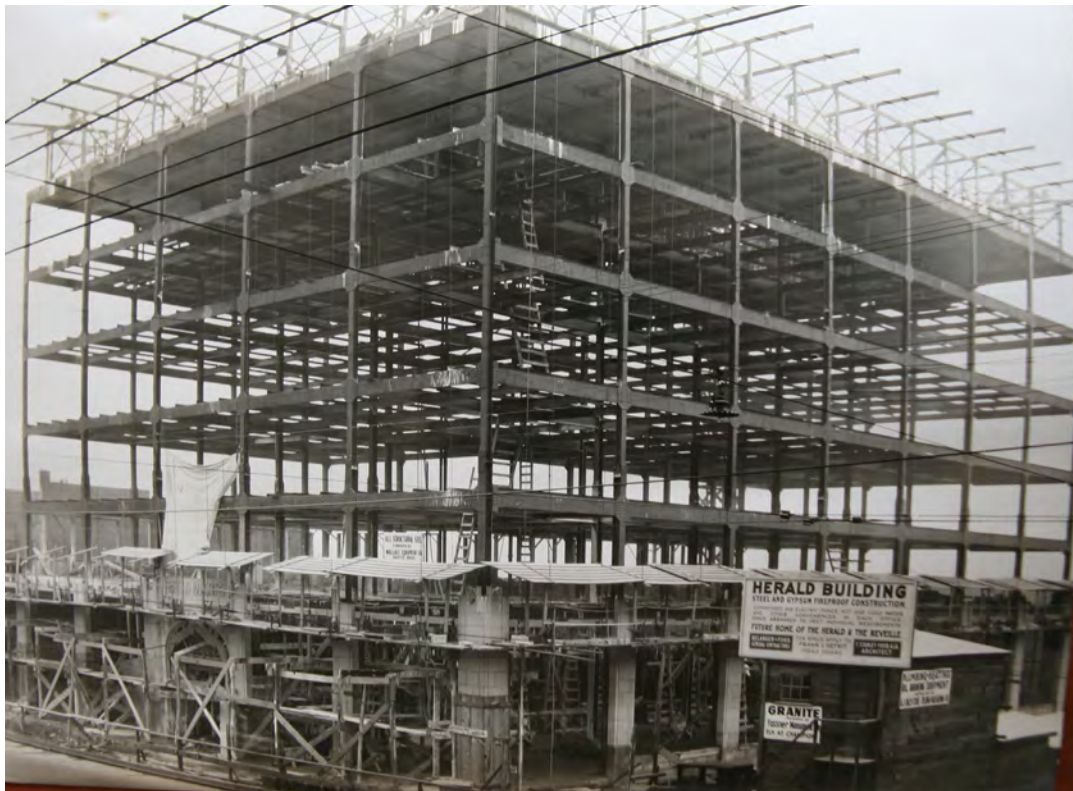
1925-26 view of completed steel structure and terra cotta going up at the 2nd floor, looking west. Source: Bellingham Herald's Jack Carver Collection, Whatcom Museum of History and Art, Bellingham, WA. Courtesy Daylight Properties.
