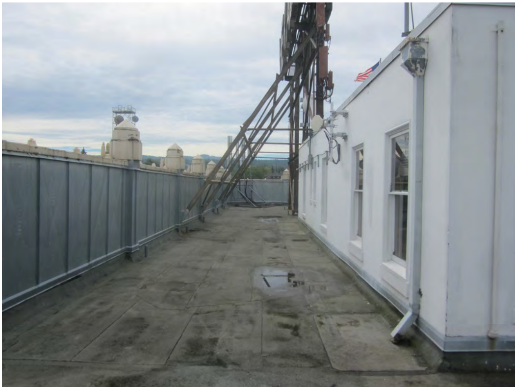
Photograph 18 of 18: View of roof, looking southeast.
