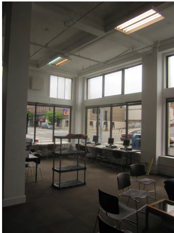
Photograph 12 of 18: View of former Herald Business Office, looking east.
