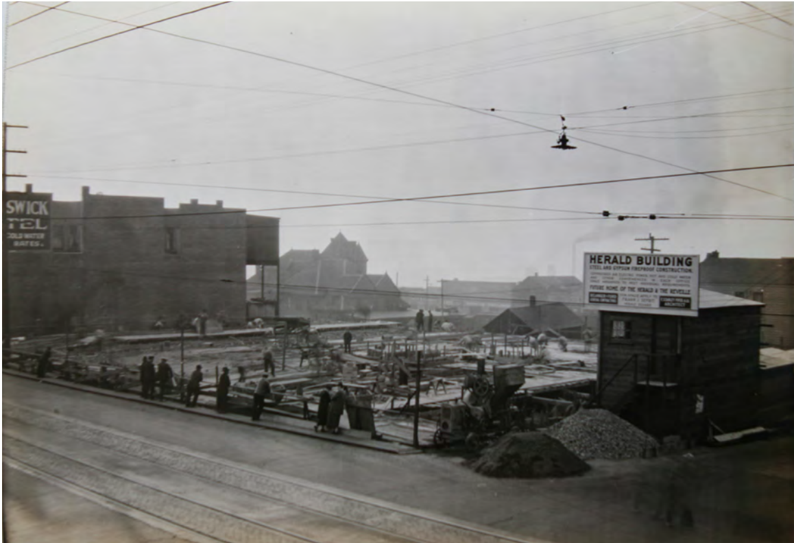
1925 view of foundation work on Herald Building, looking west. Source: Bellingham Herald's Jack Carver Collection, Whatcom Museum of History and Art, Bellingham, WA. Courtesy Daylight Properties.
