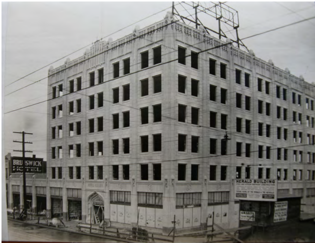
1925-26 view of construction in progress, upper story windows not yet in place. Source: Bellingham Herald's Jack Carver Collection, Whatcom Museum of History and Art, Bellingham, WA. Courtesy Daylight Properties.
