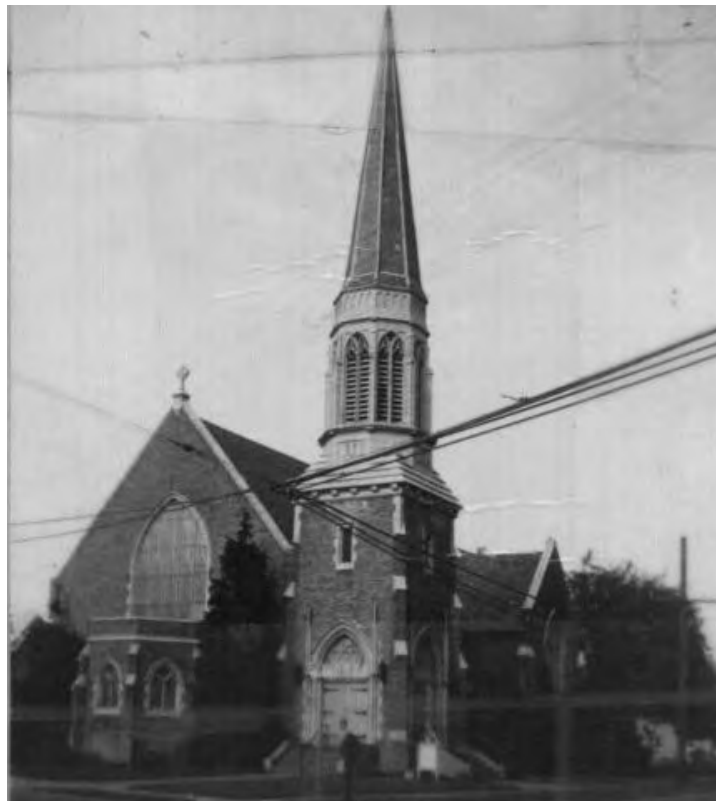
Undated view of St. Paul's Episcopal Church, Bellingham. Source: Whatcom County Assessor.
