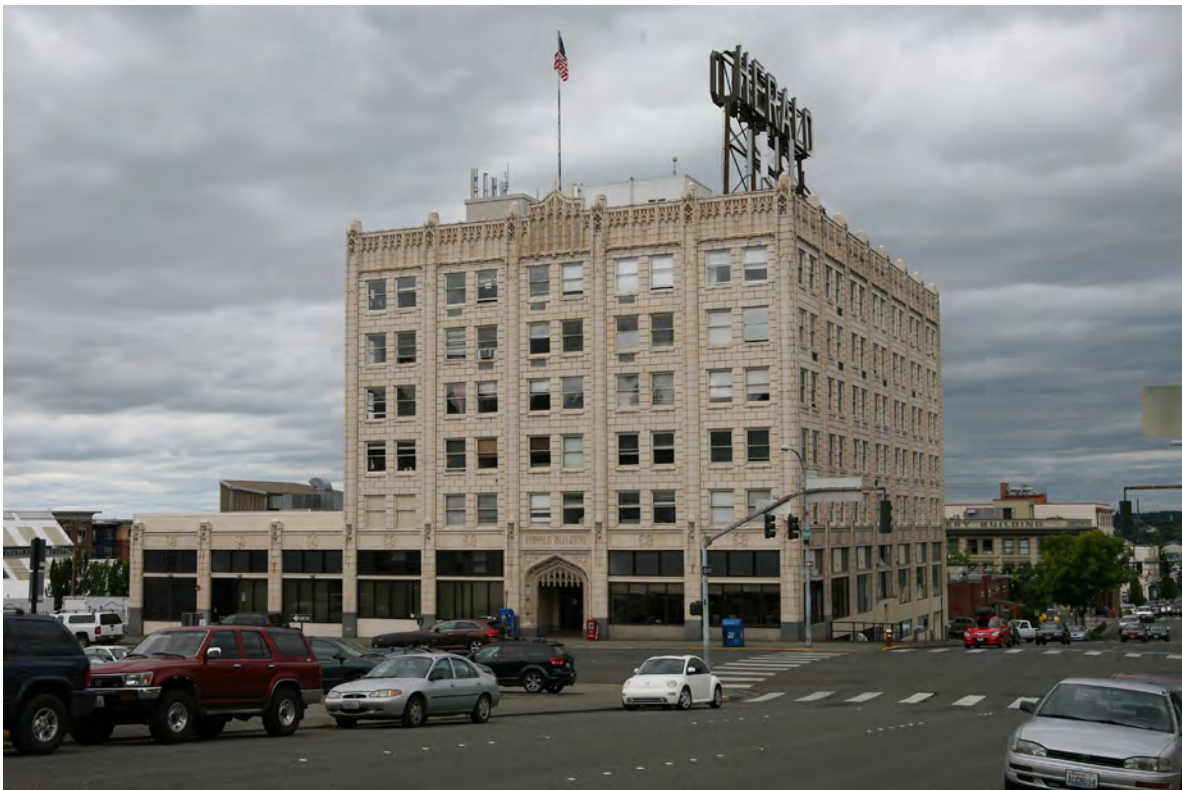
Photograph 2 of 18: View of southeast and northeast facades.
