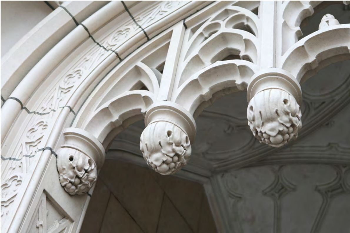
Photograph 7 of 18: Detail of finials and tracery present at main entrance.
