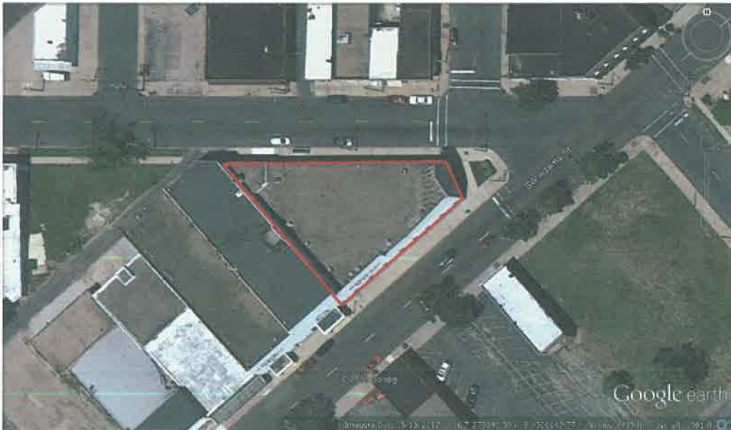
Figure 12. 2201 SW Adams St., Peoria, Illinois. Aerial view.
