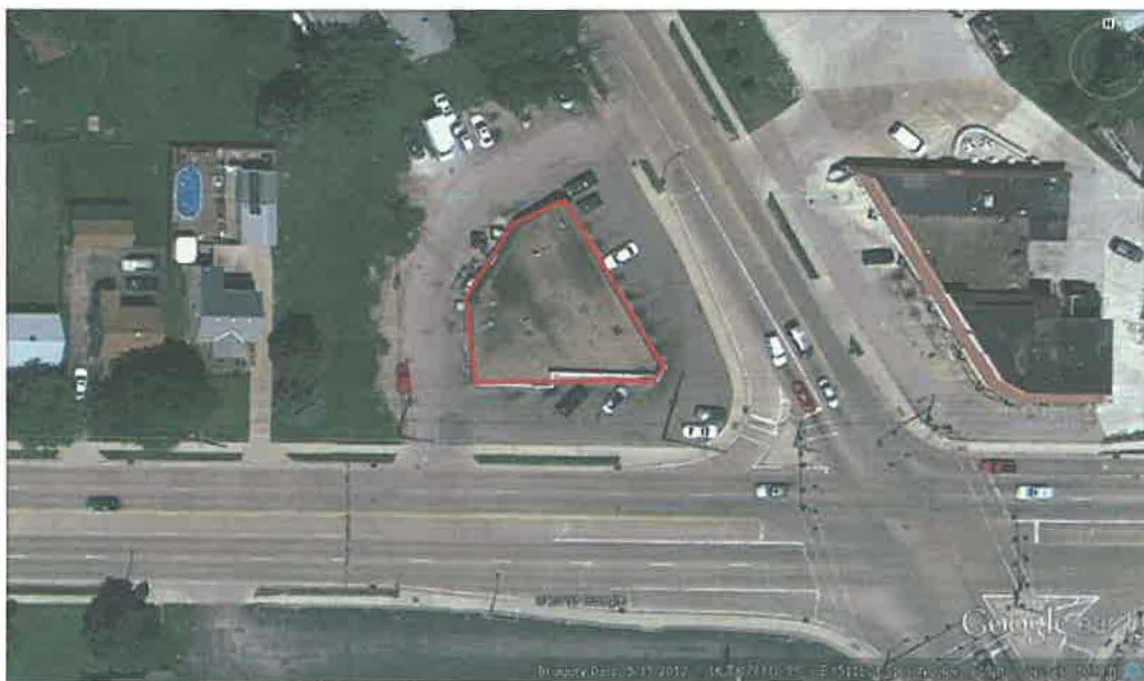
Figure 22. 2009 W. Forrest Hill Ave., Peoria, Illinois. Aerial view.
