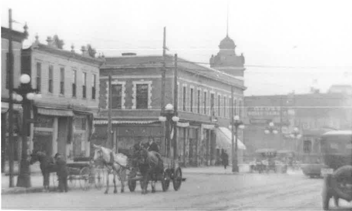
Figure 5. Kickapoo Building, corner of Glendale Avenue and Main Street (n.d.).
