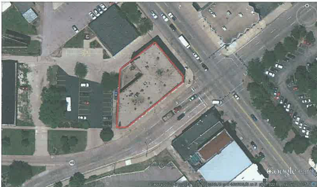
Figure 24. 701 W. Main St., Peoria, Illinois. Aerial view.
