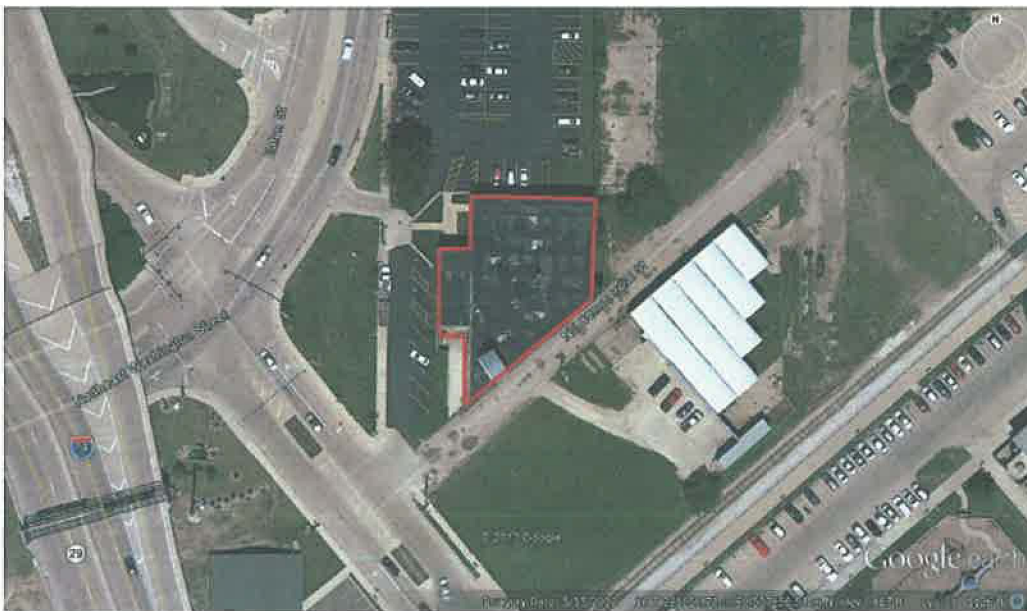
Figure 28. 120 Eaton St., Peoria, Illinois. Aerial view.
