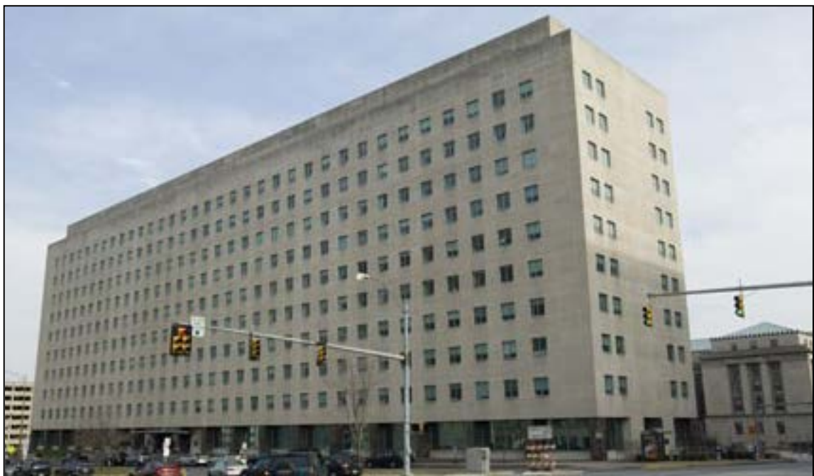
Figure 7: Health and Welfare Building, Capitol Park Extension, Harrisburg Completed 1956/7 Architect: Lacey, Atherton and Davis (Harrisburg, Wilkes-Barre)
