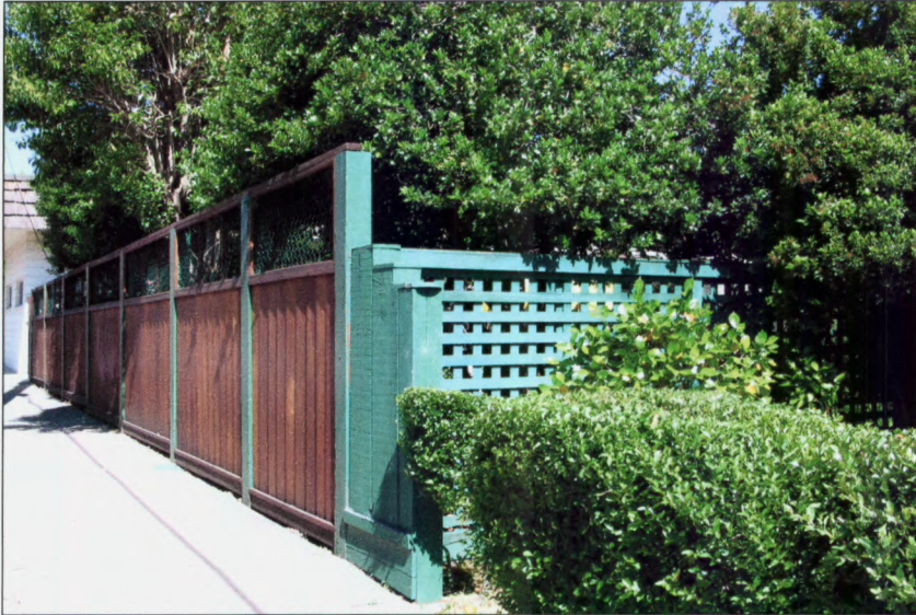
A. Redwood fence along Mendocino Street at Dr. Raymond Babcock Home. Facing (North) West.
