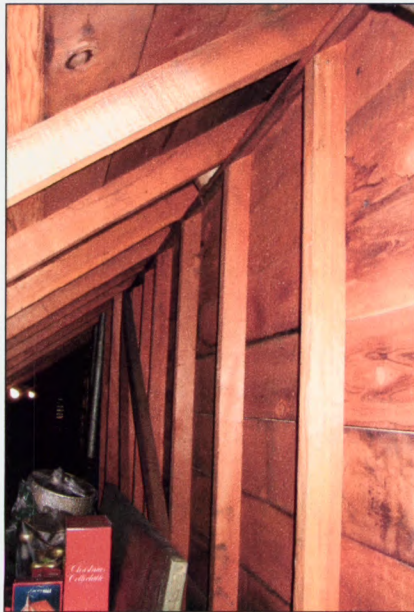
B. Redwood also visible in eaves of the attic in Dr. Raymond Babcock Home.
