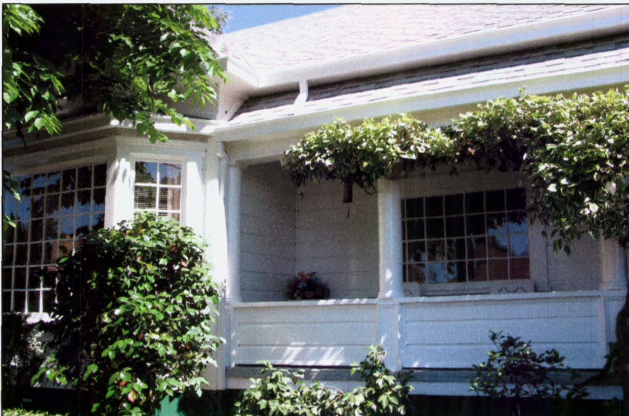
B. Mendocino Street Side of home showing dining room bay and veranda with its roof detail. Facing north.
