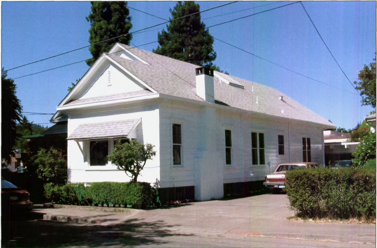
Front and driveway of Dr. Raymond Babcock Home. Showing double gable and soffits. Facing Southwest.
