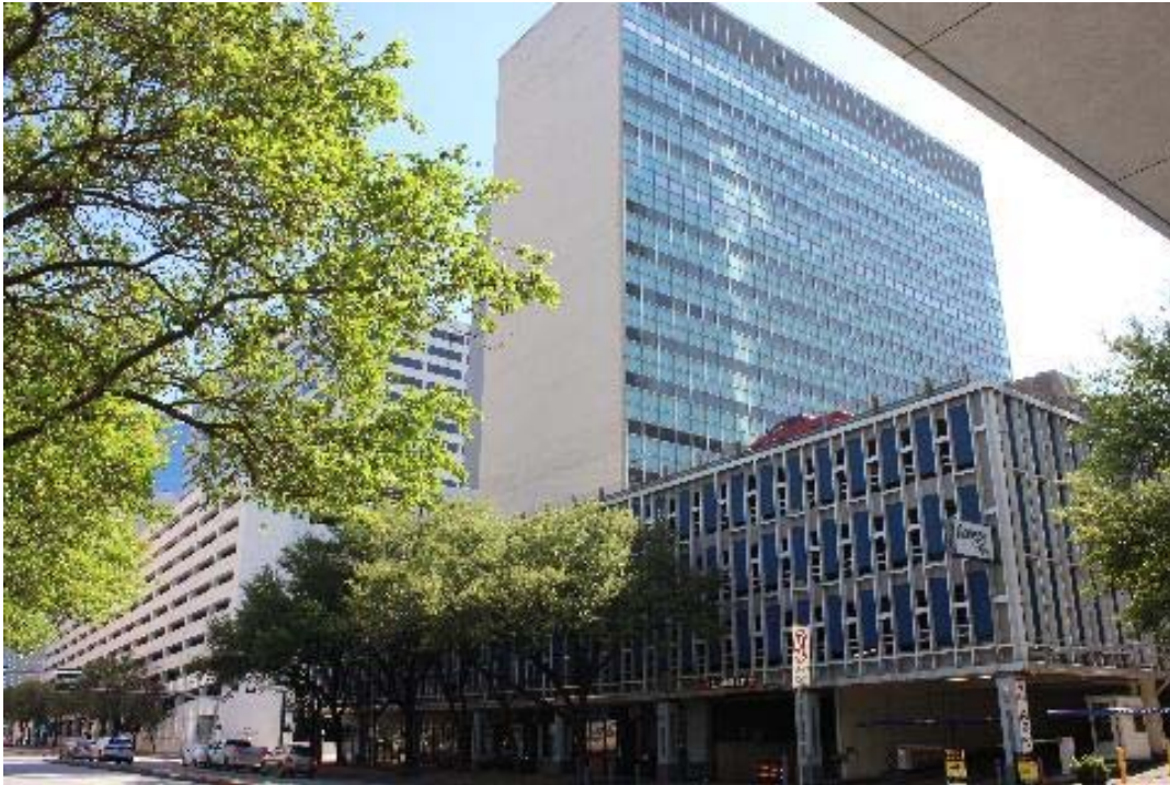
Photo: TX_Harris County_Medical Towers_0002
