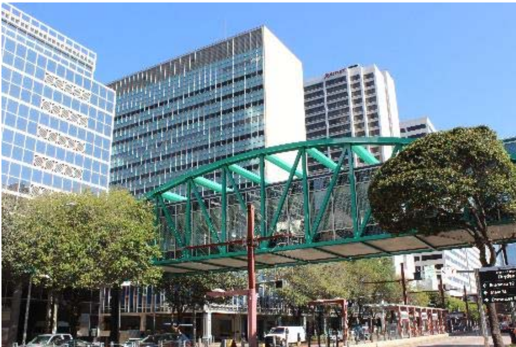
Photo: TX_Harris County_Medical Towers_0003
