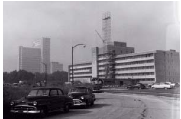
Figure 32 – St. Luke's Hospital, 1953
