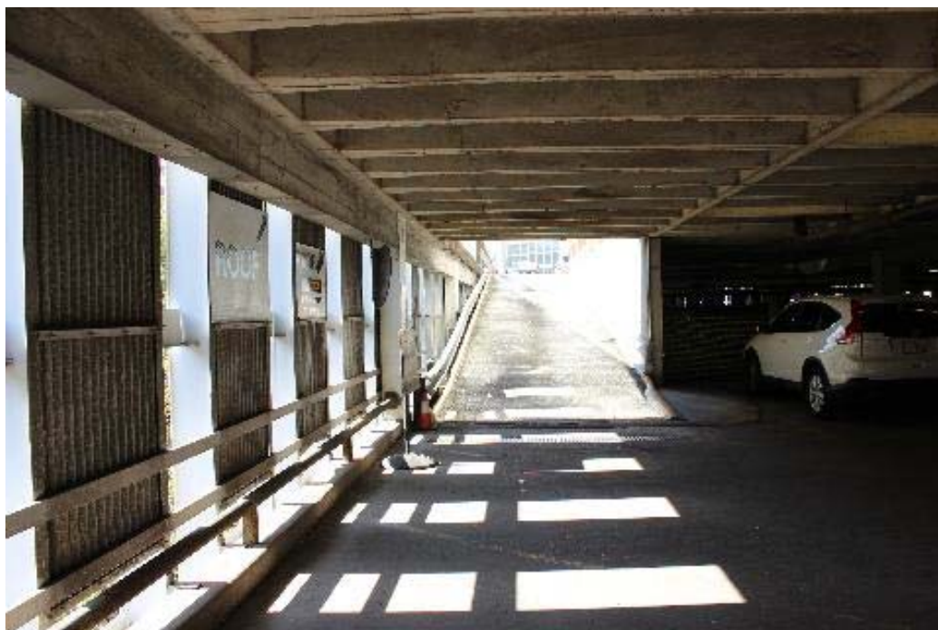
Photo: TX_Harris County_Medical Towers_0011
