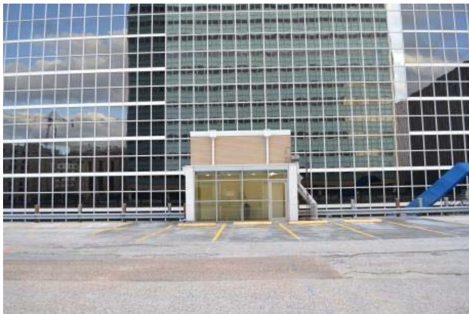
Photo: TX_Harris County_Medical Towers_0014
