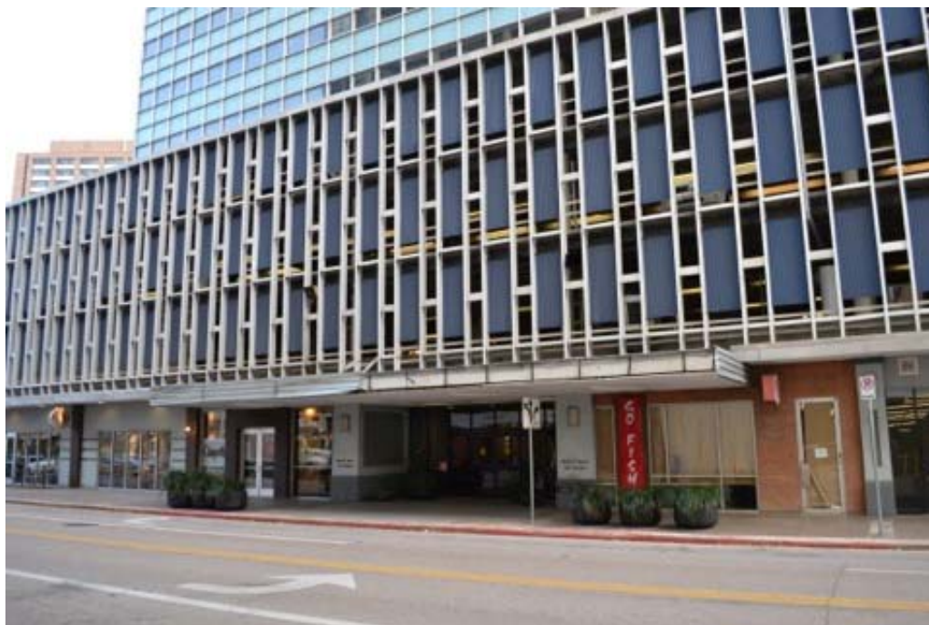
Photo: TX_Harris County_Medical Towers_0004
