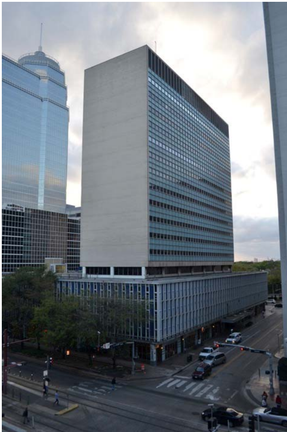
Photo: TX_Harris County_Medical Towers_0001
