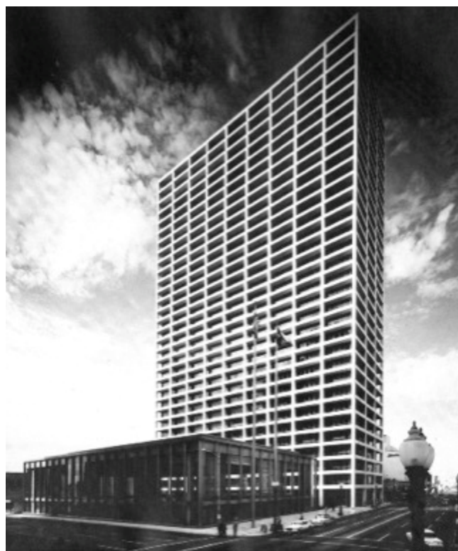
Figure 22 – First City National Bank, 1960 Source:
