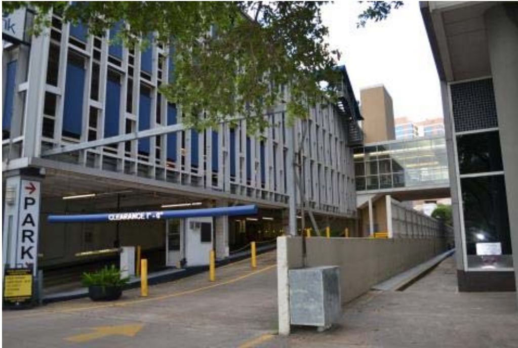
Photo: TX_Harris County_Medical Towers_0012
