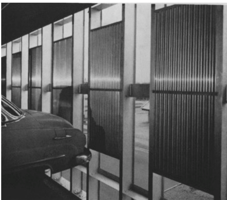
Figure 9 – Medical Towers Parking Garage Interior
