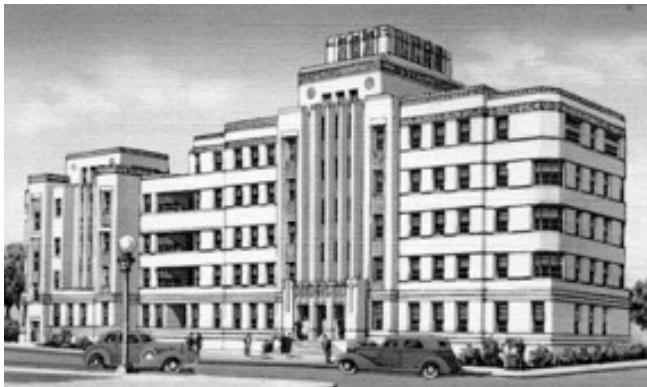
Figure 15 – St. Joseph Infirmary Maternity and Children's Building, 1940 Source: Collection of Randy Pace, Houston, Texas
