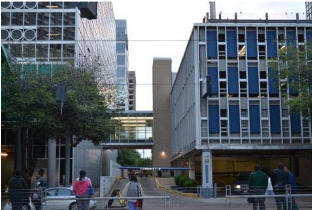
Photo: TX_Harris County_Medical Towers_0013
