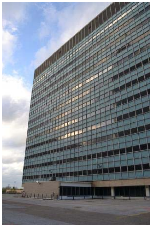
Photo: TX_Harris County_Medical Towers_0015
