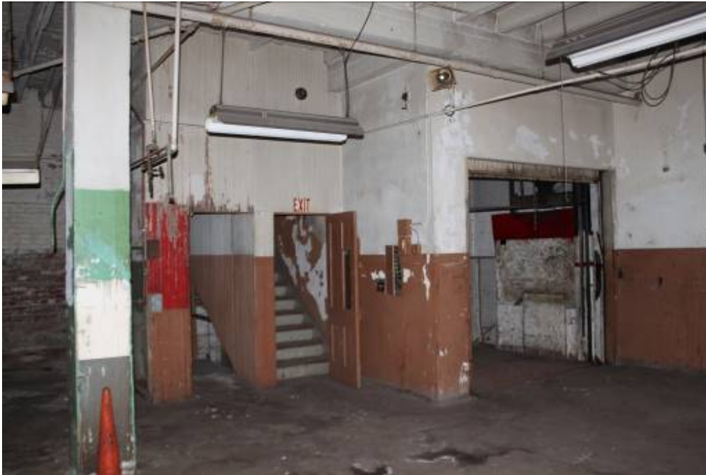
Photo 9: Main level, second room, freight elevator and staircase.
