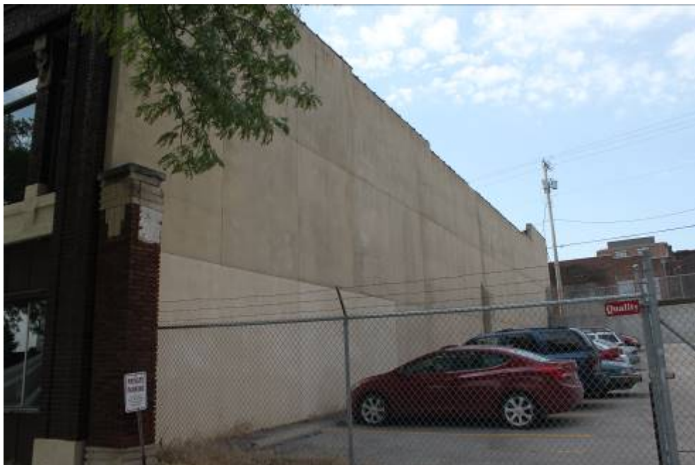
Photo 4: West facing wall and parking lot.
