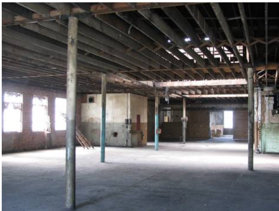
Photo 12: Upper level, facing south towards Harney Street.
