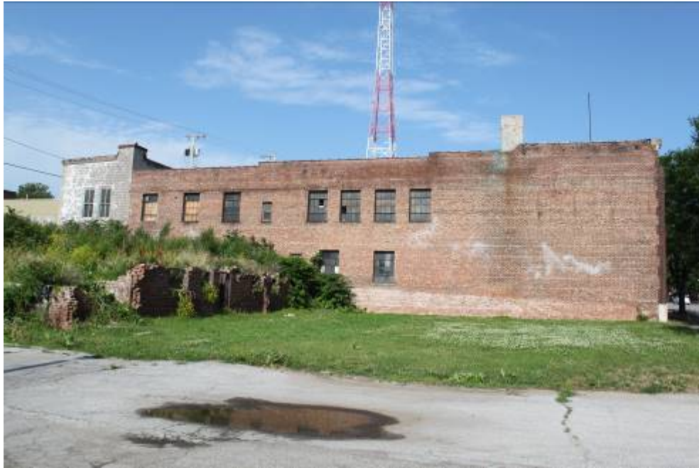
Photo 3: East facing wall.
