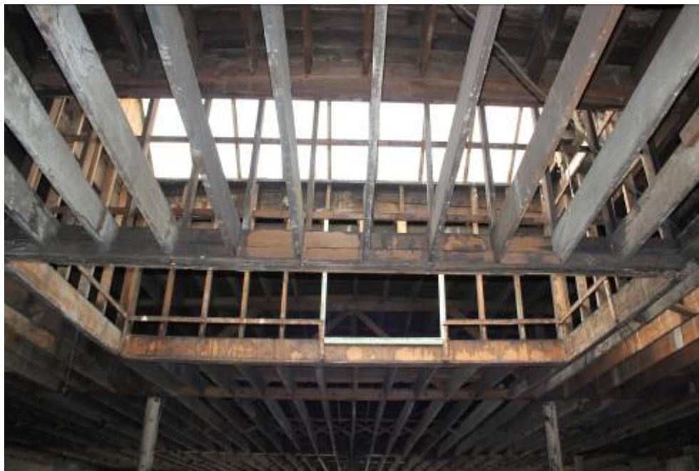
Photo 13: Upper level, skylight and ceiling joints
