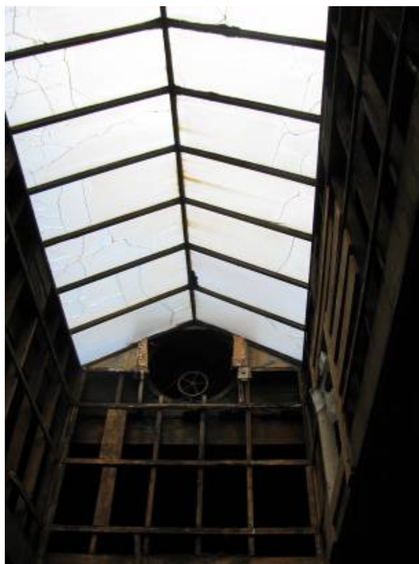
Photo 14: Upper level, skylight.
