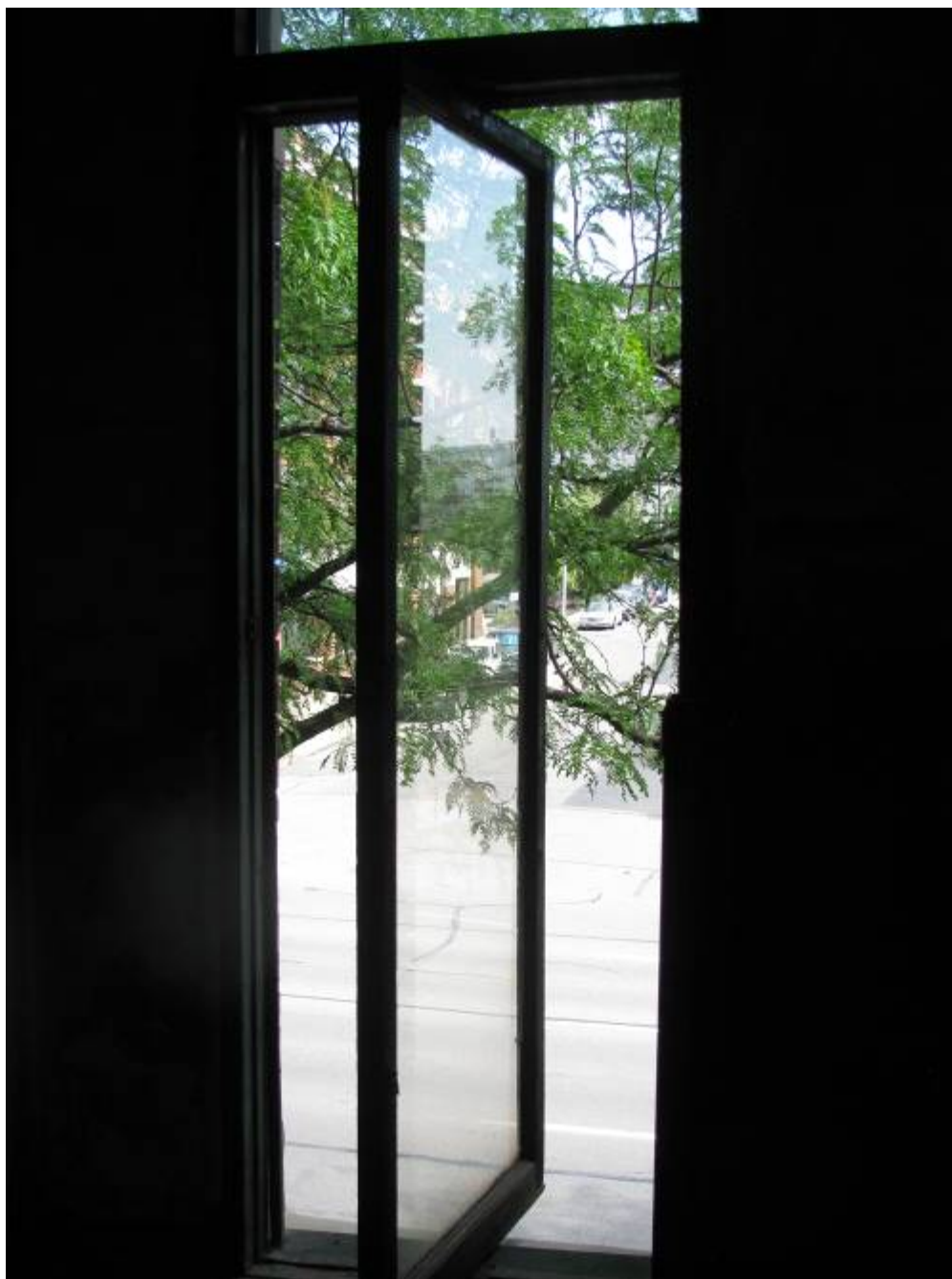
Photo 15: Upper level, center-pivot operating wood window sashes overlooking Farnam Street.
