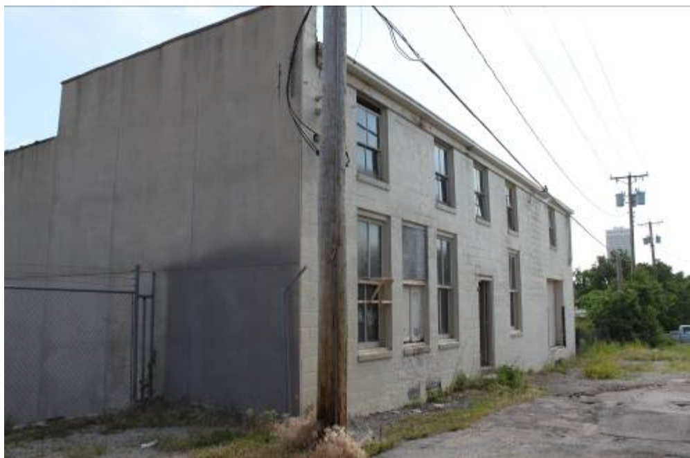
Photo 5: Rear facing south, alley leads to Harney Street.
