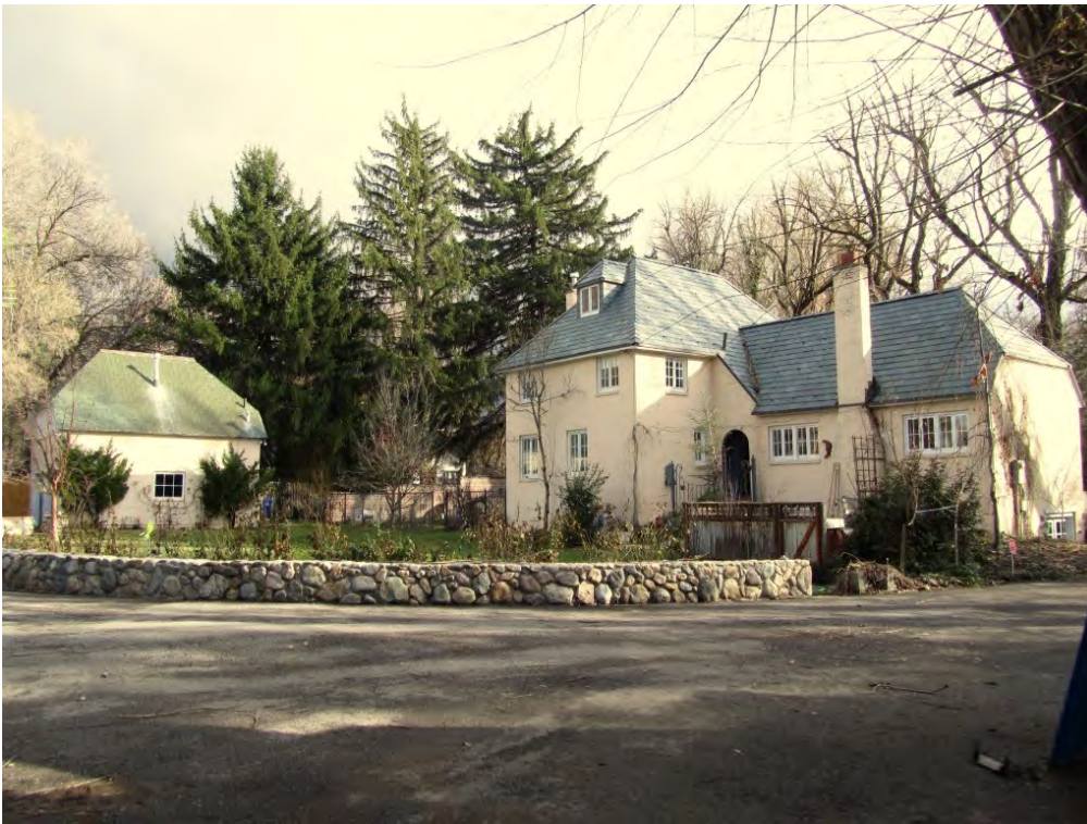
Photograph 8 of 19. Setting, camera facing southeast.
