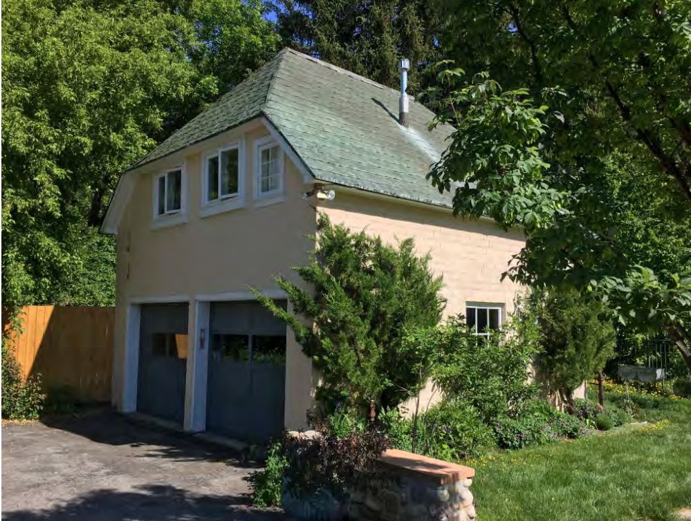
Photograph 7 of 19. North and west elevation. Camera facing southeast.
