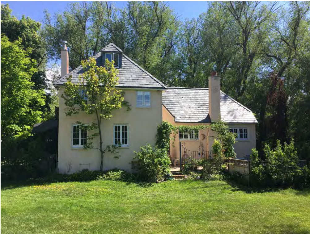
Photograph 4 of 19. North elevation. Camera facing south.
