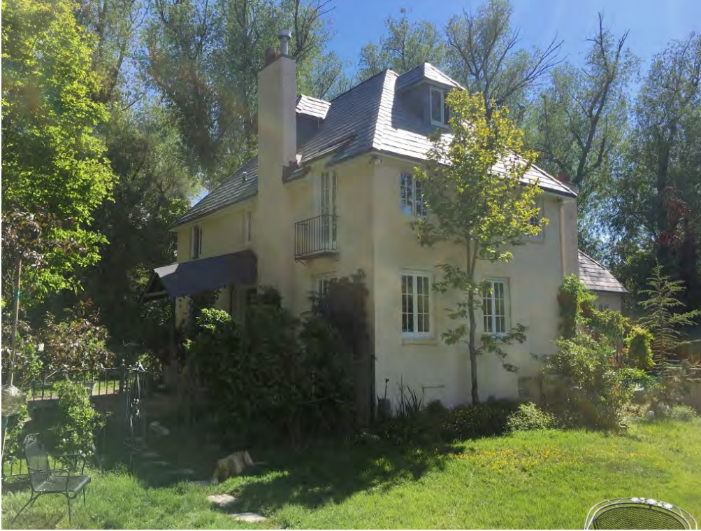
Photograph 3 of 19. East and north elevations. Camera facing southwest.
