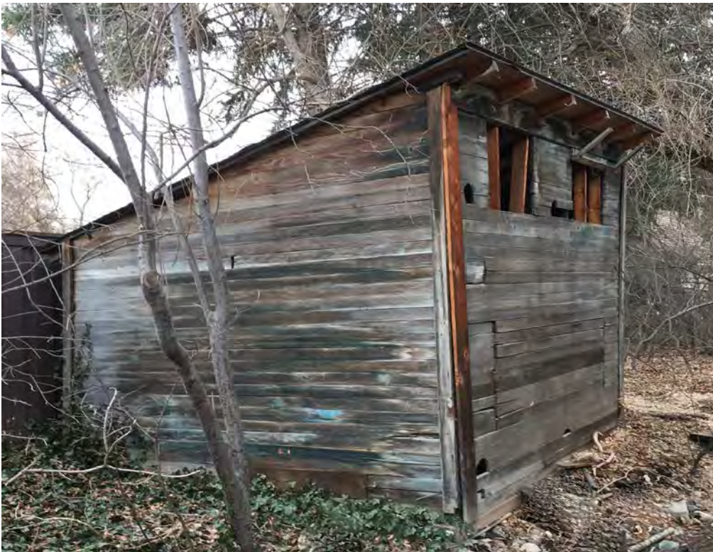
Photograph 10 of 19. Coop, camera facing northeast.
