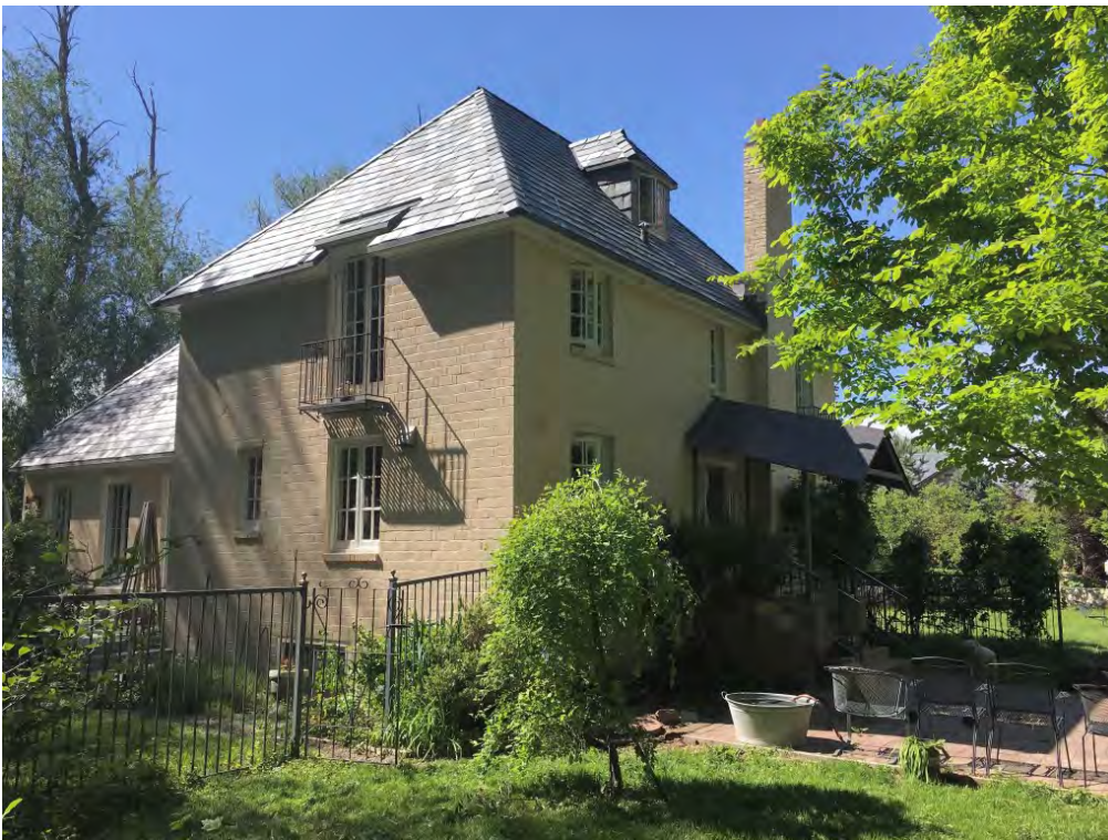
Photograph 2 of 19. South and east elevations. Camera facing northwest.
