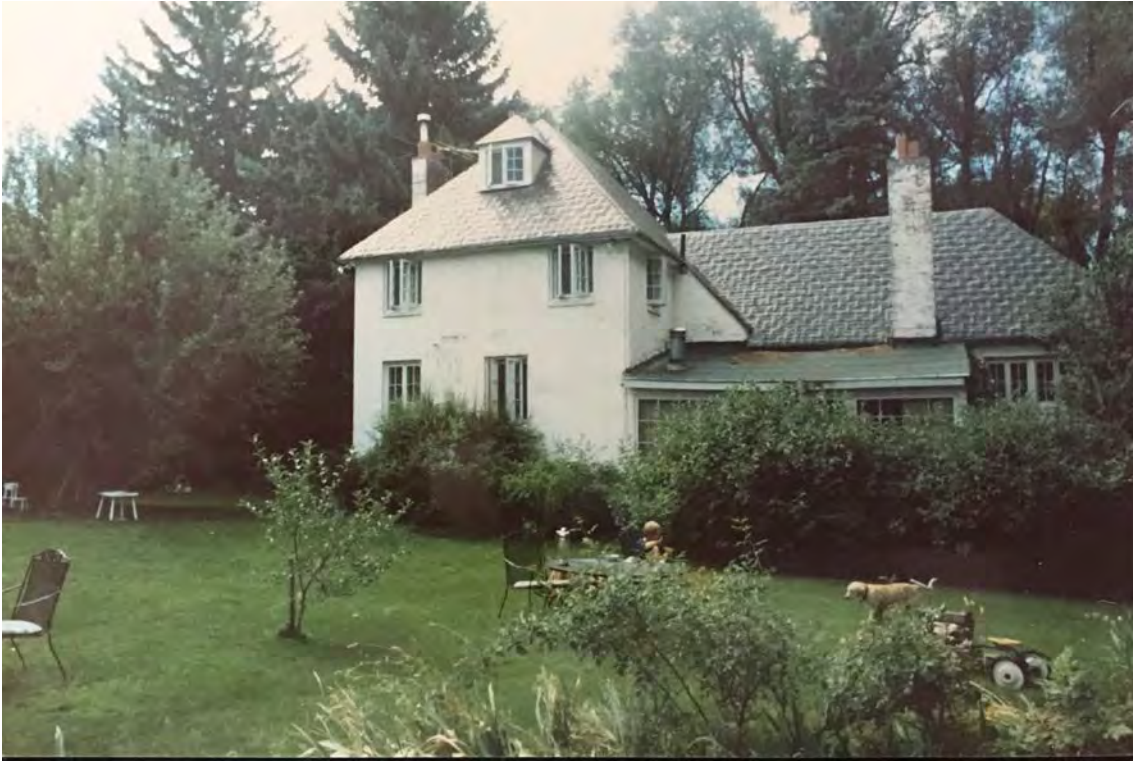
Figure 5 of 6. Photo taken in 1988 of the north facade showing the former screened porch and the former copper roof.
