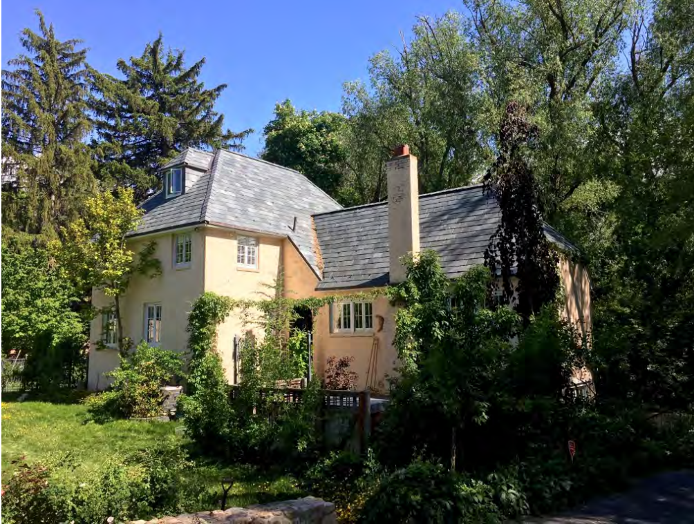
Photograph 5 of 19. North and west elevation. Camera facing southeast.
