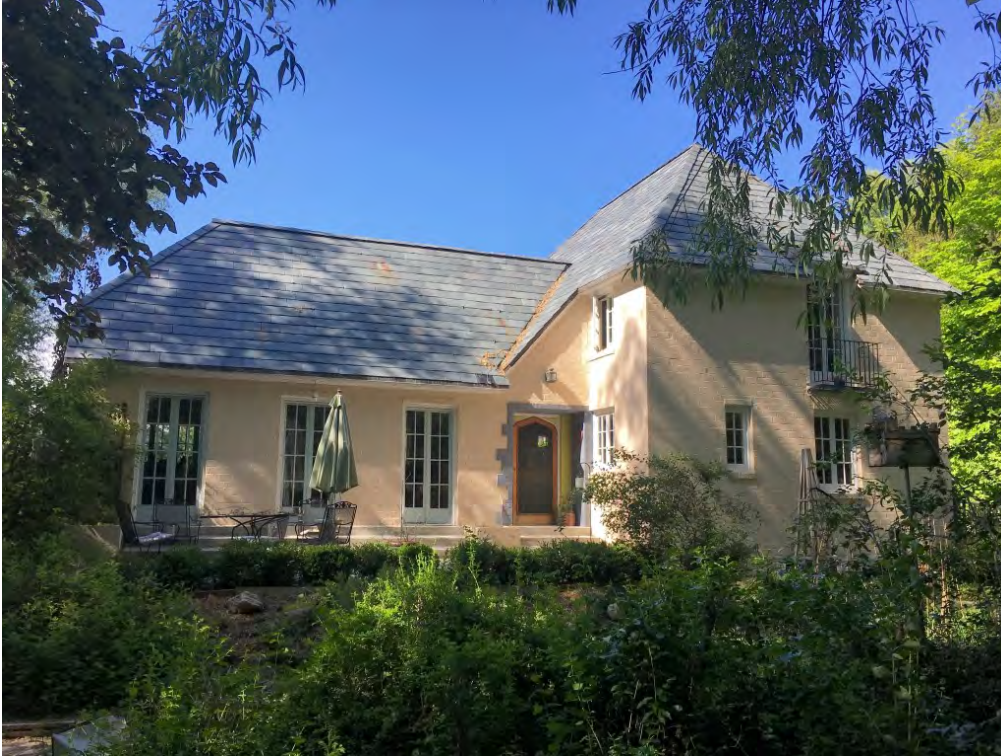
Photograph 1 of 19. West and south elevations. Camera facing northeast.
