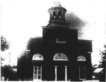
German Reformed Church with 1832 façade with ca.1870 belfry. In 1890 the parapet, ca.1870 belfry, and central entrance were removed and replaced with the tower entrance seen on the building today (2008). (Copy of historic photo at Maryland Historical Trust, original at the Christ Reformed UCC Church).
