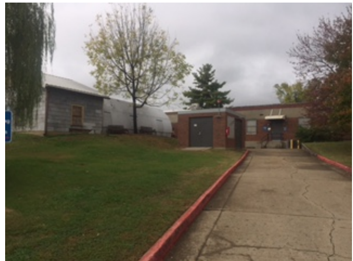
Buildings near to the Paint Shop
