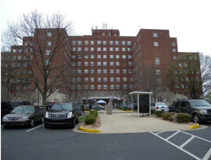
Main Hospital, main façade, northeast side
