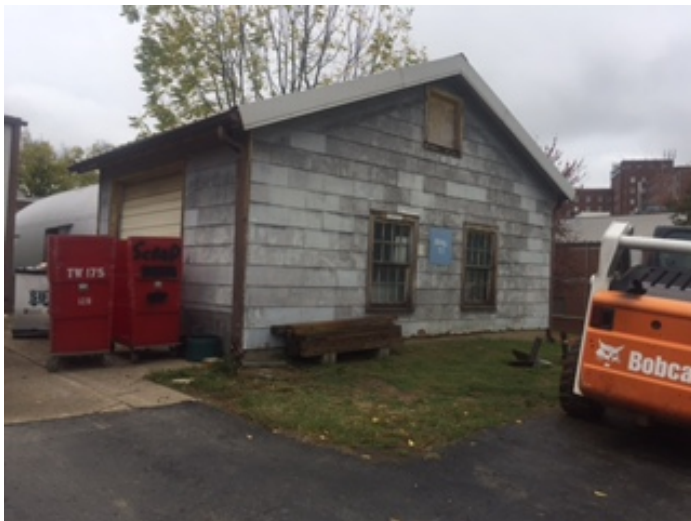
Building T-1, Paint Shop
