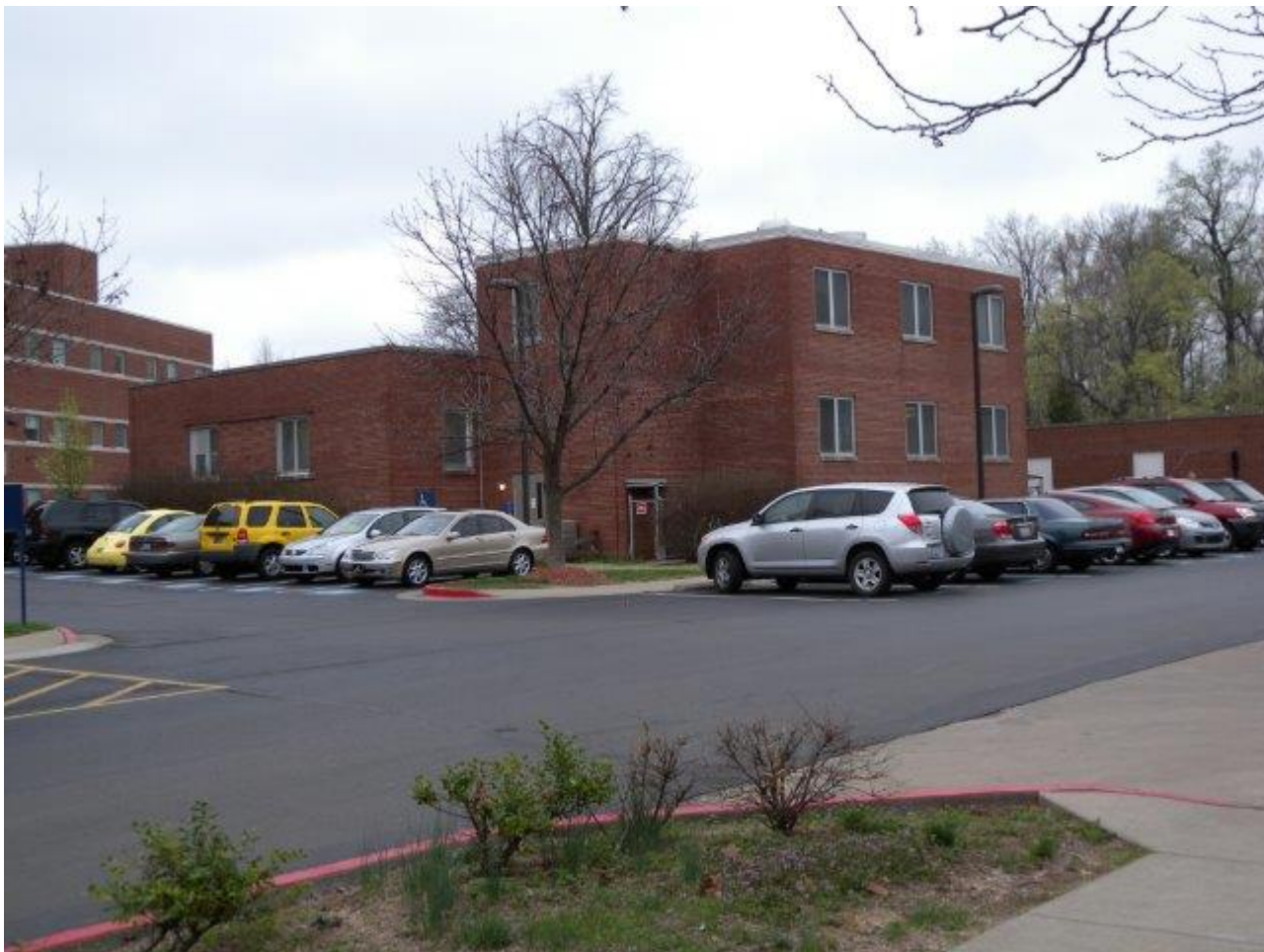
Building 19, former Radioisotope Lab, now Research Facility
