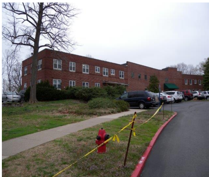
Buildings 3 and 4: Administrative & Engineering
