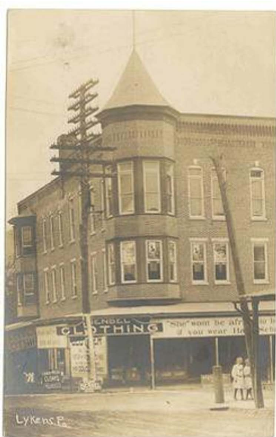
Figure 5.2 Historic Photograph, ca. 1910. Looking north at the Main and Market St facades and turret.
