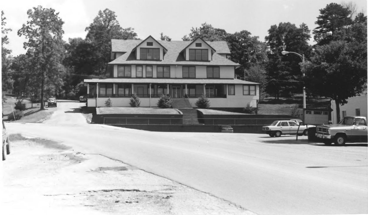
Stearns Commercial Historic District, McCreary Co., KY, Photo 1
