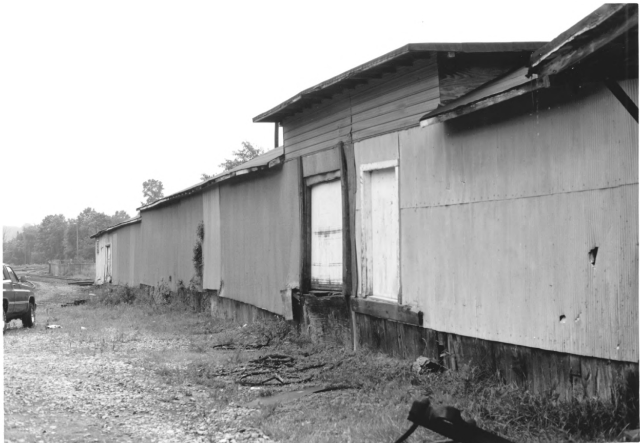
Stearns Administrative and Commercial District. McCreary Co., KY
