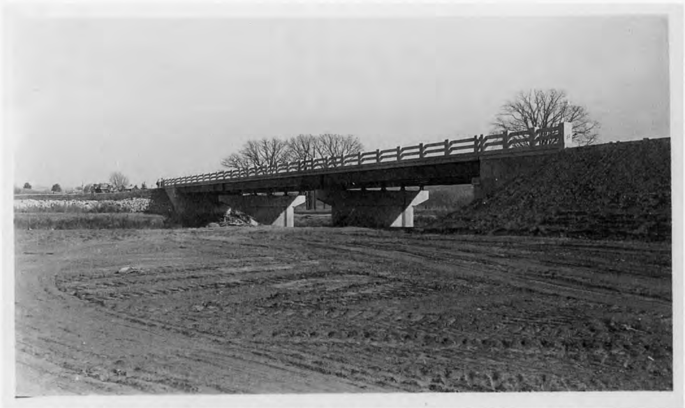
1949 Image of Bridge No. 6679. Photograph courtesy of the Minnesota Historical Society.
