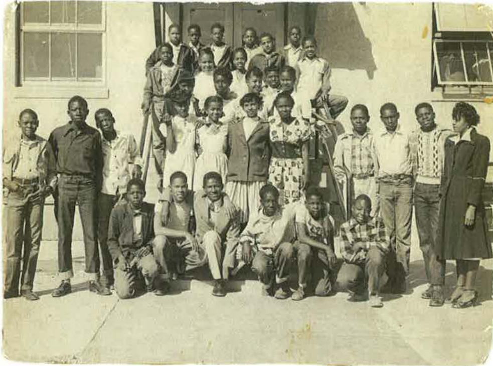
Figure 43. Image of a homeroom class along the west elevation of the Dunbar School ca. 1940s. Image courtesy of the Dunbar Coalition Archives.
