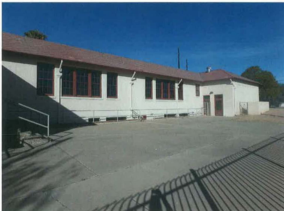
Figure 20. Overview of south elevation of the 1918 building, view facing northeast (AZ_PimaCounty_DunbarSchool_0012).
