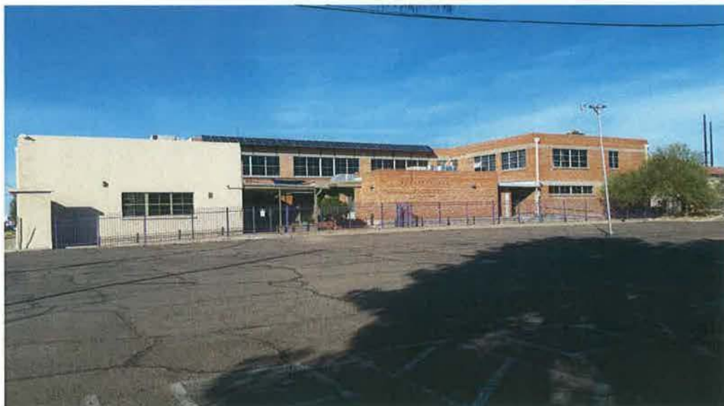
Figure 43. Overview of the south elevation of the 1950 junior high school building, view facing north-northeast (AZ_PimaCounty_DunbarSchool_0016).
