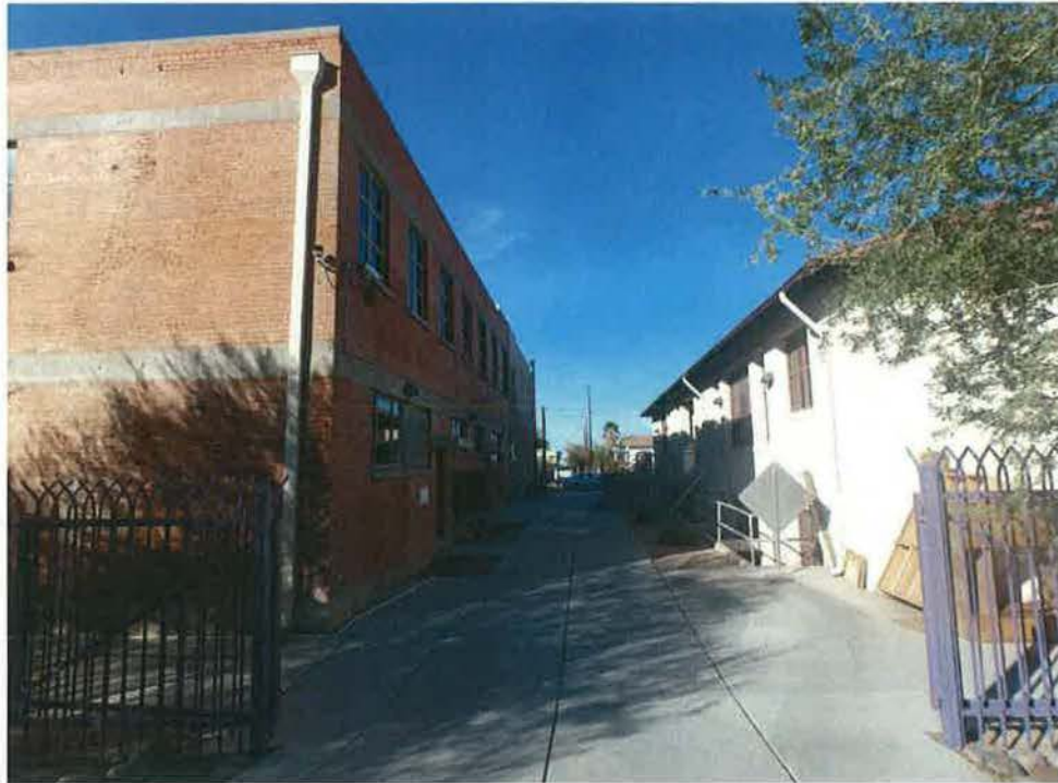
Figure 21. Overview of west elevation of the 1918 building, view facing north (AZ_PimaCounty_DunbarSchool_0013) (note the connection between the buildings was removed during the 2002 rehabilitation project and the west elevation was restored).
