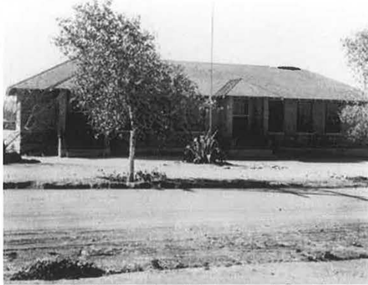
Figure 5. Historical image of the first iteration of the Dunbar School, north elevation (1918). Image courtesy of the Arizona Historical Society, Tucson.
