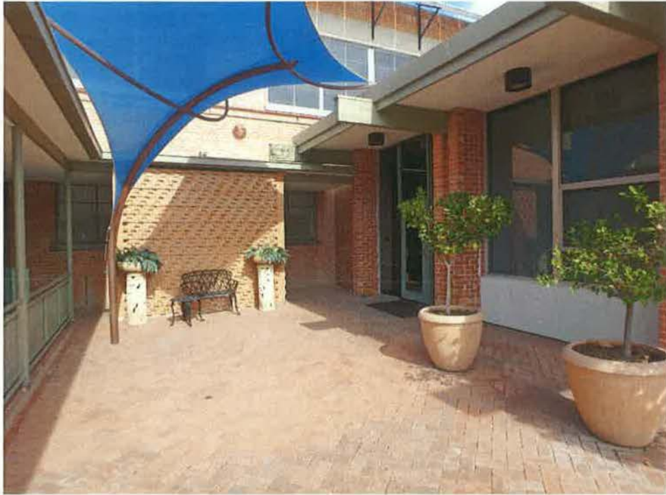
Figure 25. Detail of 1966 library along the south elevation of the 1950 junior high school building, view facing northeast (AZ_PimaCounty_DunbarSchool_0017).
