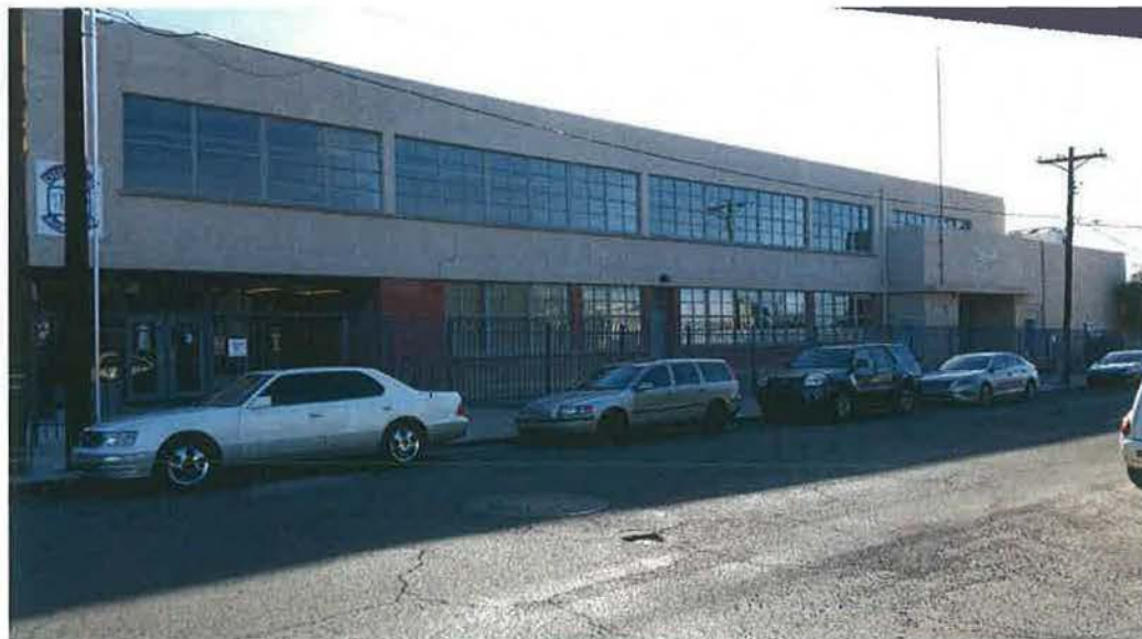
Figure 22. Overview of the north elevation of the 1950 junior high school building, view facing southwest (AZ_PimaCounty_DunbarSchool_0014).
