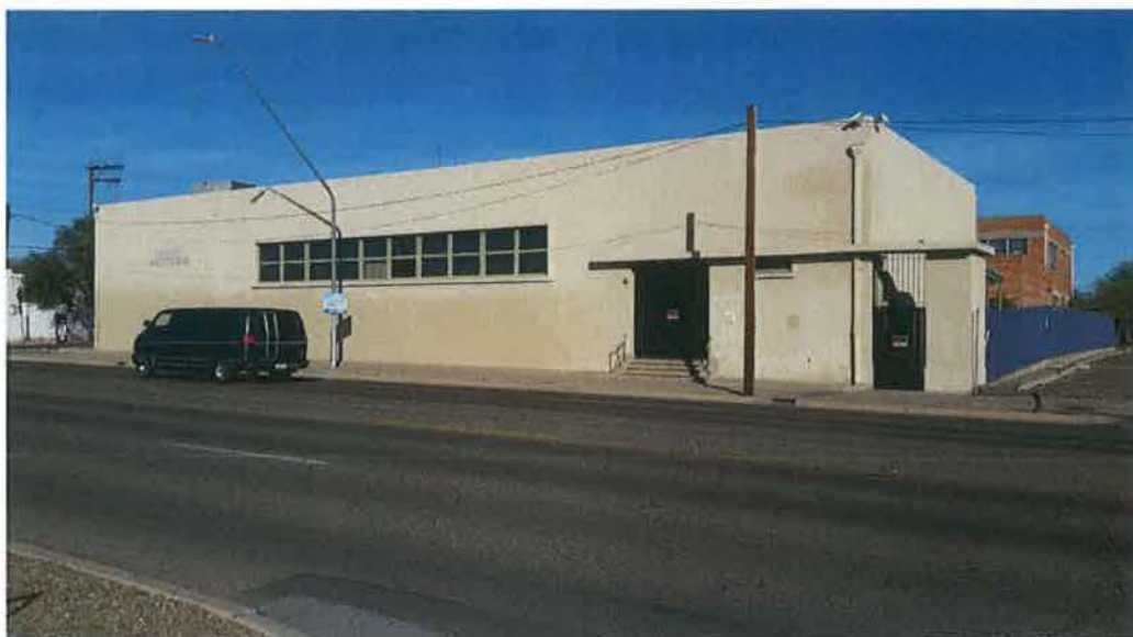
Figure 23. Overview of the west elevation of the 1950 junior high school building, view facing northeast (AZ_PimaCounty_DunbarSchool_0015).
