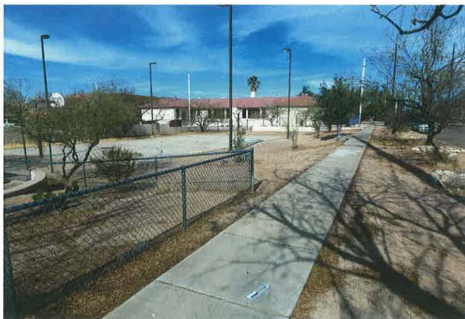
Figure 3. Overview of south elevation and basketball court along 11 th Avenue, facing north-northwest (2018) (AZ_PimaCounty_DunbarSchool_0001).
