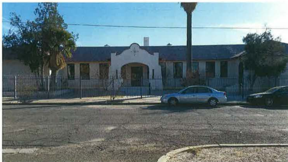
Figure 7. Overview of the north elevation of the 1918 Dunbar School, view facing south (2018) (AZ_PimaCounty_DunbarSchool_0002).
