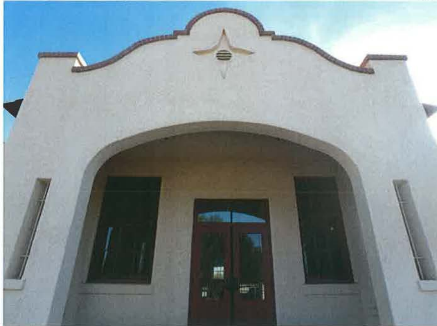
Figure 13. Detail of restored primary entrance of the north elevation, view facing south (2018) (AZ_PimaCounty_DunbarSchool_0008).
