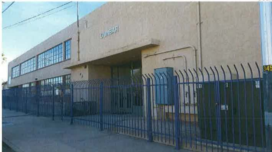
Figure 8. Overview of the north elevation of the 1950 Dunbar/John Spring Junior School portion of the Dunbar School, view facing east-southeast (2018)(AZ_PimaCounty_DunbarSchool_0003).
