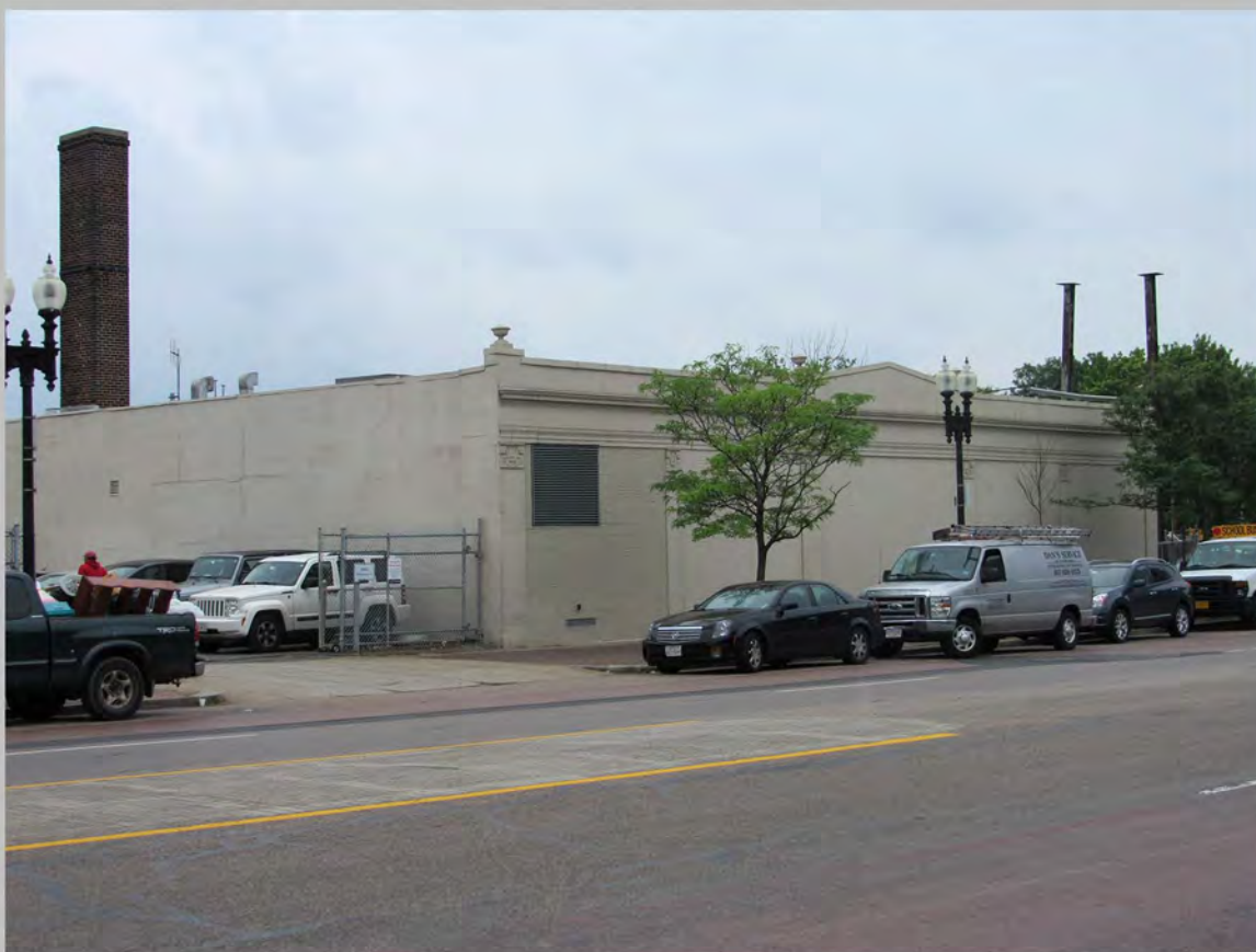
8. View southeast toward 2000 Washington Street
