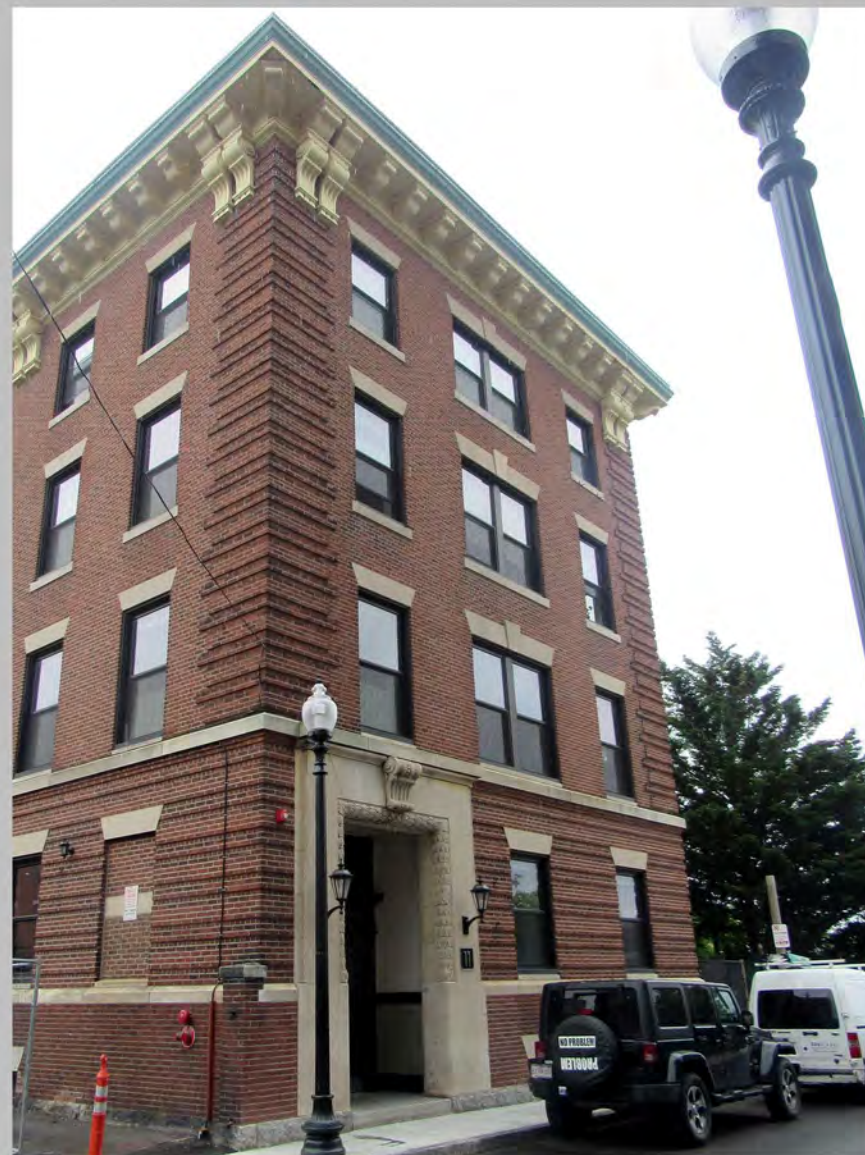
6. View northeast toward 11 Newcomb Street
