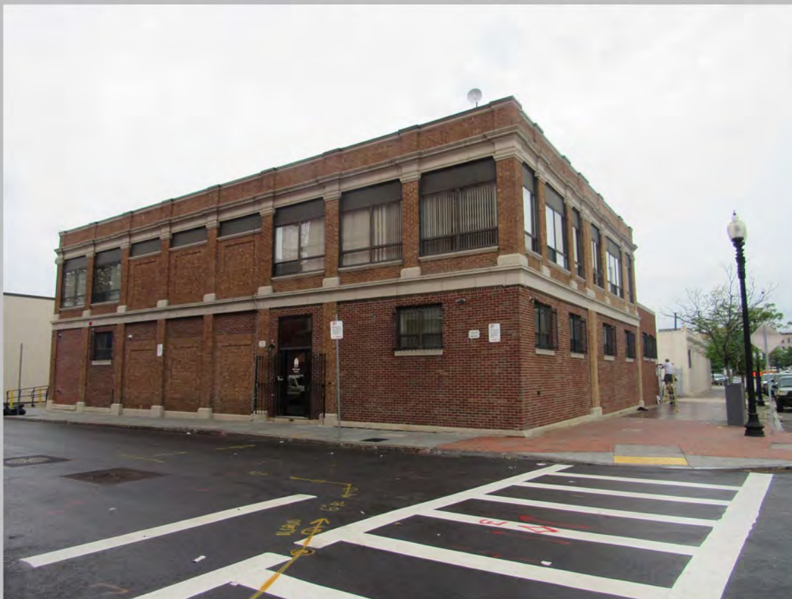
7. View south toward 1960 Washington Street
