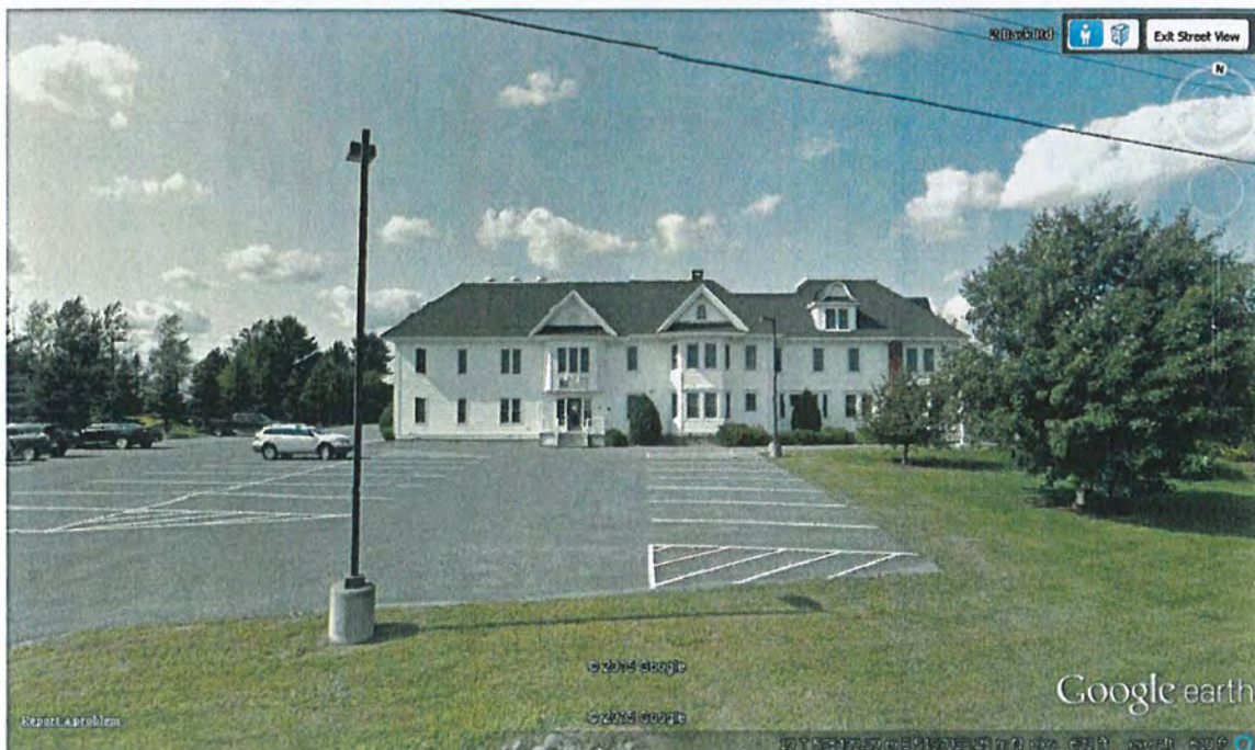
South elevation, McElwain House, July 2014.
