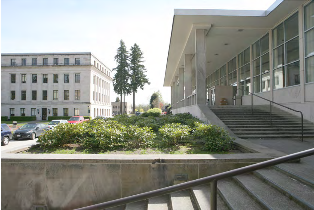
3 of 14. Washington State Library, front north facade looking east with the Cherberg Building in the background.
