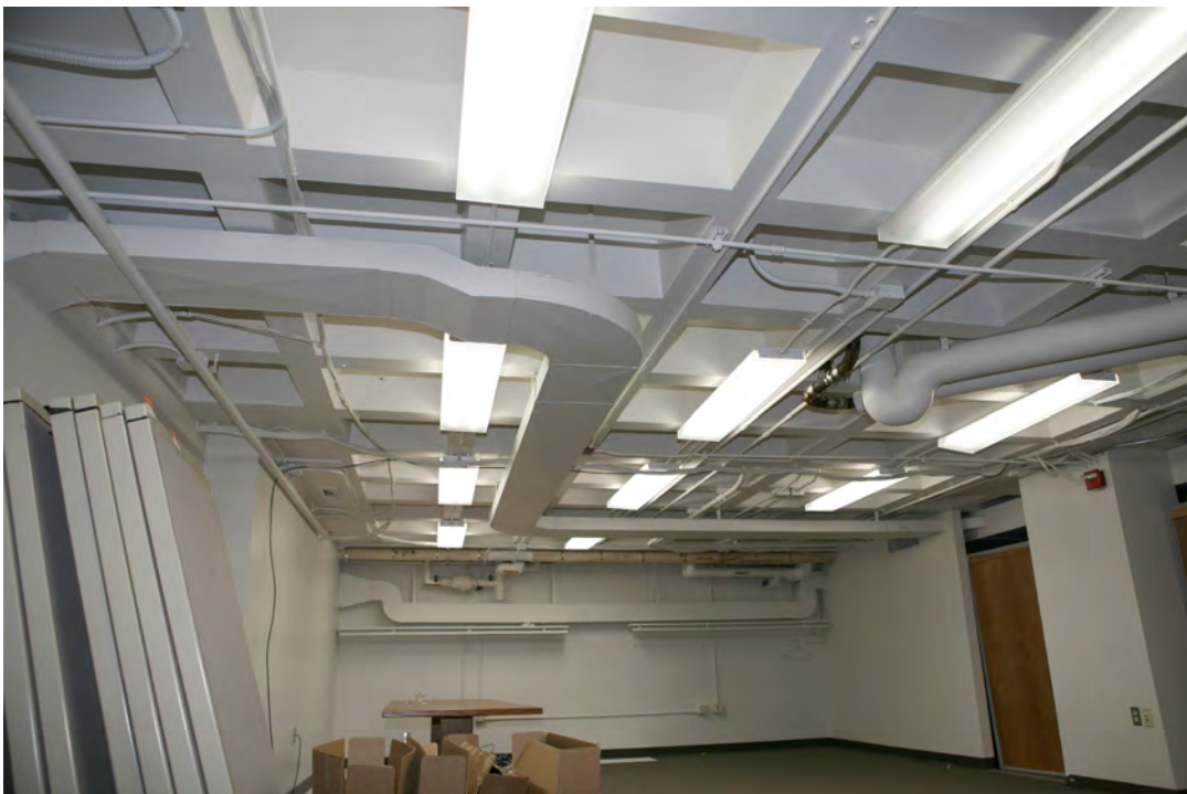
12 of 14. Washington State Library, typical waffle slab configuration in the rear stack volume.
