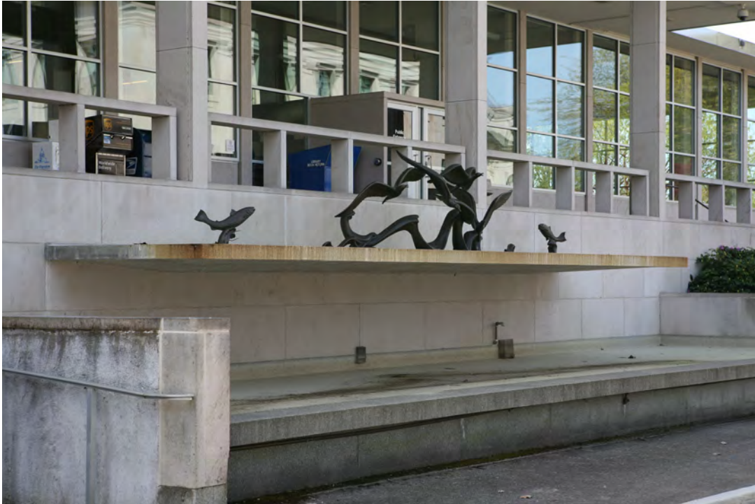
7 of 14. Washington State Library, DuPen fountain on the front north facade.
