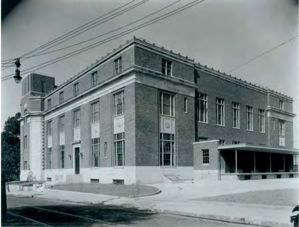
Figure E. Rear (east) and Side (south) elevations, 1931 National Archives, RG 121-BS, Box 79, Folder SS, Print 2
