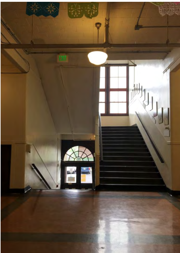
16 of 26: Current Second (Main) Floor – Corridor looking south
