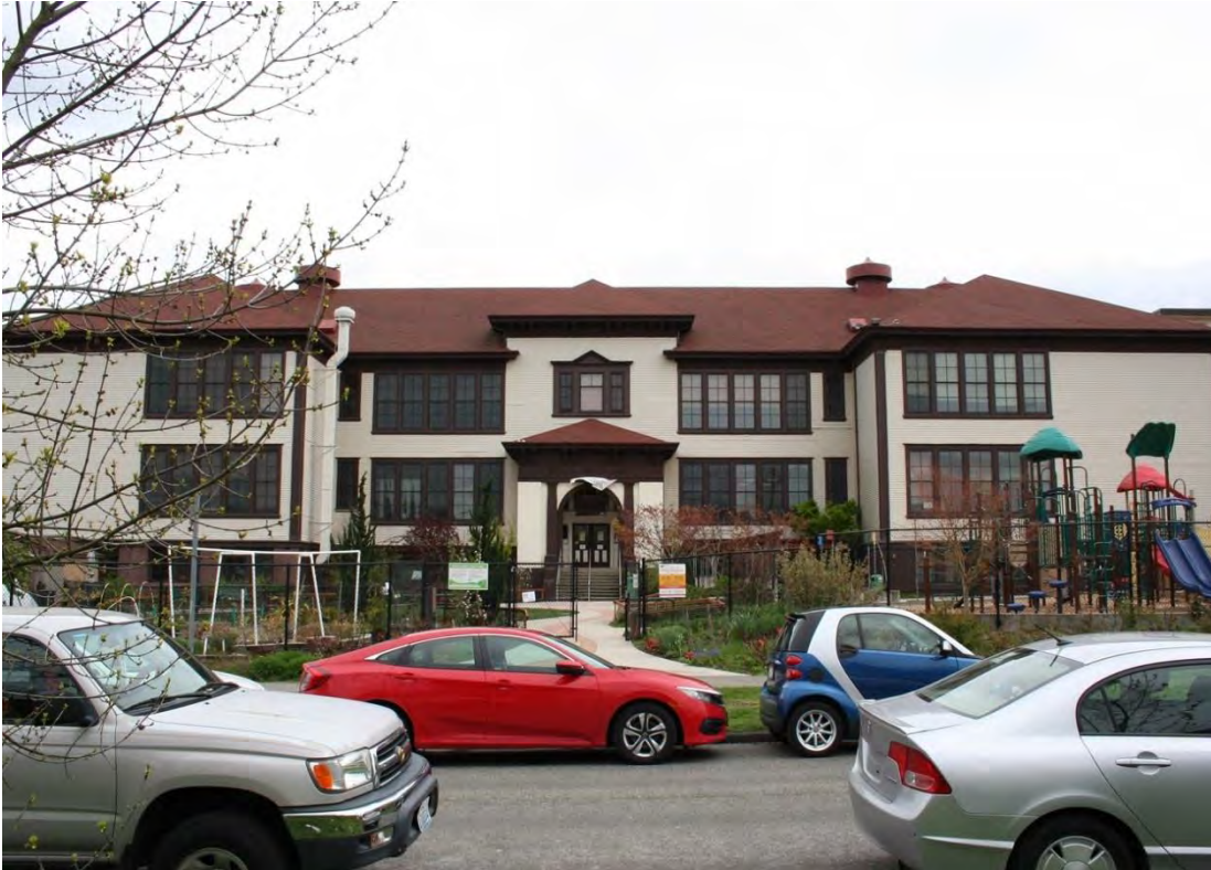
2 of 26: Current west facade
