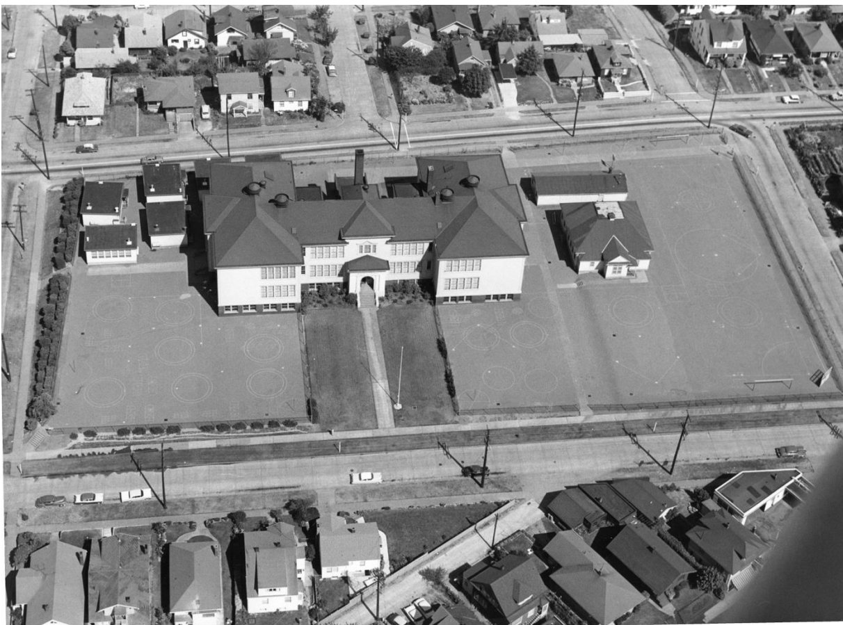
Aerial view of Beacon Hill School from west showing portable classrooms and original 1899 school (at right). c. 1968 Courtesy of Seattle Public Schools, Image 205-14
