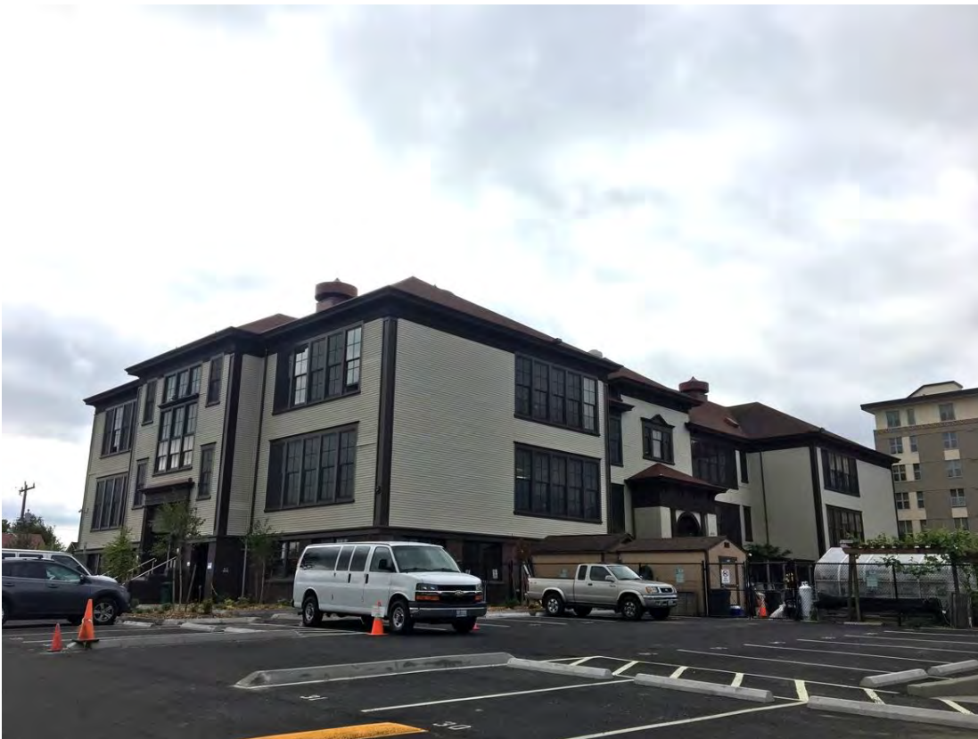
3 of 26: Current northwest corner
