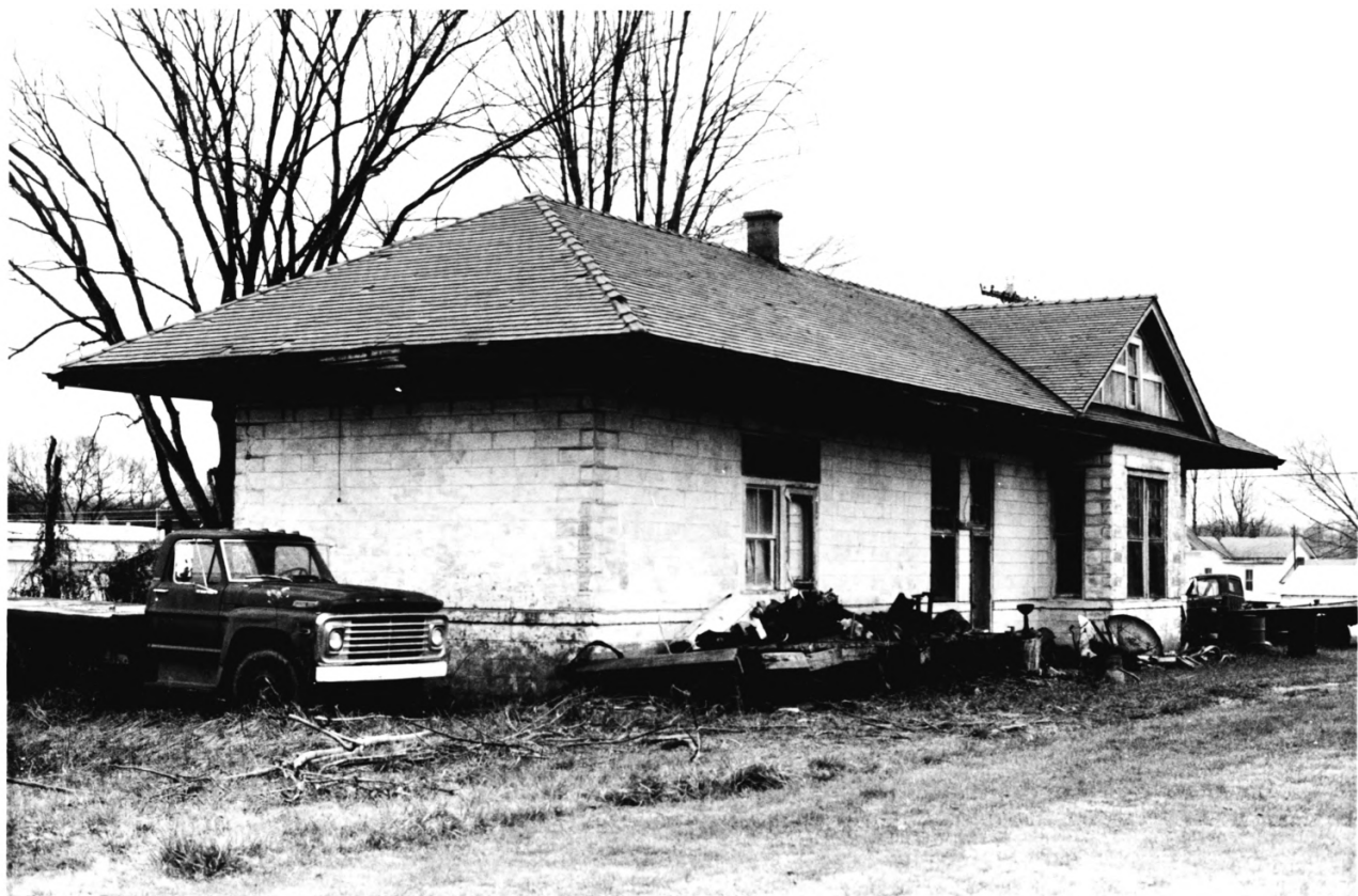
2. Louisville, Henderson and St. Louis Railroad Depot Fordsville, Ohio County, Ky.
