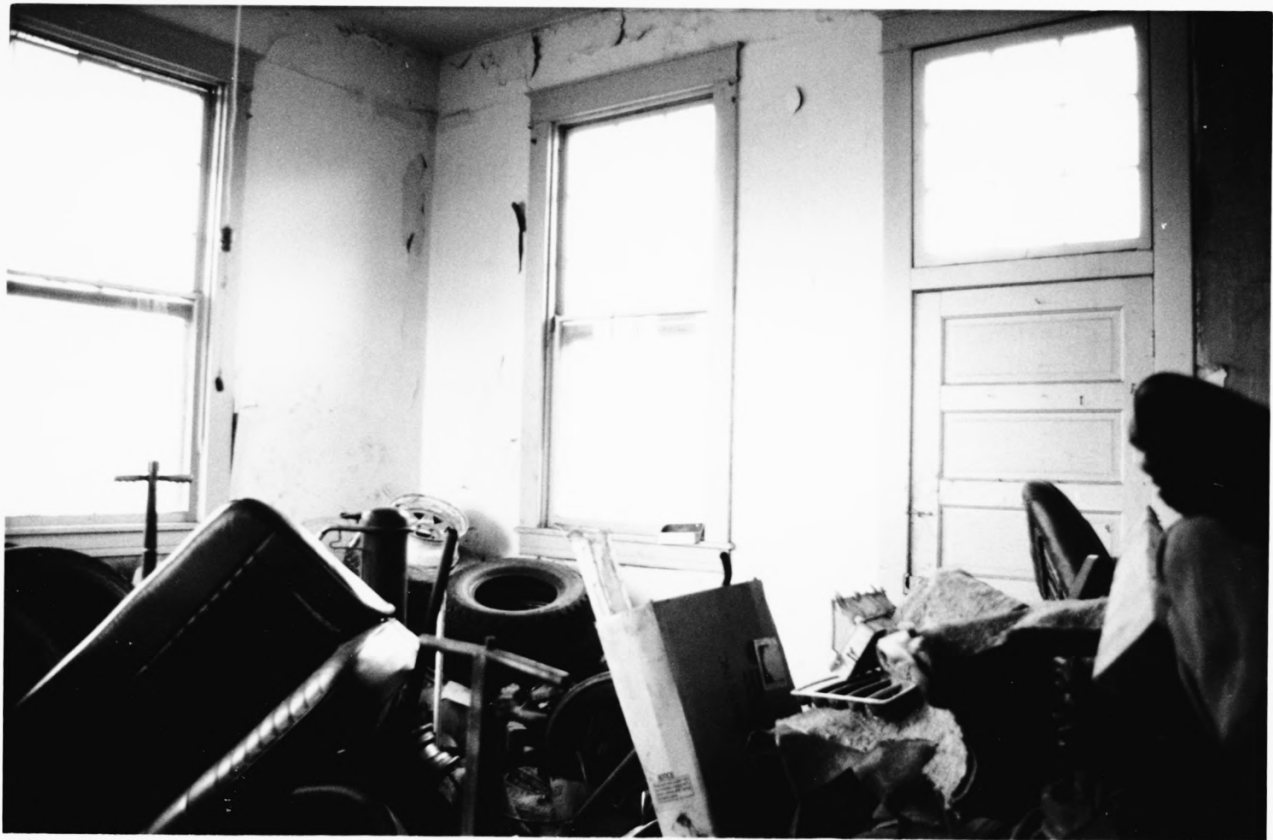
6. Louisville, Henderson, and St. Louis Railroad Depot Fordsville, Ohio County, Ky.
