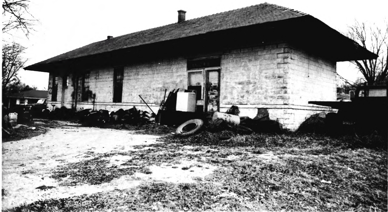
4. Louisville, Henderson, and St. Louis Railroad Depot Fordsville, Ohio County, Ky.
