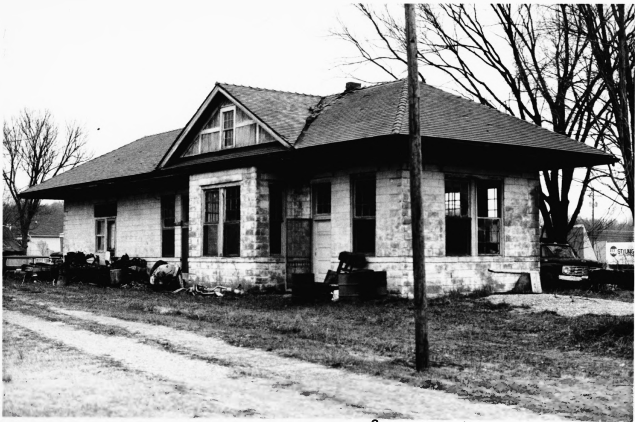
1. Louisville, Henderson, and St. Louis Railroad Depot. Fordsville, Ohio County, Ky.
