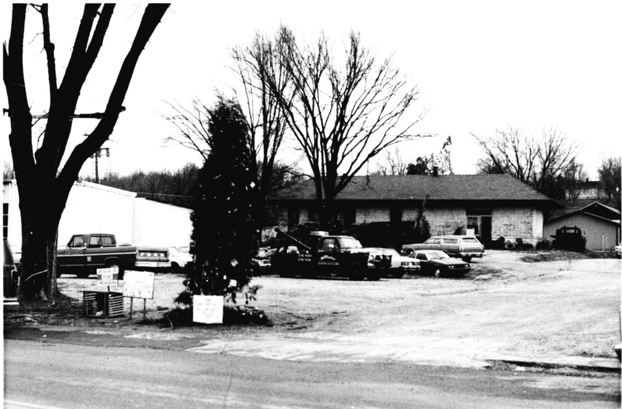
5. Louisville, Henderson, and St. Louis Railroad Depot Fordsville, Ohio County, Ky.
