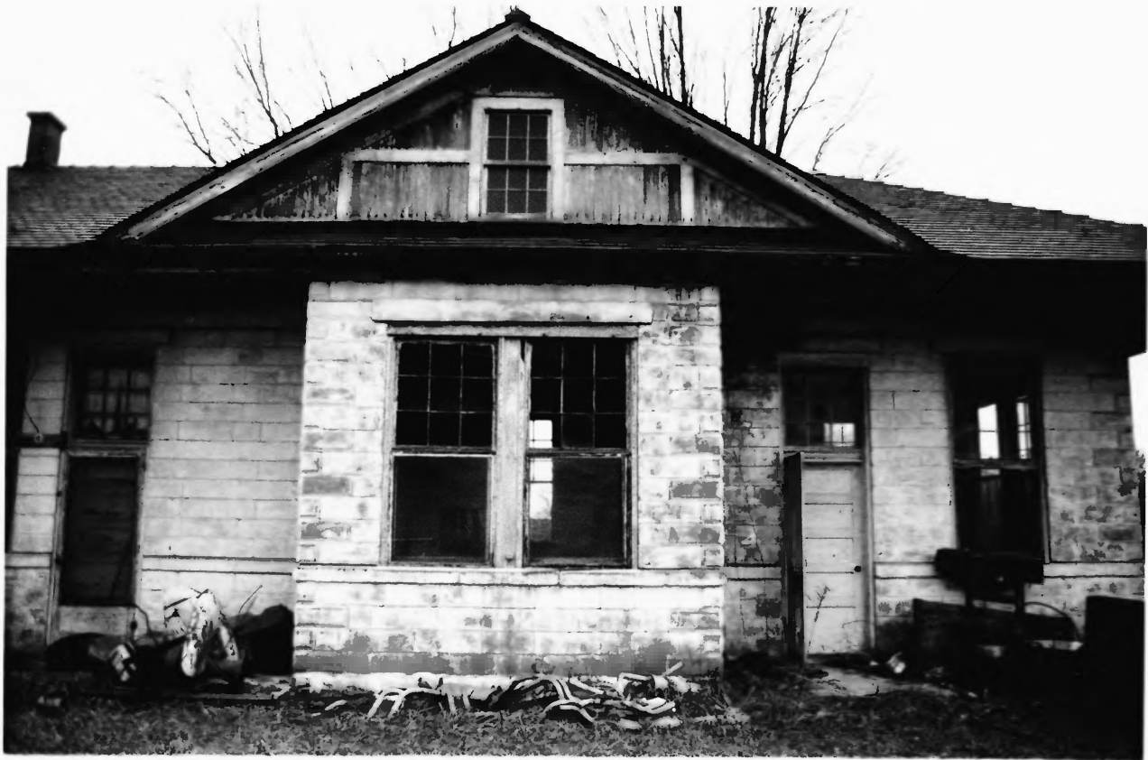
3. Louisville, Henderson, and St. Louis Railroad Depot Fordsville, Ohio County, Ky.
