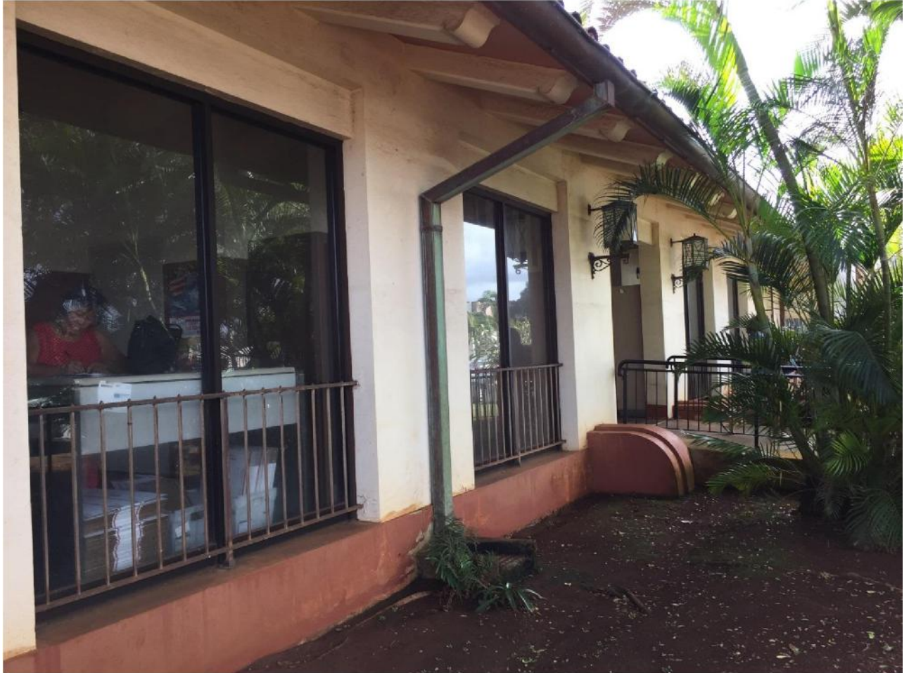
Photograph #2. West elevation (camera facing southeast).
