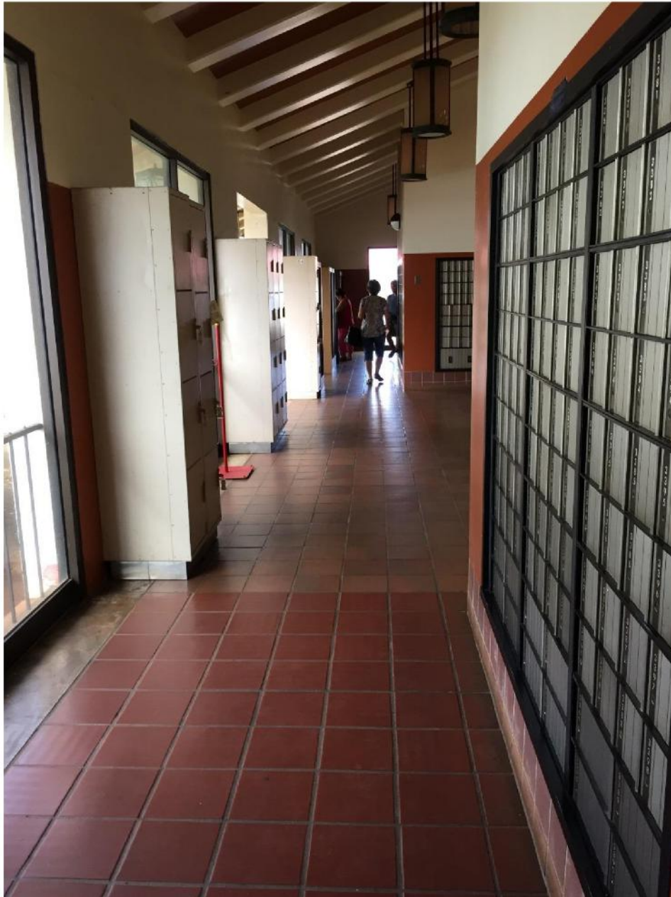
Photograph #8. Interior post office box lobby at west elevation (camera facing southeast).
