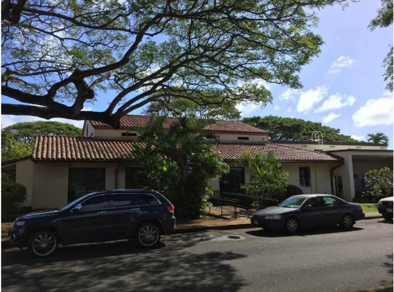
Photograph #3. West elevation (camera facing southeast).
