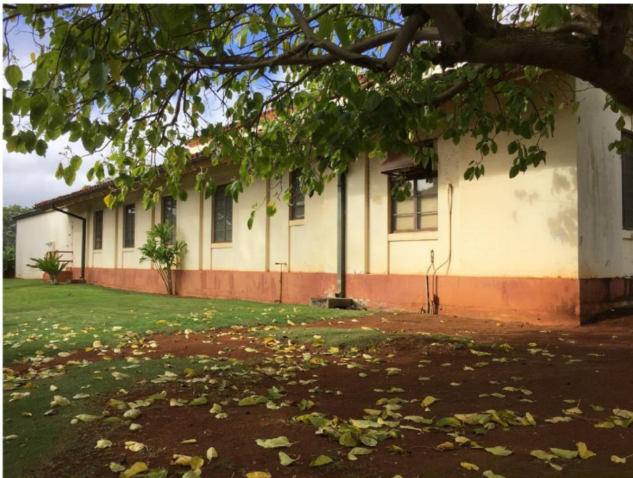
Photograph #4. East elevation (camera facing southwest).
