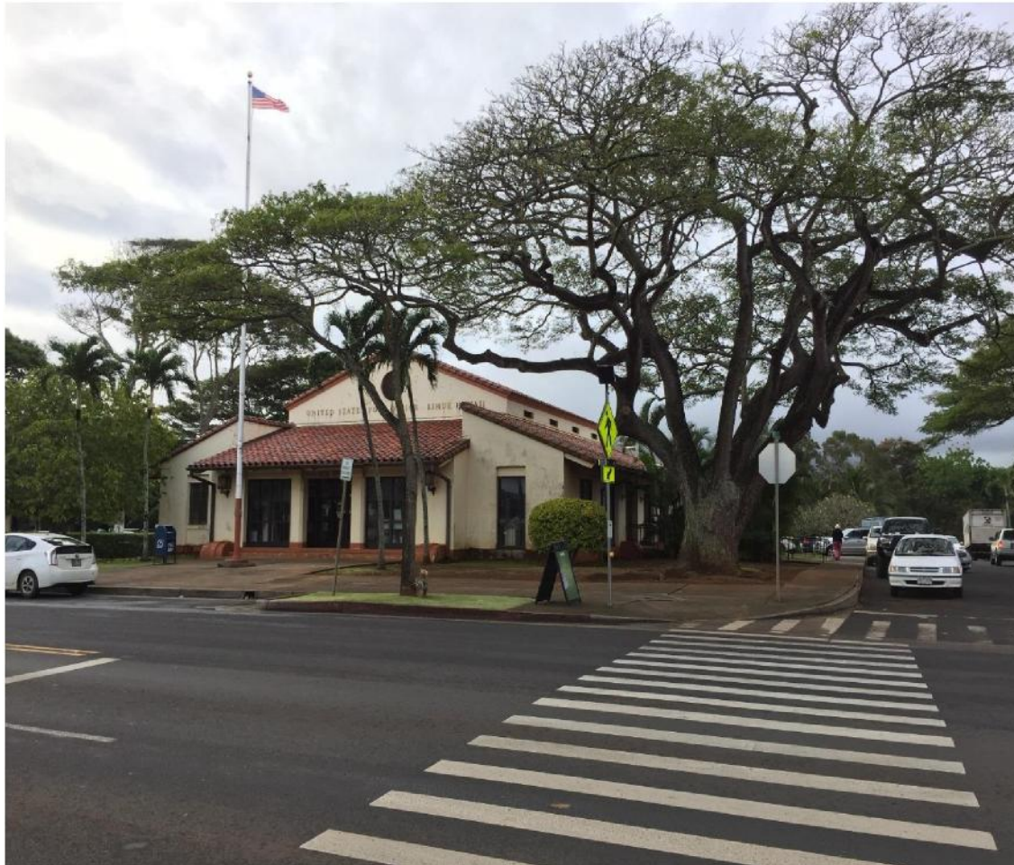
Photograph #1. North (main) and west elevations (camera facing southeast).
