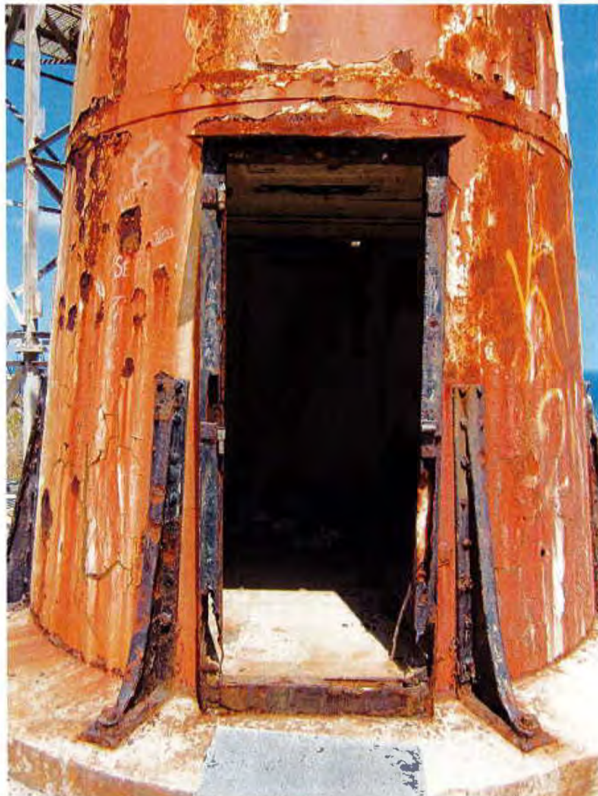
2018 Photo # 3. Entrance exterior, camera facing north, 2018 (VI_St Croix County_Hams Bluff Light_0005
