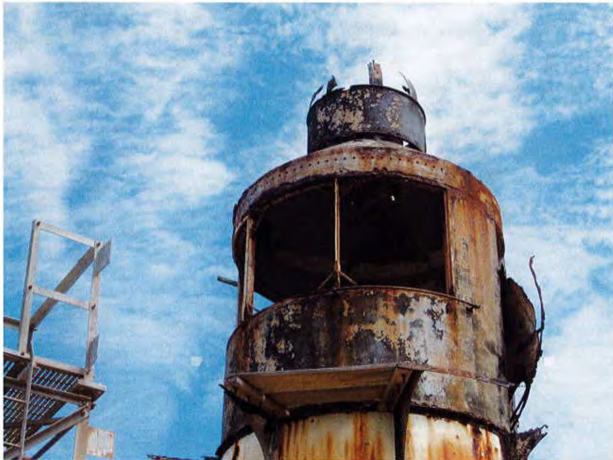
2018 Photo # 2. Lantern exterior, camera facing northeast, 2018 (VI_St Croix County_Hams Bluff Light_0004).
