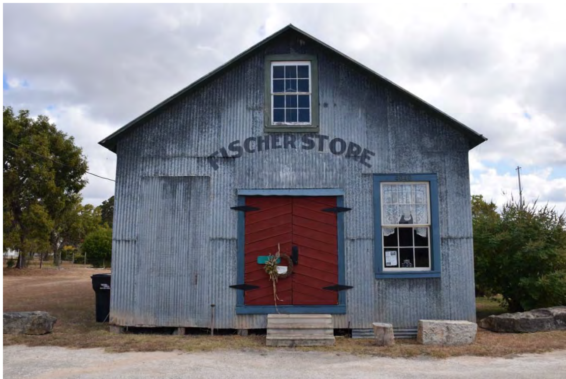
Photo No. 13. PIDN 76783a, 4040 FM 484, front façade of Fischer Store, view facing northeast. October 2015.
