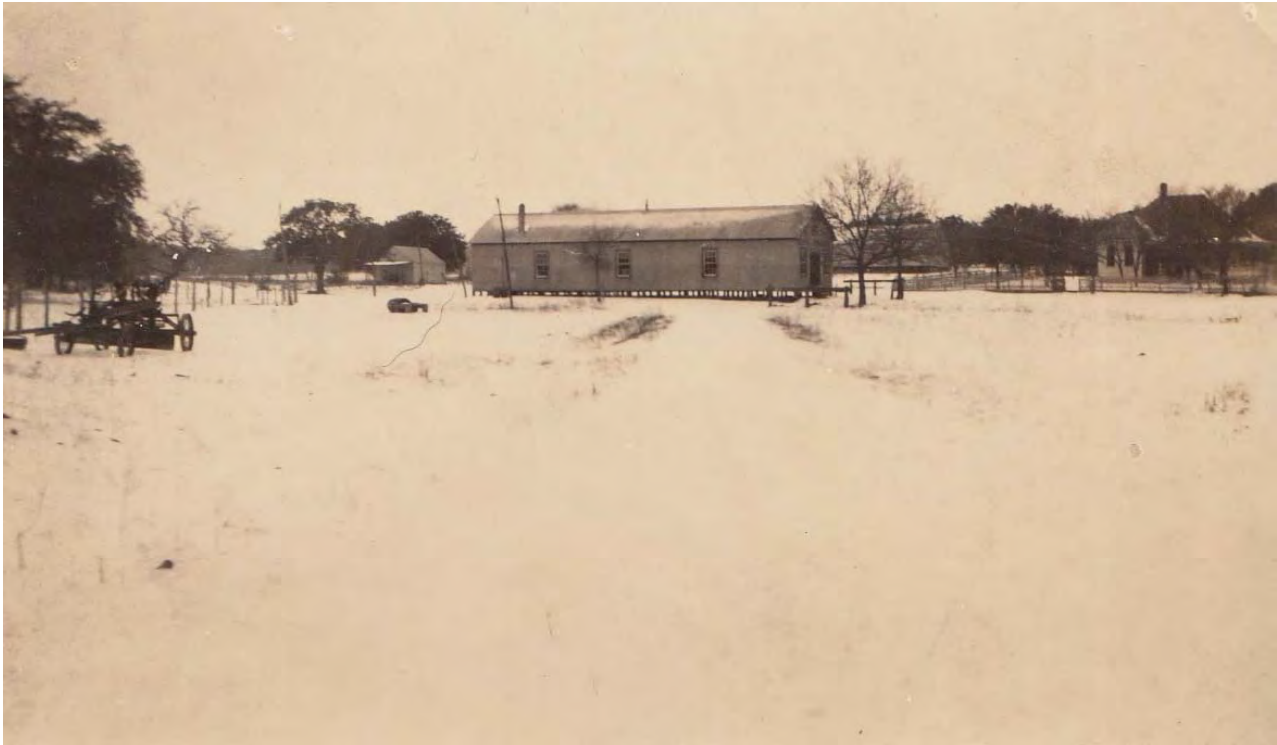
Figure 5. Undated photograph of Fischer Store with the oil house set behind. Source: Arnold B. Fischer Photograph Collection, courtesy of Bryan Weidner.
