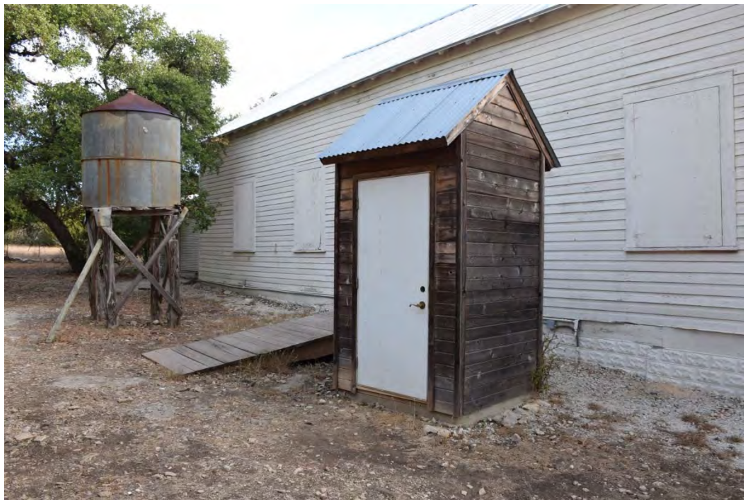
Photo No. 31. PIDN 76773d, 701 Fischer Store Road, oblique view of non-contributing outhouse, view facing northeast. October 2015.
