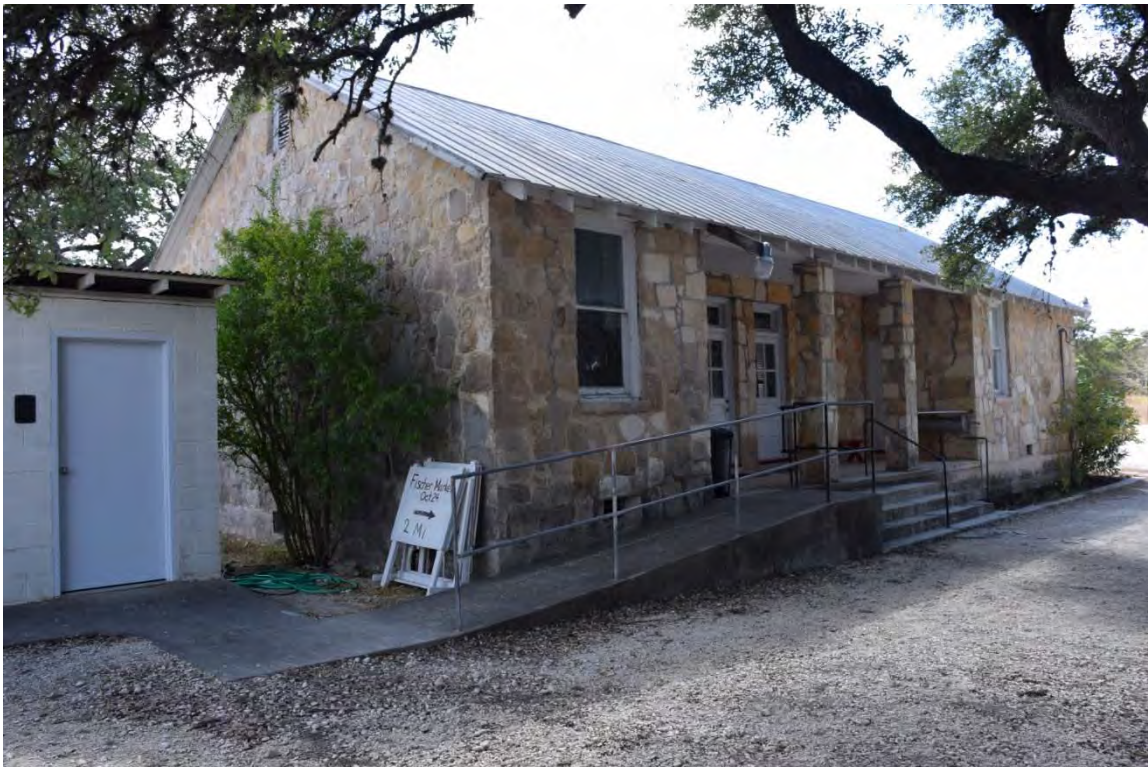
Photo No. 28. PIDN 81591a, 12400 FM 32, oblique view of school, view facing southeast. October 2015.
