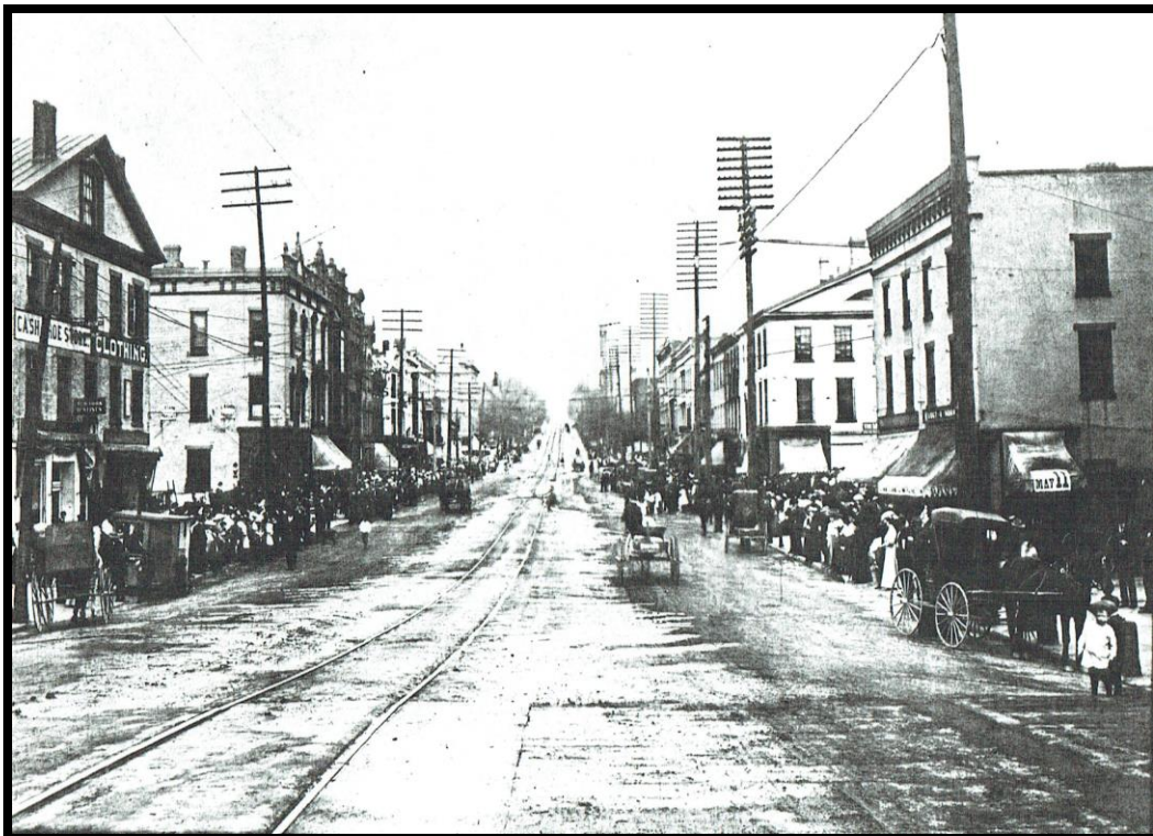
FIGURE 6: Main Street (Lincoln Way), looking east toward Erie Street, c. 1890s
