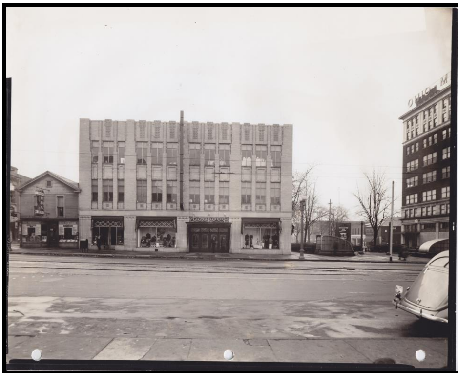
FIGURE 15: South side of Lincoln Way, Stark Department Store, 1938
