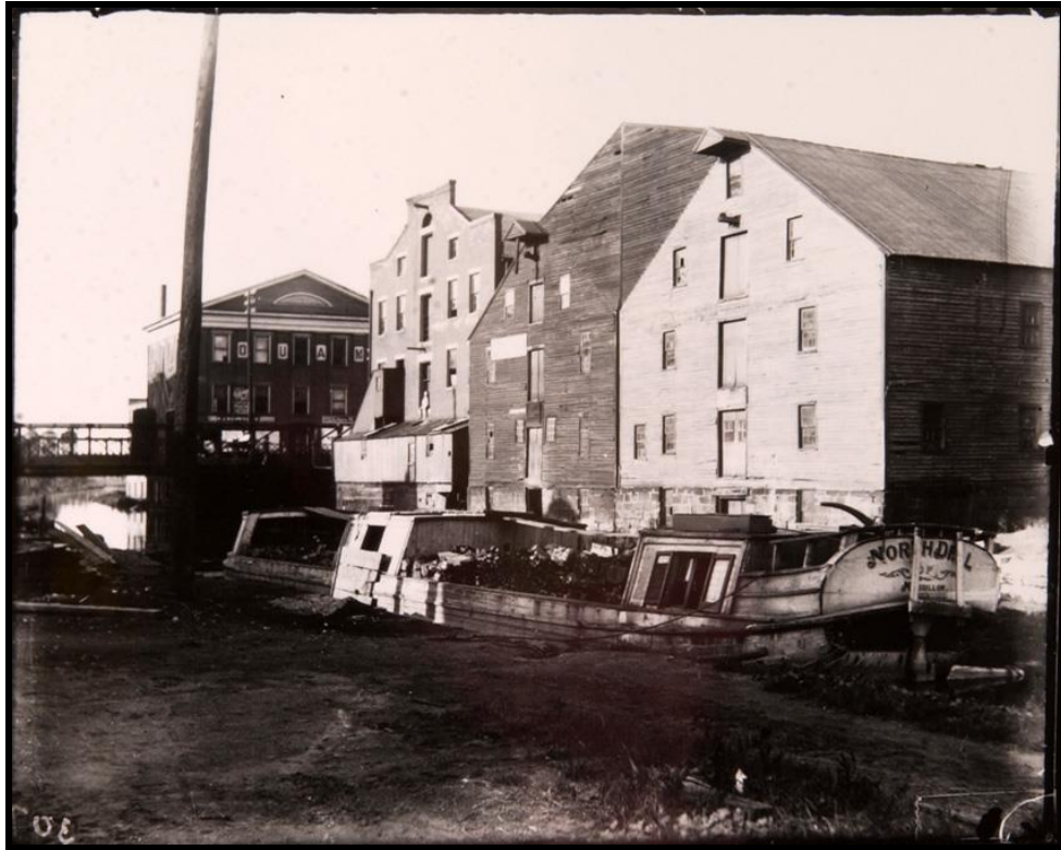
FIGURE 1: Ohio and Erie Canal, looking toward Main Street (Lincoln Way) Bridge
