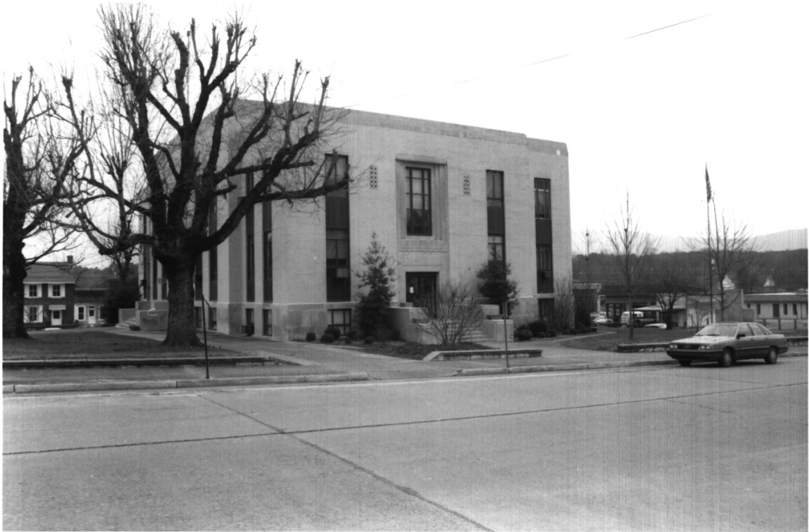
Polk County Courthouse Polk County TN
