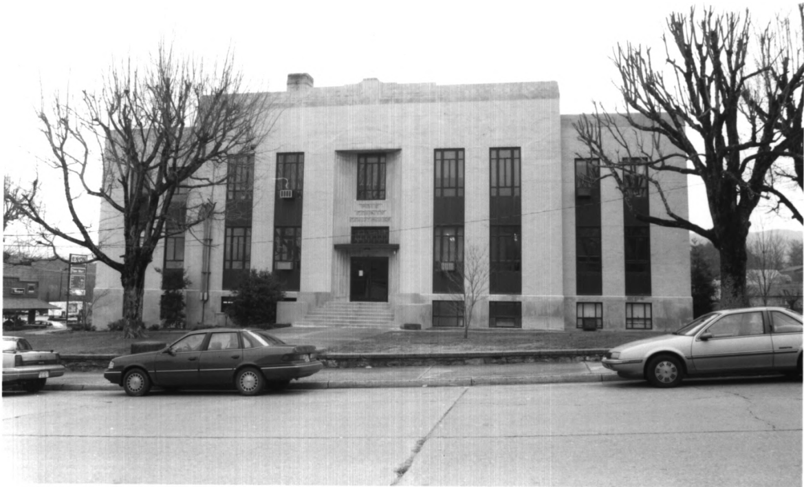
Polk County Courthouse Polk County TN
