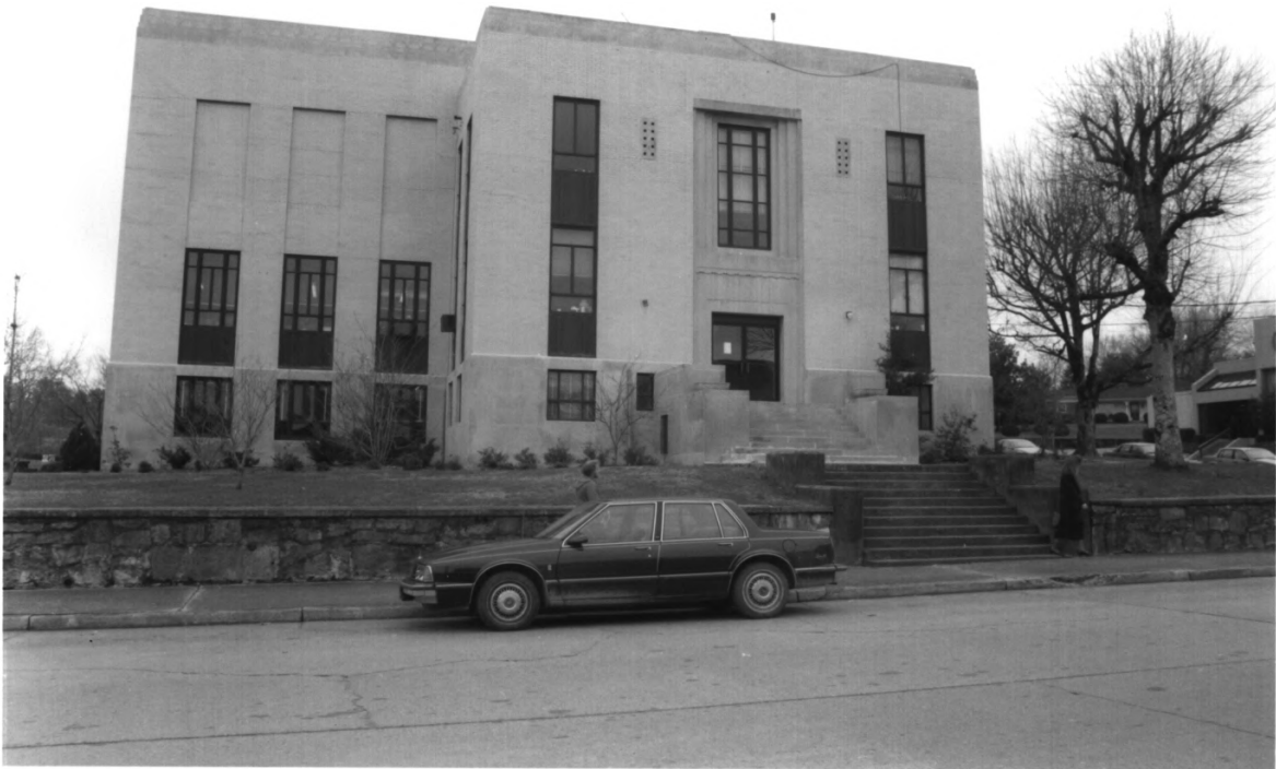
Polk County Courthouse Polk County TN
