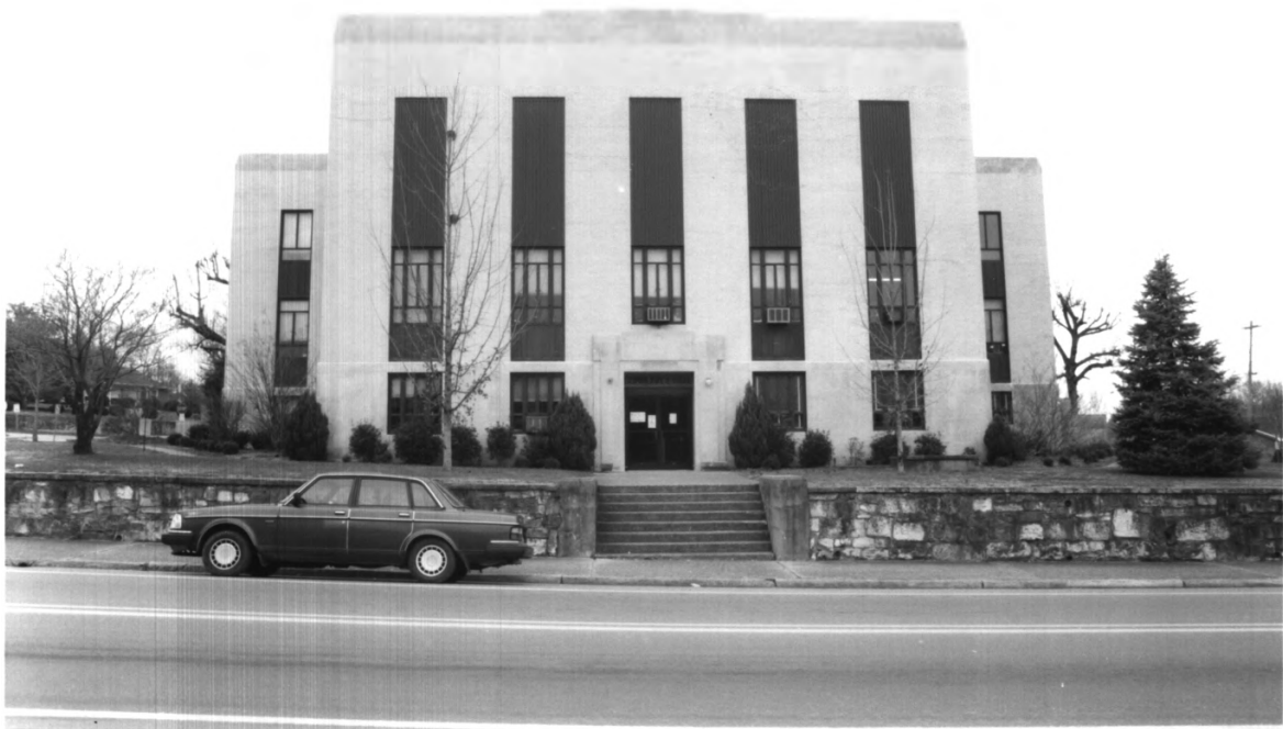
Polk County Courthouse Polk County TN
