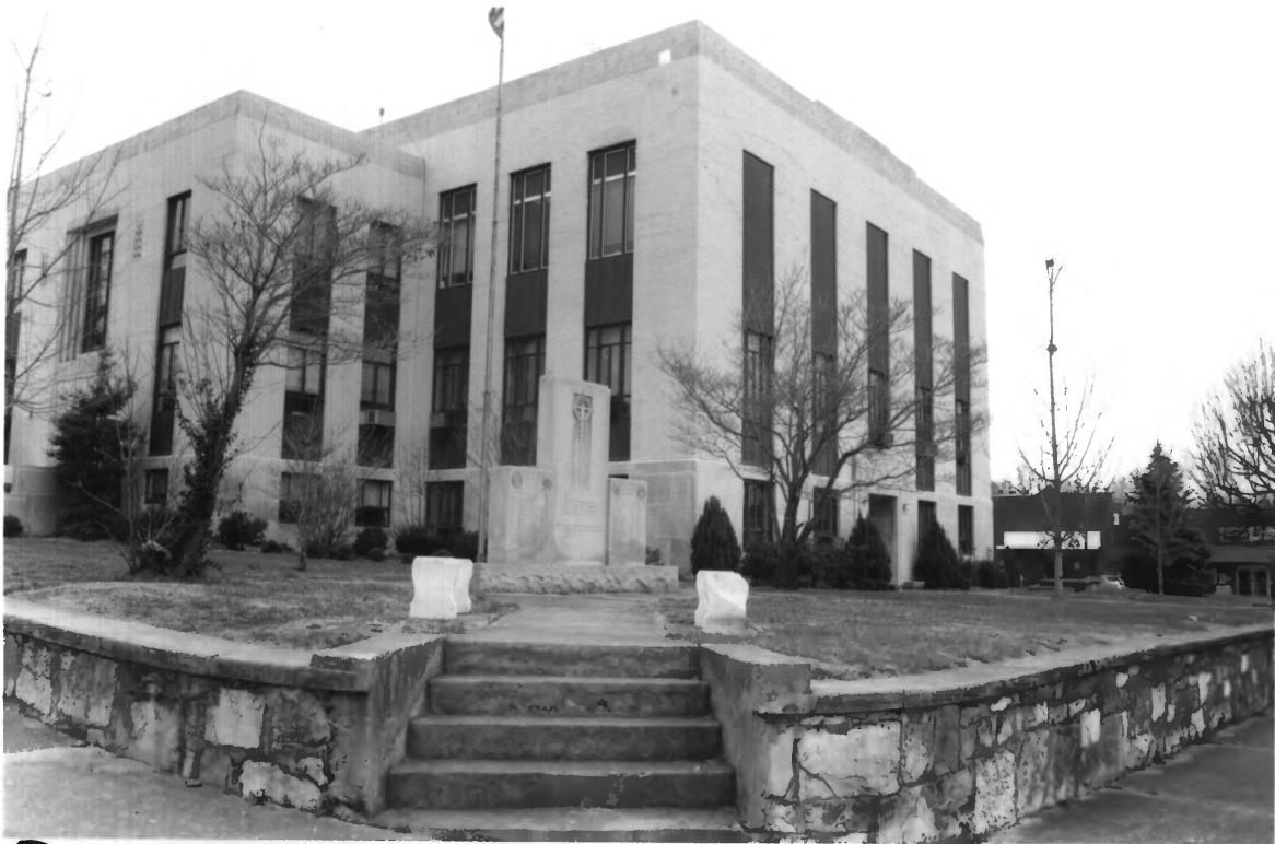
Polk County Courthouse Polk County TN
