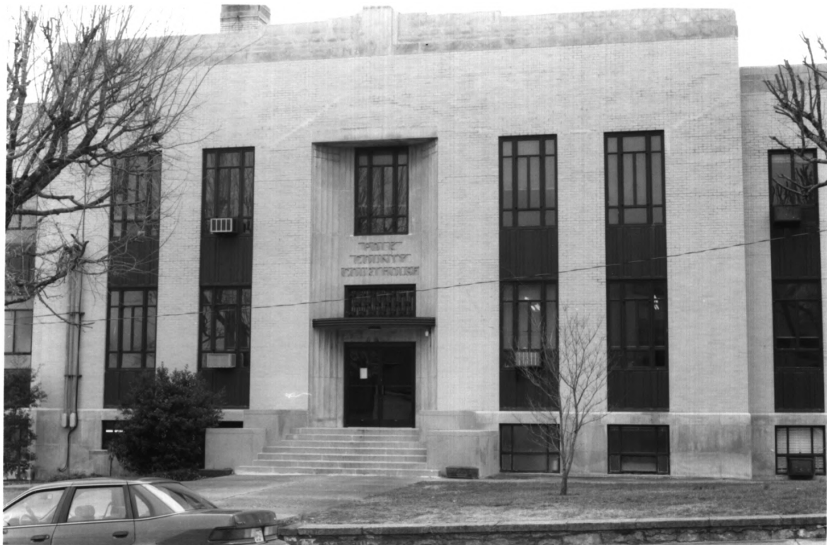
Polk County Courthouse Polk County TN
