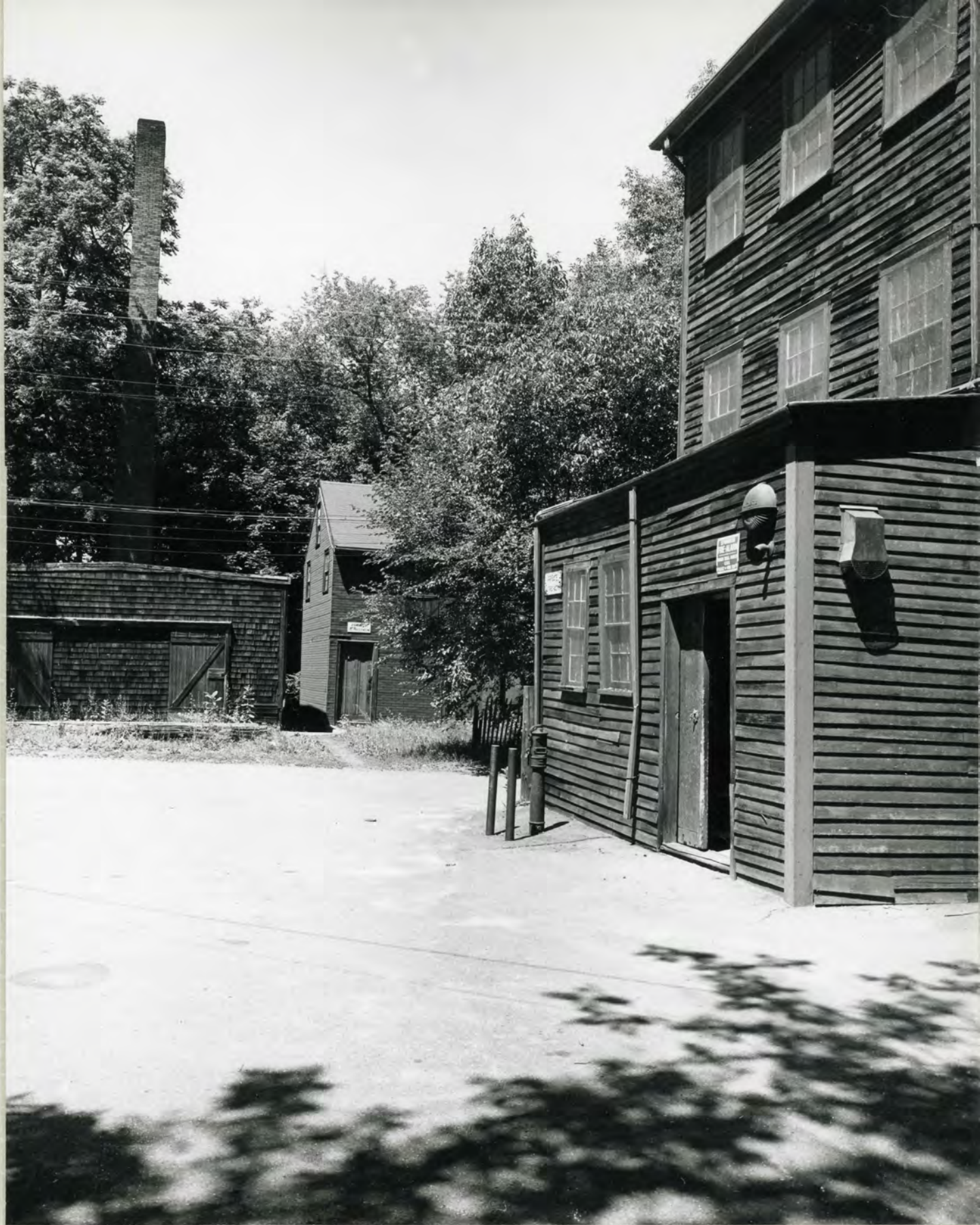
The Old Schwamb Mill, which the Schwamb Mill Preservation Trust is trying to save. The three-story mill on the right contains the unique face plate lathes and other antique machinery. The buildings across Mill Lane are the kiln, left, where lumber was dried and straightened before being made into frames and the wood storage barn, right, whose basement contained the steam engine that powered all the mill's machinery after conversion from water power and before conversion to electricity.
