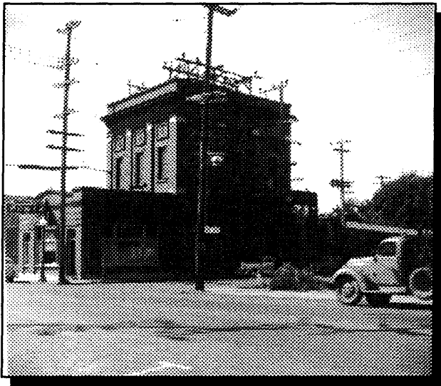
Figure 6. The Oregon Power Company substation ca. 1940. The Mountain States Power Company (a Byllesby affiliate) was housed here by this time.
