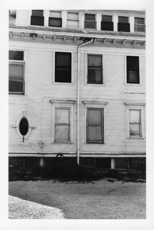
1983 W Detail View showing former location of bay (center 4 windows.) Note splice lines in soffits, patched siding.
