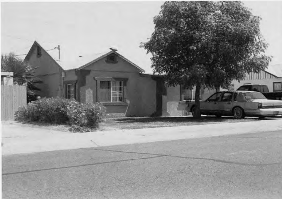
Similarly, the house at 422 West 1 st St. has been sheathed and ornamented in a manner that makes it ineligible for listing as a contributor. View toward northeast.
