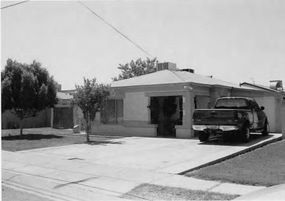
The house at 429 West 1 st St. (WS-86) has been sheathed with stucco and had its original steel casement windows replaced with aluminum sliders. These changes make it a non-contributor to the district. View toward southeast. Photo 7
