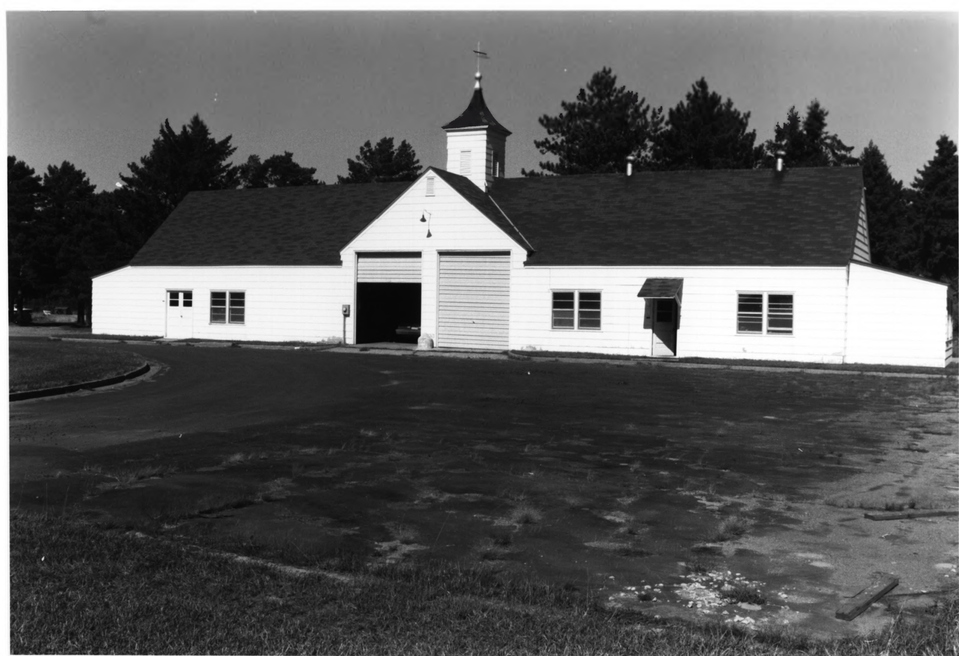
Barn & Storage Building, Carlos Avery Game Farm Ham Lake vicinity, Anoka County, MN 010659-17A
