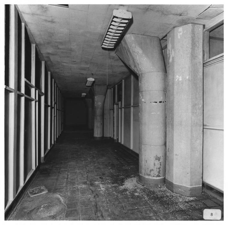
Photographer: James R. Lockhart Negative filed: Georgia Department of Natural Resources Date: February, 1983 Description (8 of 12): First floor area under railroad track showing coal chutes; photographer facing south.
