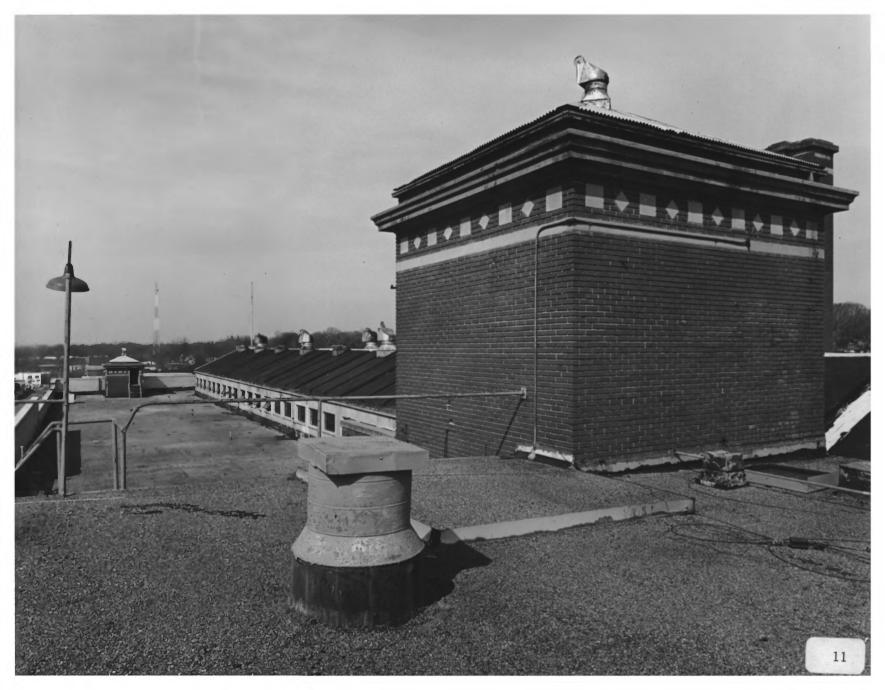
Photographer: James R. Lockhart Negative filed: Georgia Department of Natural Resources Date: February, 1983 Description (11 of 12): Roof showing clerestory area and two elevator towers; photographer facing north.
