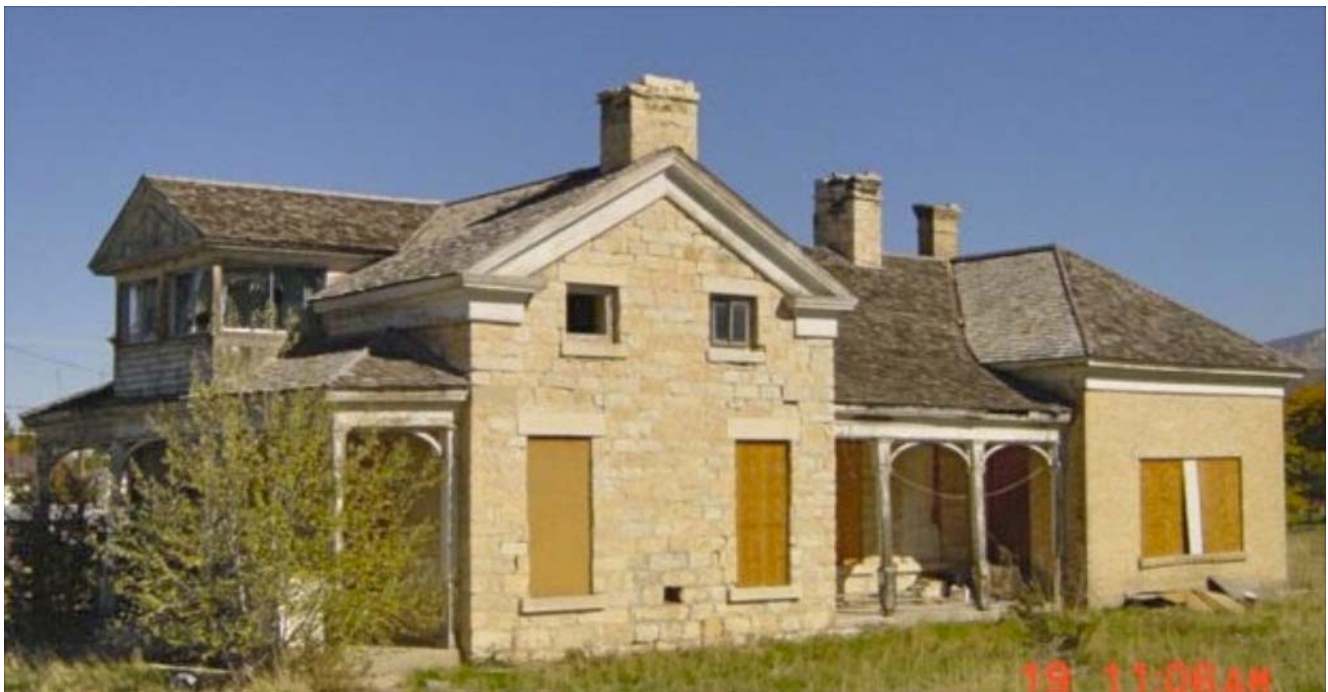
Figure 4 South elevation, detail. Photographed by Shannon Miller, 2002.
