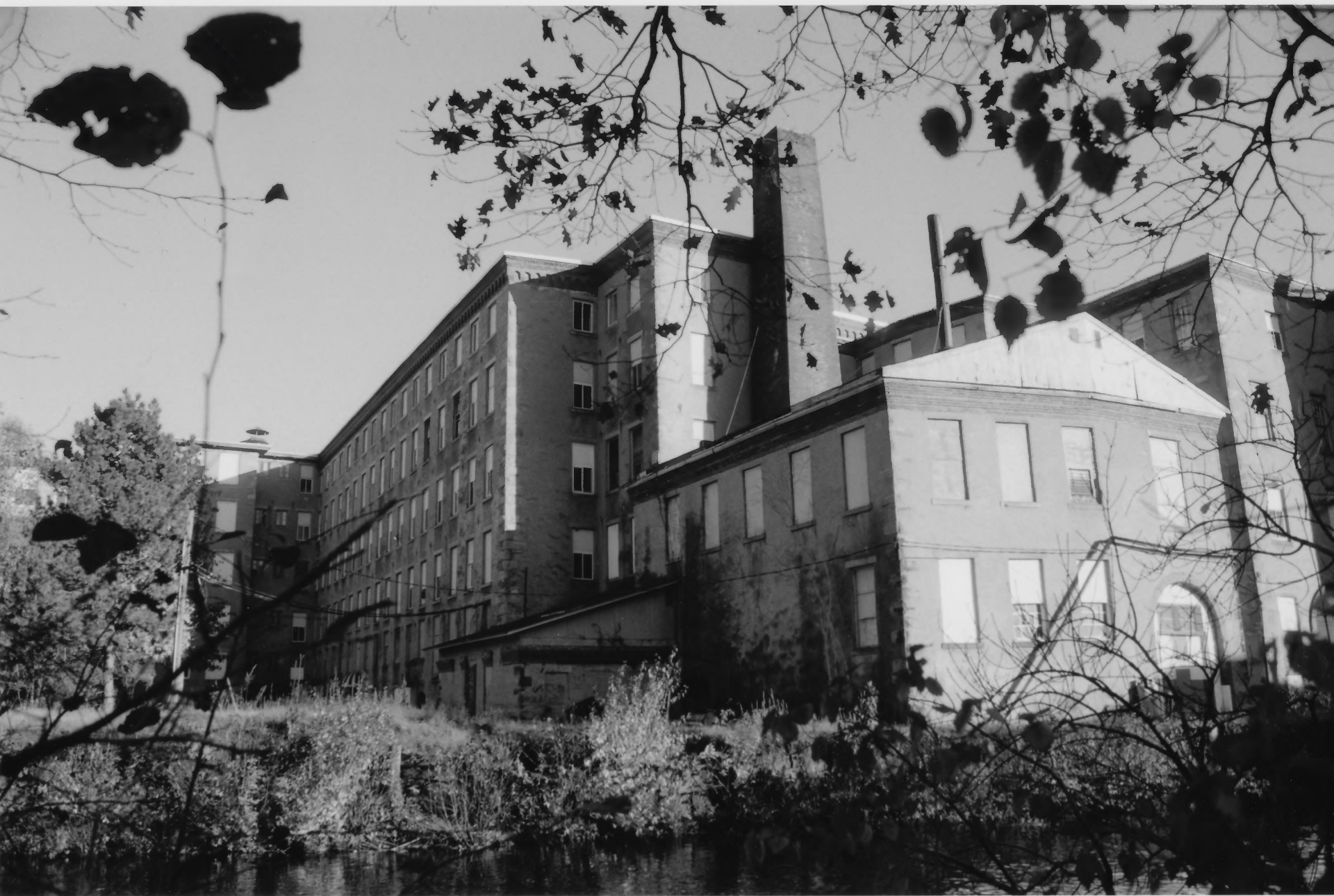
CENTREVILLE MILL WESTWARWICK, KENT COUNTY RHODE ISLAND 3
